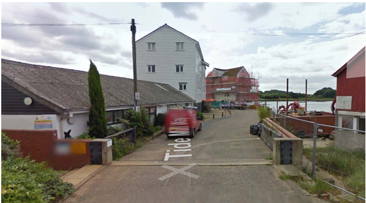
Figure B.1 Example flood gates at Woodbridge in the Deben Estuary
