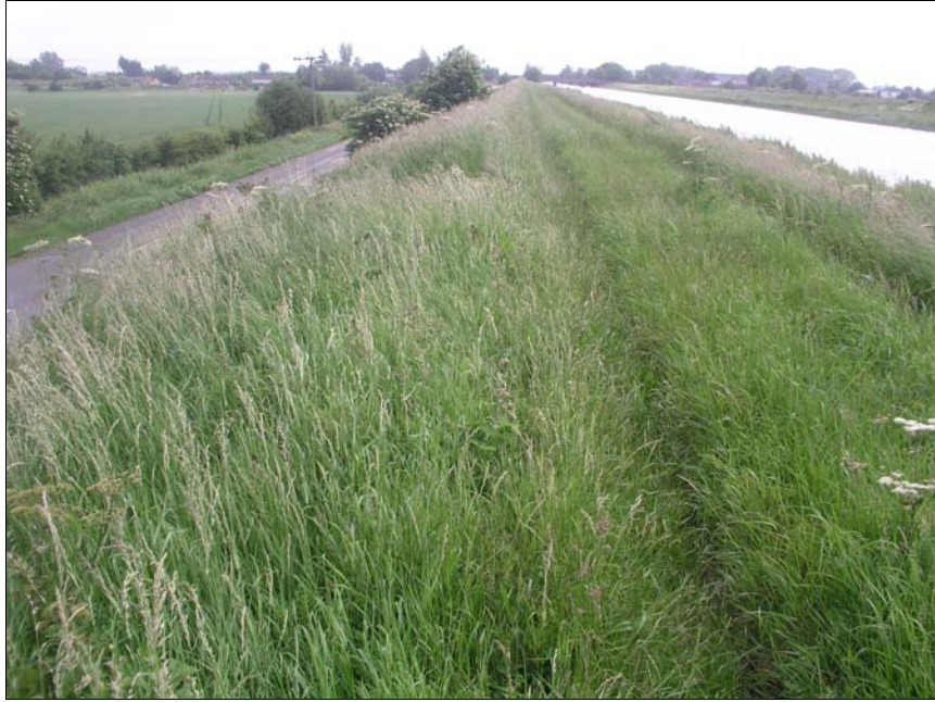
Figure 4.147 Ely Ouse Community G photographed on the landward face of Treatment 11 in June 2007.
