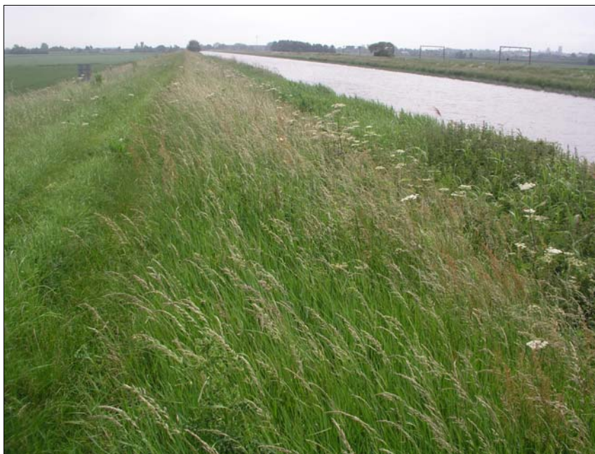
Figure 4.146 Ely Ouse Community F photographed on the river face of Treatment 4 in June 2007.
