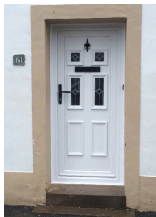
Sue can't keep water out because she floods to 7ft but a flood door gives time to move things
