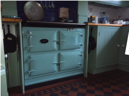
AGA raised on plinth
