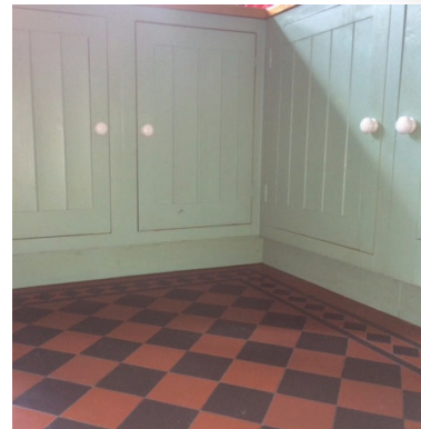
Marine ply units and tiled floors
