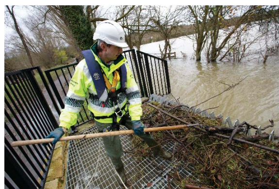
Figure 3. Clearing a trash screen during a flood
