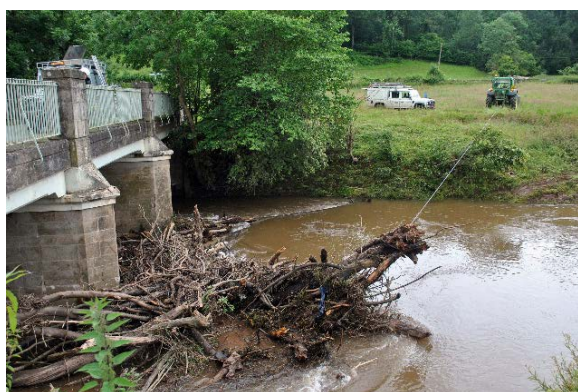
Figure 2. Large debris blockage under a bridge
