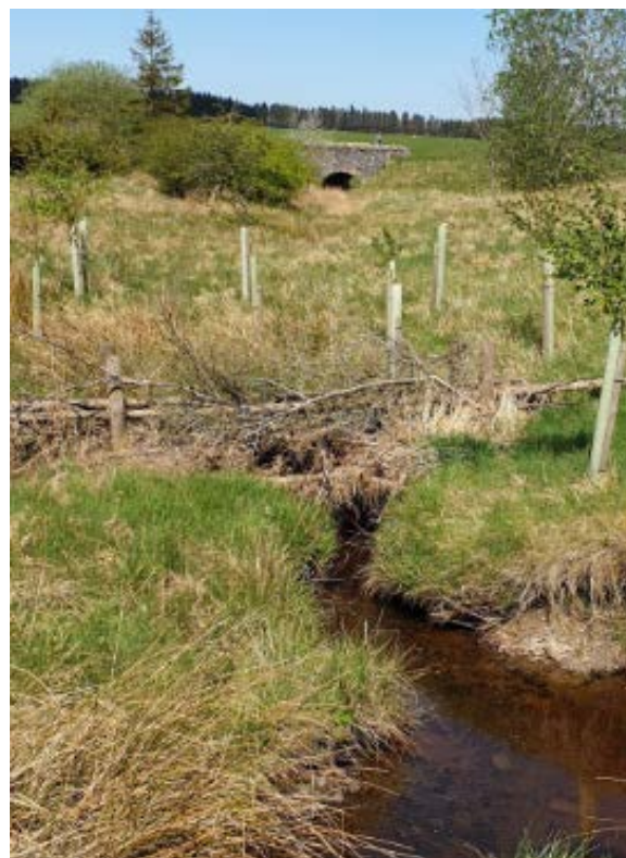
Figure 1. NFM measure: a leaky wooden barrier in Scotland. Source: Lydia Burgess-Gamble
