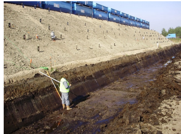
Figure 4. Sensors within a dyke – Courtesy the Rijkswaterstaat
