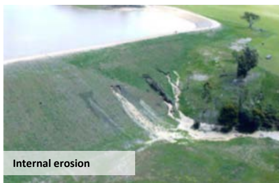
Figure 1. 3 types of erosion processes in dams and levees (photos USDA ARS, RHDHV, D Bowles / USBR/ USACE / URS / UNSW)
