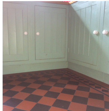
Marine ply units and tiled floors
