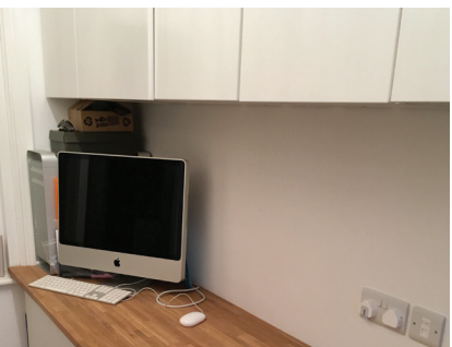
Study with wall mounted cupboards, so important documents can be stored safely above flood level
