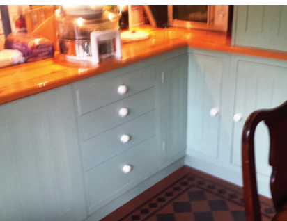
Kitchen units made of Marine Ply (these have already survived a flood event).
