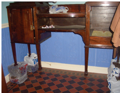
Antique furniture raised on several bricks, which are enclosed in plastic bags (to prevent water seeping up into wooden legs).
