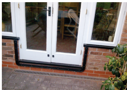
Non-standard doorway with unobtrusive barrier fittings
