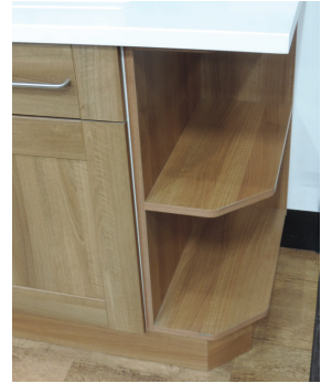
Wrap the end of units to avoid end boards that reach the floor
