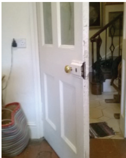
Original solid wood doors retained
