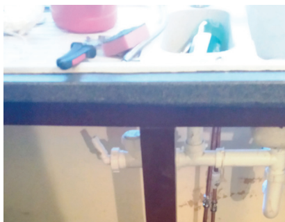
Kitchen and utility moved from basement to ground floor, and space converted to workshop use
