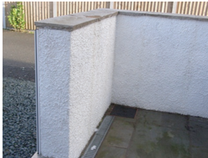
Drainage, pump and sump to get any water out again quickly.
