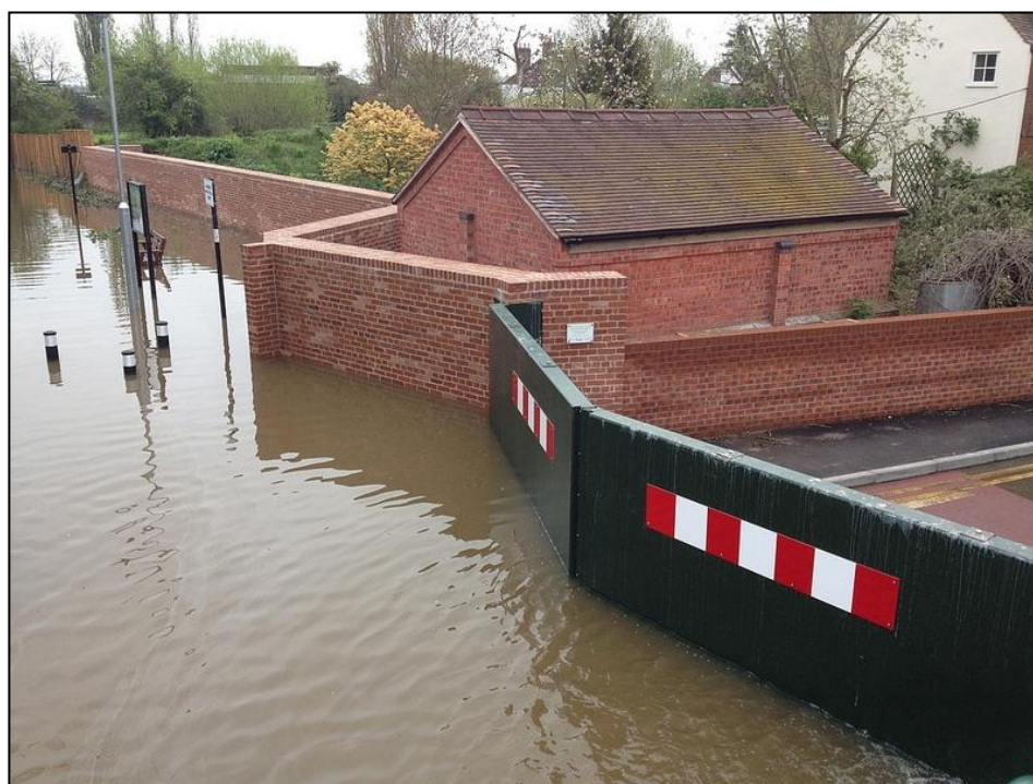
Flood gate in action at New Street, Upton upon Severn, April 2012 © Jackie Surtees
