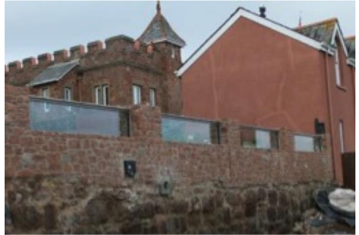
Flood glazing at Ringmore Towers © TFS Defence Doors http://www.defencedoors.com/news.htm
