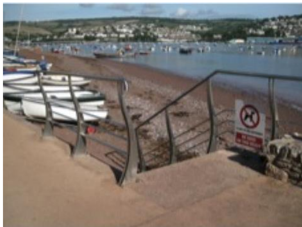
Steps and railings Marine Parade
