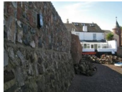
New wall on top of old, Embankment
