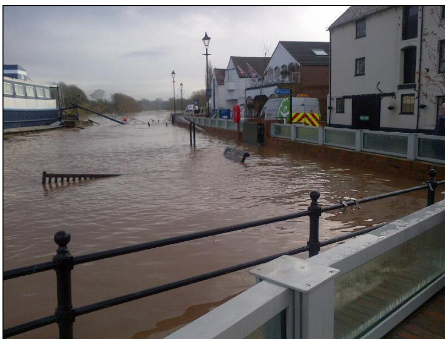
Flood defence in Upton upon Severn, November 2012 © Environment Agency
