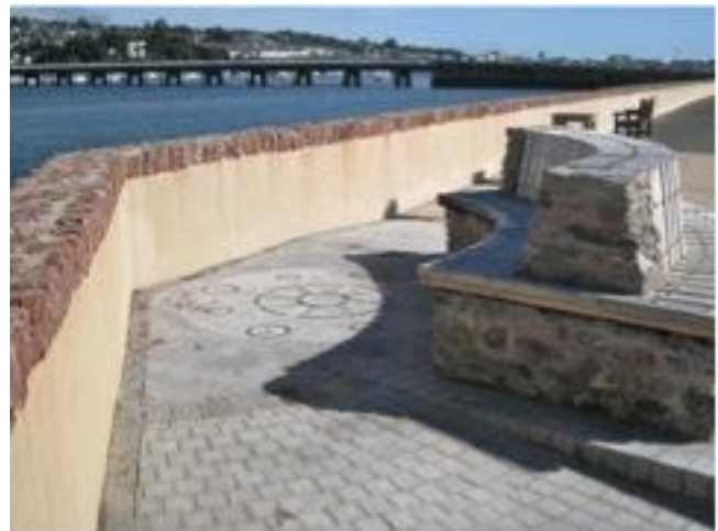
Feature seat at the Embankment
