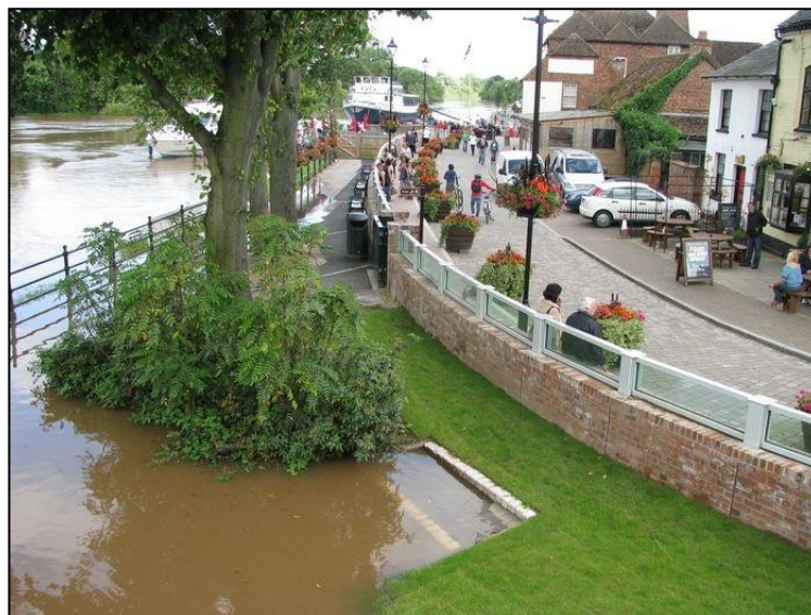
Upton upon Severn flood defence wall, July 2012 © Jackie Surtees
