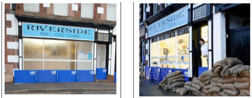
Figure 14 Flood Barriers Deployed in Appleby – with Backup Sandbags
