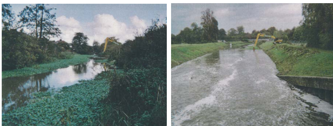
Figure 5-7 Control using long-reach excavators (courtesy Michele Cooper, Environment Agency)
