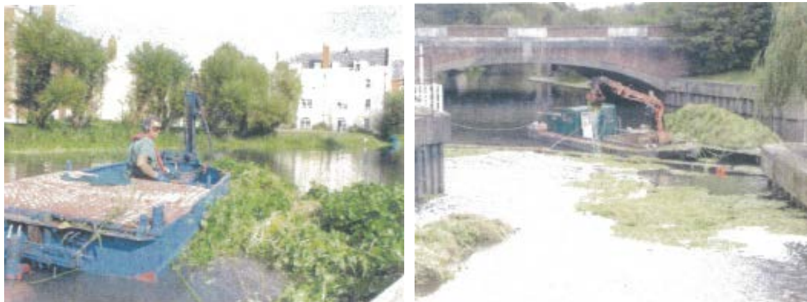
Figure 5-6 Control in September 2002 using weed boats and tugs to collect arisings at Zenith Weir (courtesy Michele Cooper, Environment Agency)
