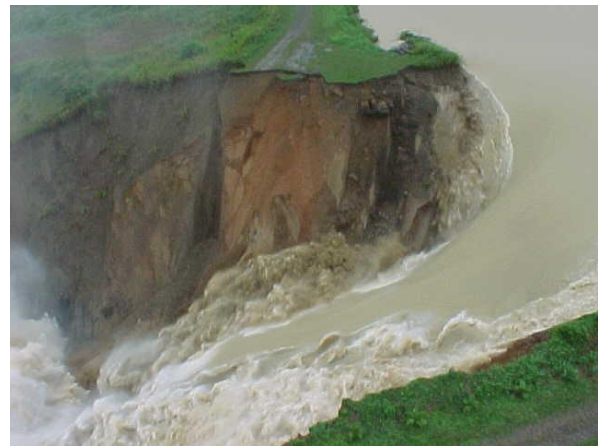
b. Vortices undercutting the breach sides just after failure of the spillway crest (El Guapo Dam, Venezuela)
