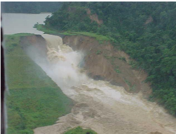
a. Headcut erosion back through dam after failure of the spillway (El Guapo Dam, Venezuela)
