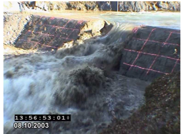
d. Soil wasting – block failure on left face of breach 2s after failure of block into breach (that is block has been removed)
