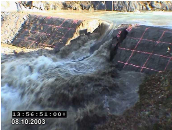
c. Soil wasting – block failure on left face of breach
