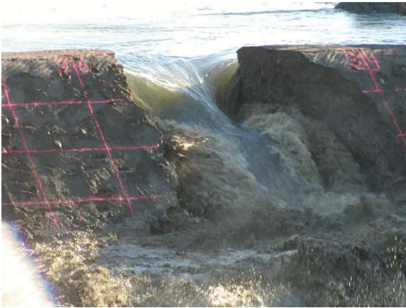
a. Sediment erosion by turbulent flow along base of breach sides
