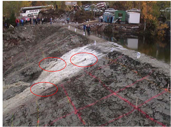
b. Mass erosion – small lumps of soil/clay being removed
