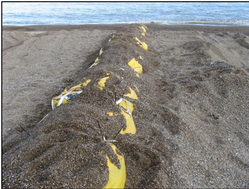
Figure 5.3 Partially completed 'hump'
