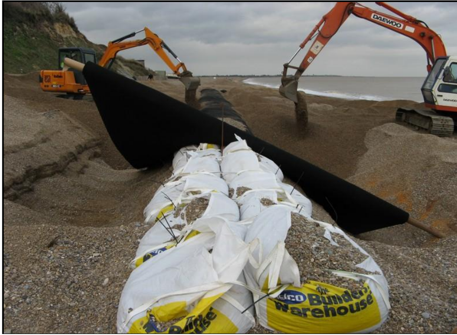
Figure 5.2 Placing geomembrane on top of bulk containers
