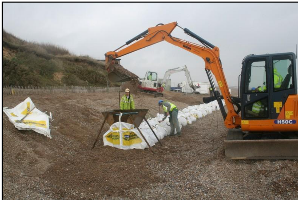
Figure 5.1 Filling and placing of the flexible intermediate bulk containers
