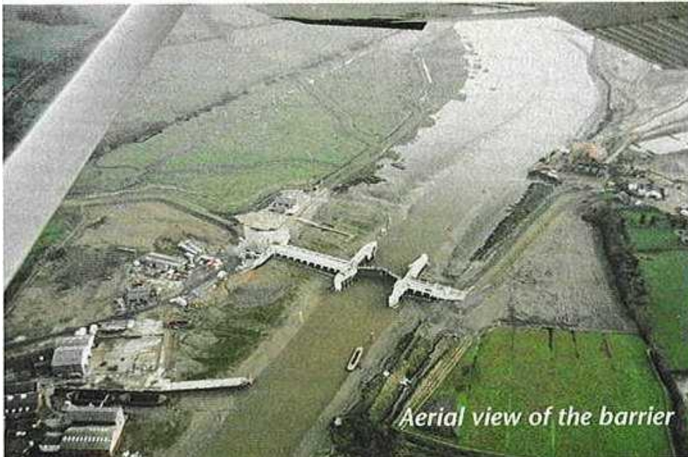
Figure 6-1 Colne Barrier (aerial view)
