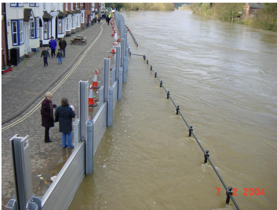
Figure 6-3 Demountable flood defence for River Sever at Bewdley
