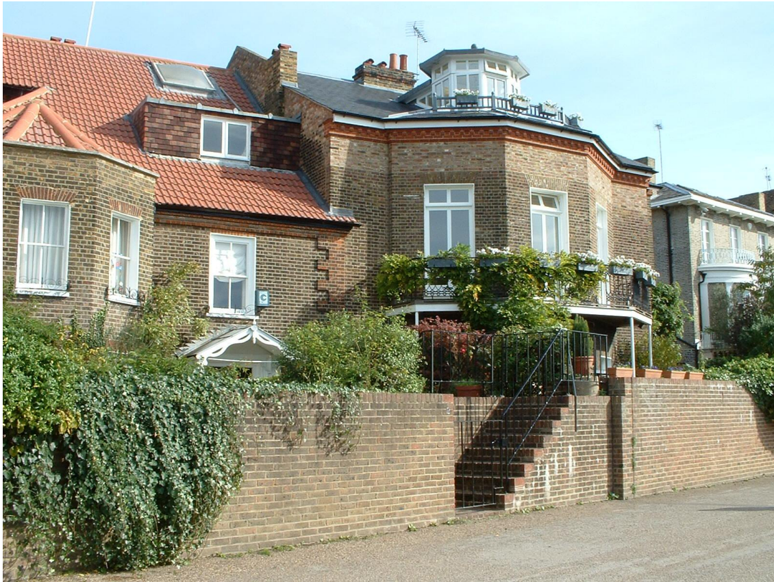
Figure A2-8 Example of frontage defence on the Thames in west London
