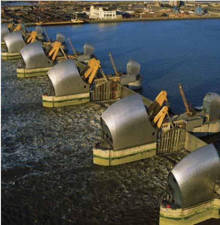
Figure 3-5 Thames Barrier, London
