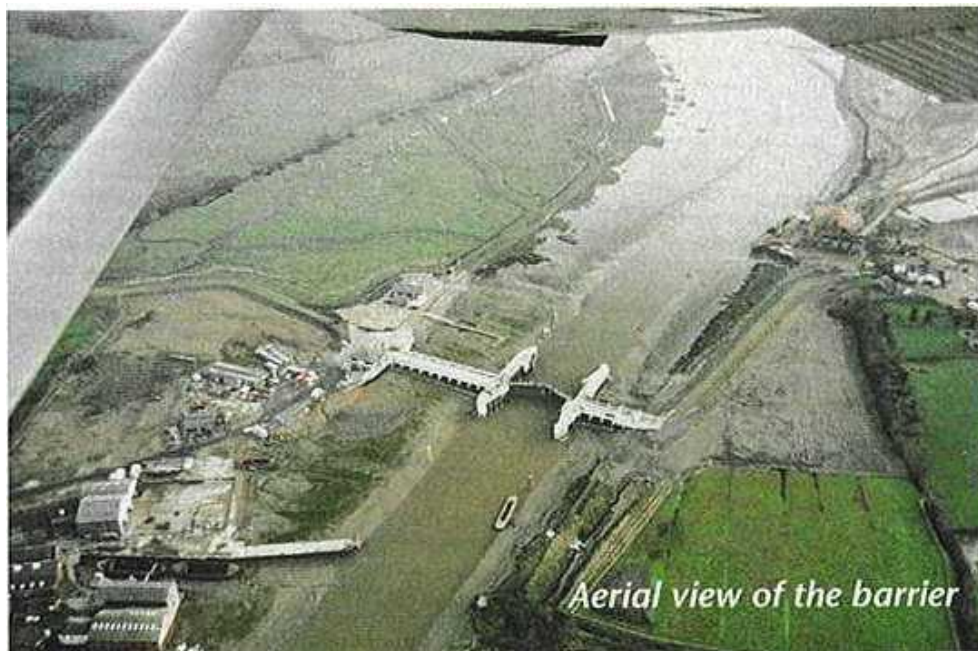
Figure 3-3 Colne Barrier (aerial view)
