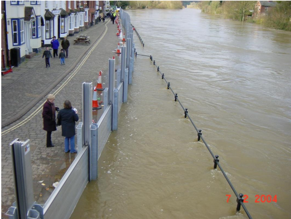
Figure 3-6 Demountable flood defences for River Severn at Bewdley
