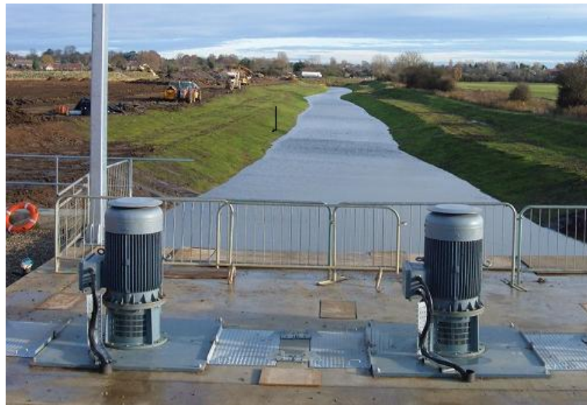
Figure 3.8: Typical vertical axial flow pump installation
