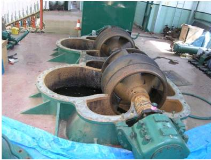
Figure 3.9: Large radial dual flow installation in flood defence application (top casing removed)
