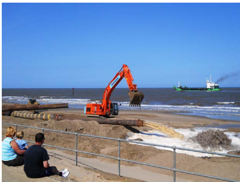
Figure C.4.4 Photograph of recharge operation (courtesy of Halcrow).
