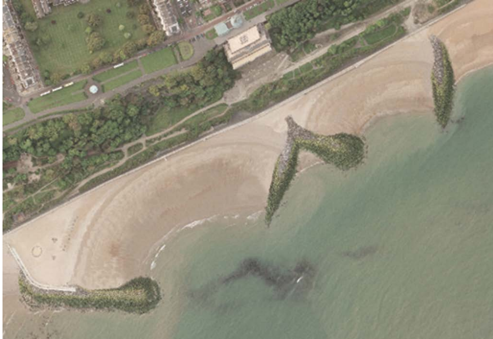
Figure 3.3 Aerial view of Folkestone scheme post-construction (from CIRIA 2010)
