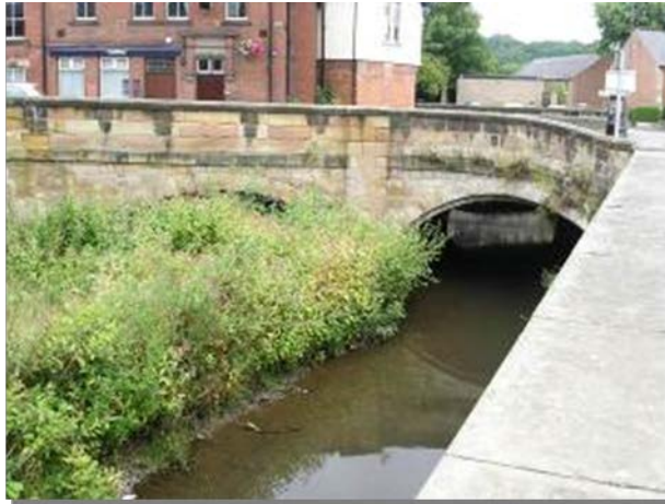
Figure 3.10 The original photograph where modelling has shown that the level of blockage is unacceptable – the ‘red’ alert.
