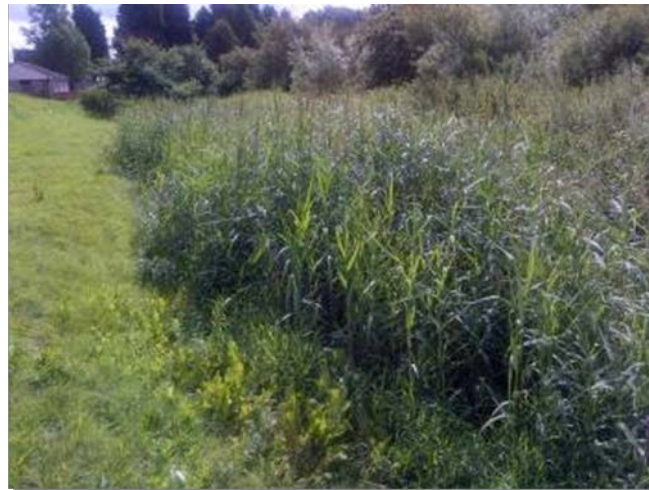
Figure 3.6 An open channel choked with aquatic plants. This is likely to cause increased water levels in flood events. This should be highlighted in view of the location of the adjacent property.
