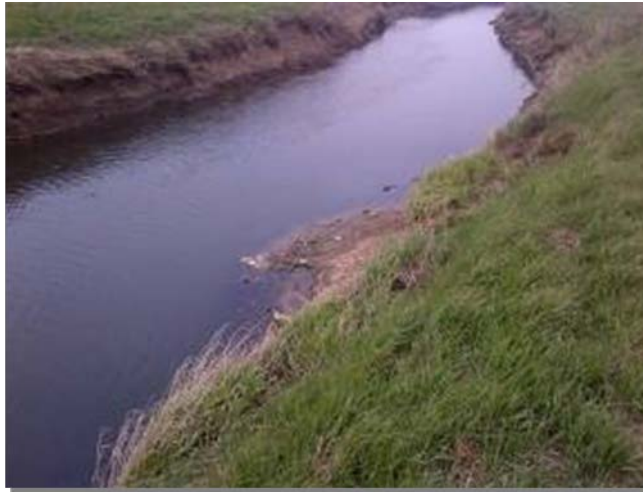
Figure 3.2 Minor transient shoaling, which is likely to have an insignificant effect on flood levels in peak floods.
