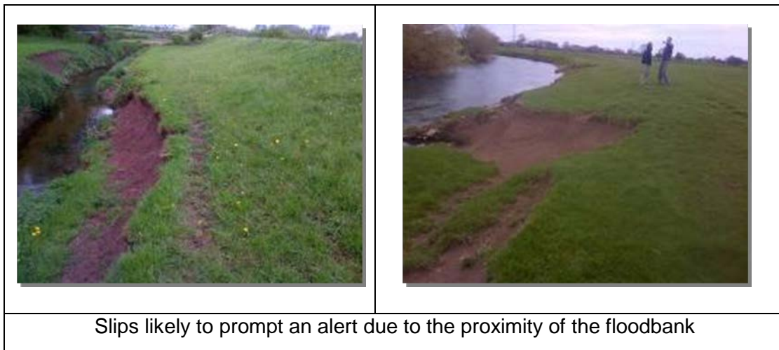
Figure A.5.1 Typical evidence of slope instability
