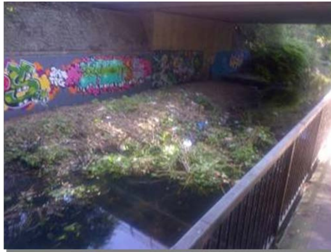
Figure 3.5 An urban open channel. The permanent vegetated shoaling will affect conveyance. The acceptability of this can only be assessed by considering the risks posed to nearby and upstream receptors by an increase in water levels. The channel may be over-widened at this bridge and channels will often silt up to regain a normal width.
