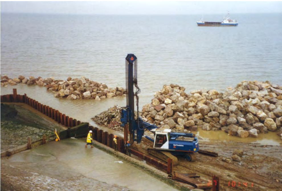
Figure C10.7 Pile driving
