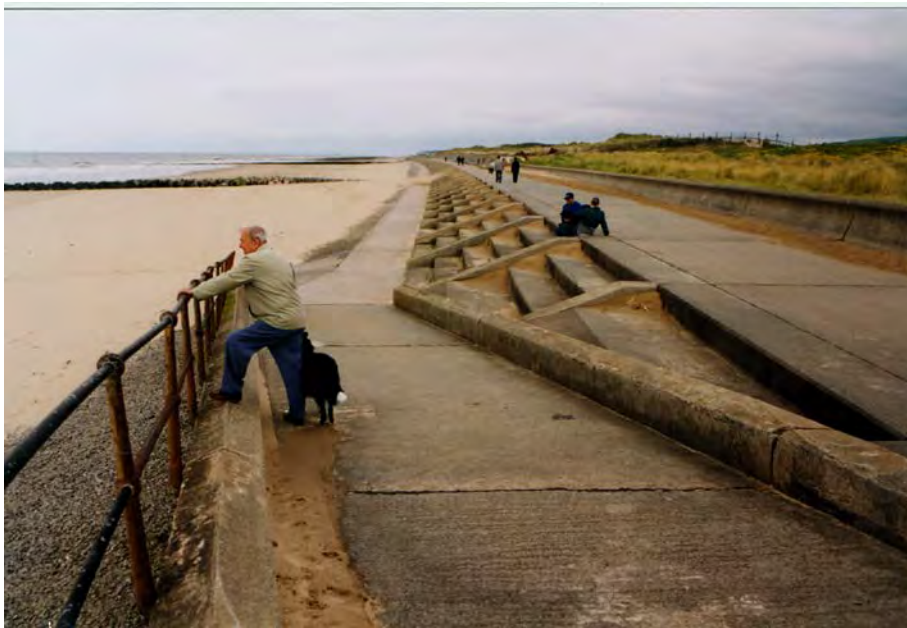
Figure C11.2 Sloping asphalt apron and rock groynes in front of steeped concrete seawall
