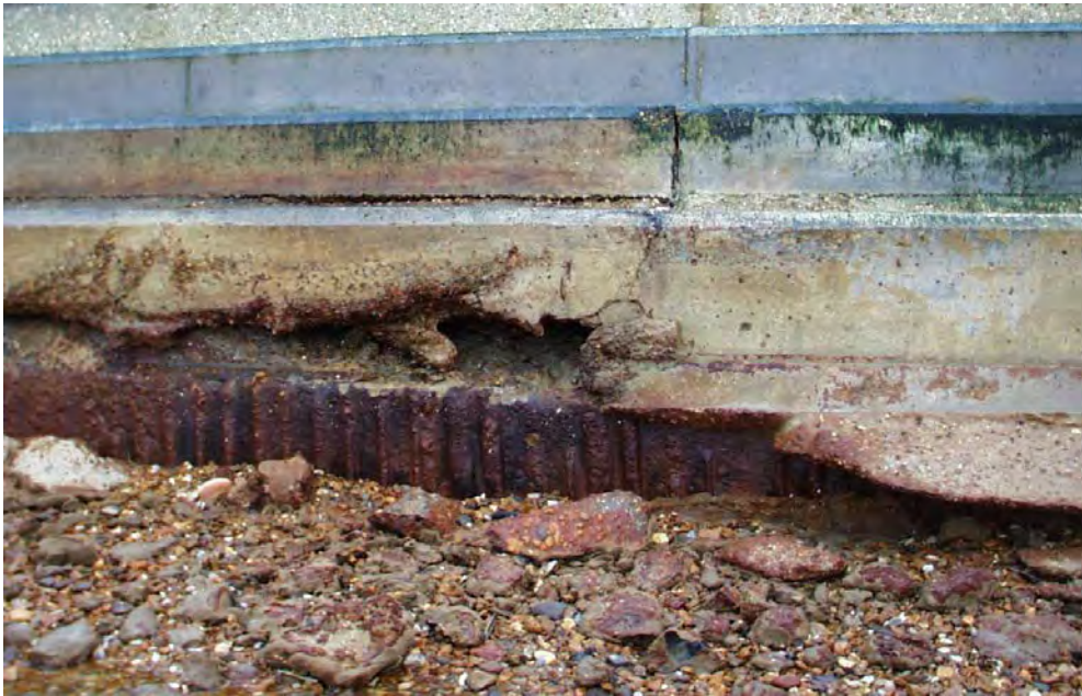
Figure 4.2 Beach that has reached trigger level prior to repair and recharge (courtesy Poole Borough Council)
