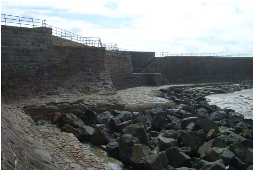
Figure 5.18 Example of rock apron (courtesy Jersey States Government)
