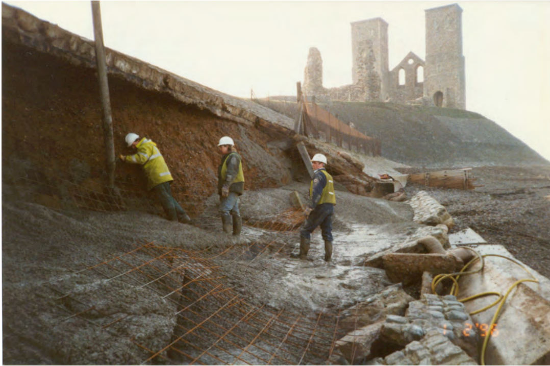
Figure C10.4 Emergency repair works, 1996
