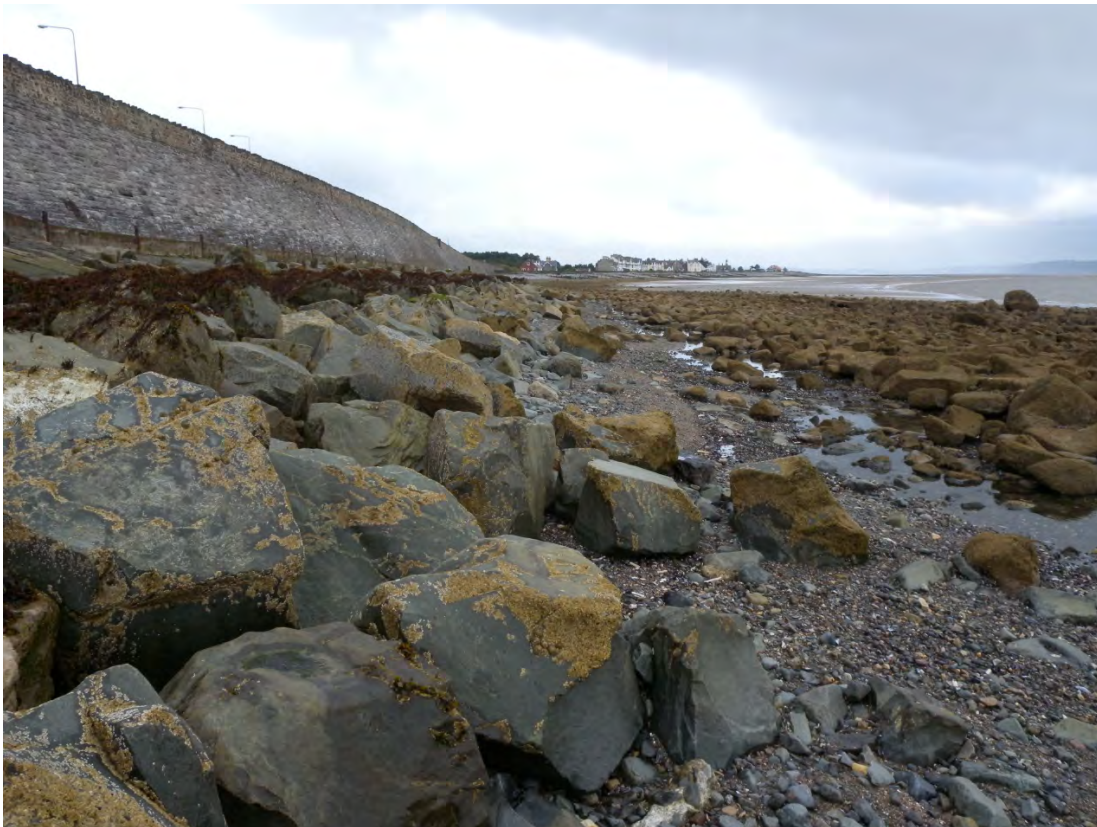
Figure 4.15 Armour displaced from a rock toe, Llanfairfechan, North Wales (courtesy Alan Williams)
