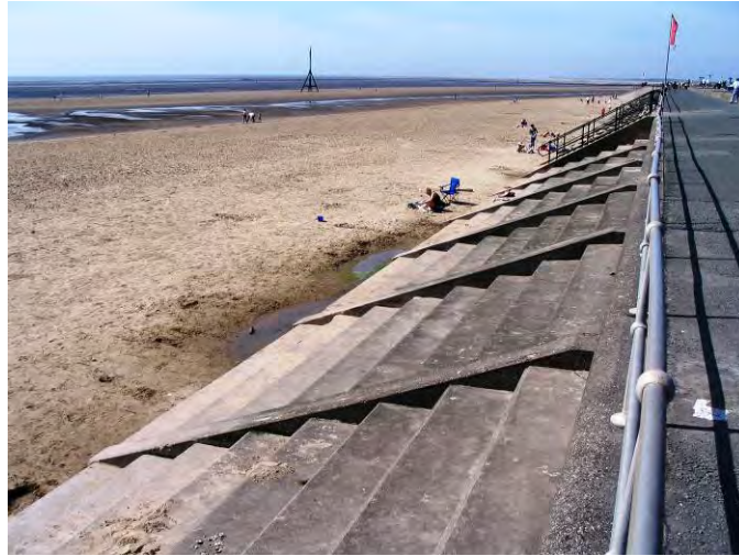
Figure 2.9 Concrete stepped revetment, Crosby, UK (courtesy Sefton Council)
