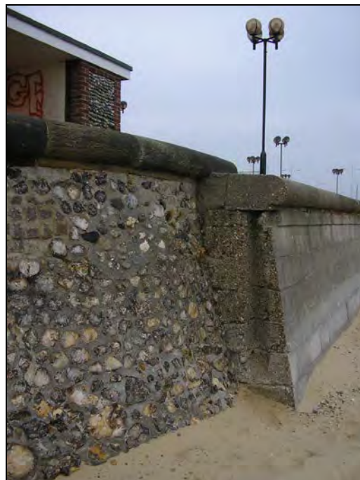
Figure C3.3 Old Flint Wall and concrete wall
