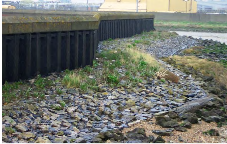
Figure 2.13 Grouted stone toe apron, Thames Estuary (courtesy HR Wallingford)
