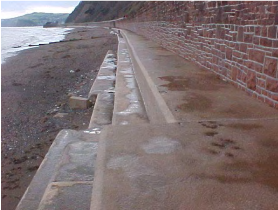
Figure C7.4 Full foundation strengthening, Smugglers Cove to Sprey Point
