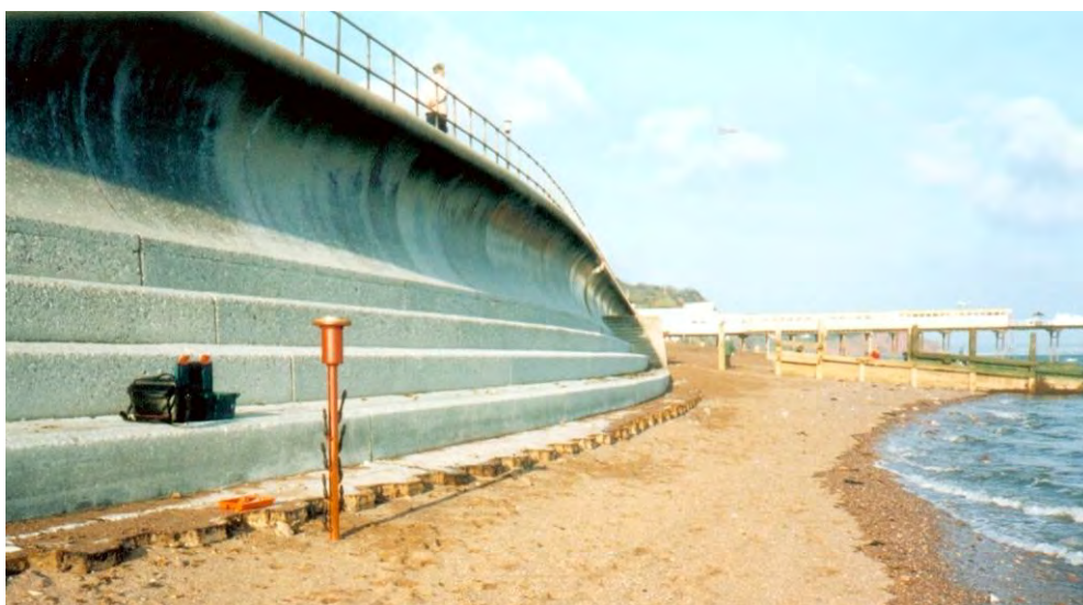
Figure 3.23 Scour monitors in operation on a shingle beach to obtain data on within tide changes in bed levels (courtesy HR Wallingford)
