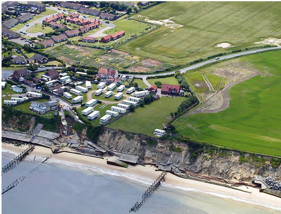
Figure C2.4 Failure of the seawall in winter 2000–2001
