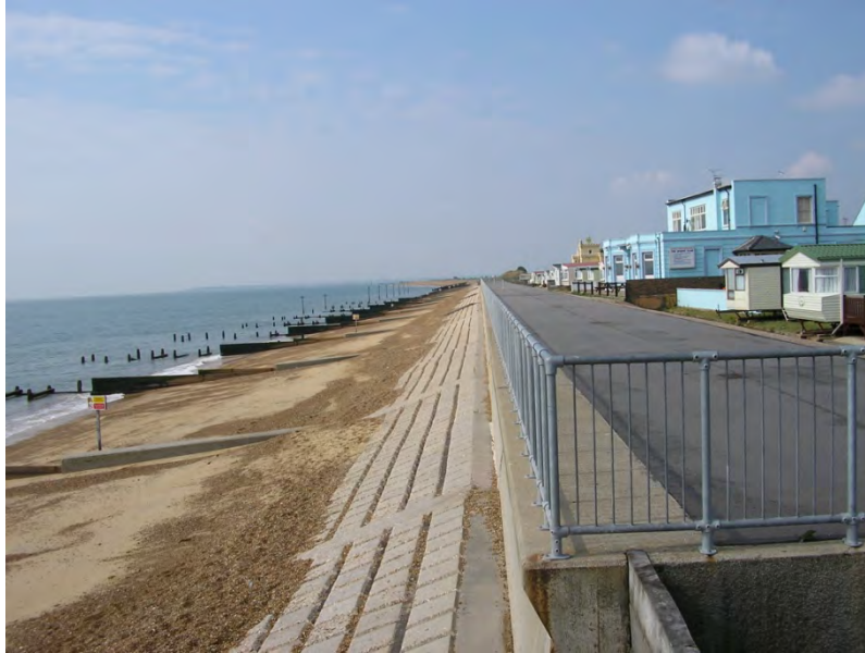
Figure C8.4 Environment Agency seawall and flood defence, 2005
