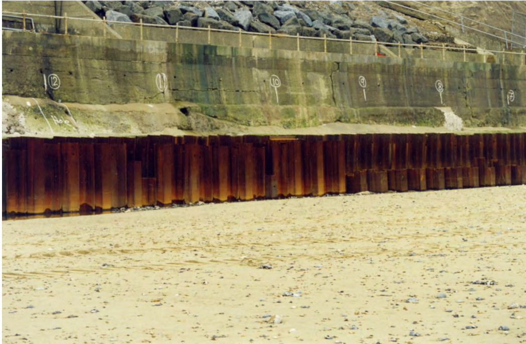
Figure C5.3 The original wall
