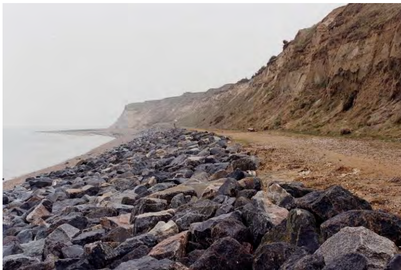
Figure 2.10 Supplemental rock armour revetment (courtesy of HR Wallingford)
