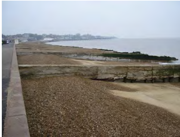
Figure C8.2 Seawall and groynes at the SCDC frontage, 2005
