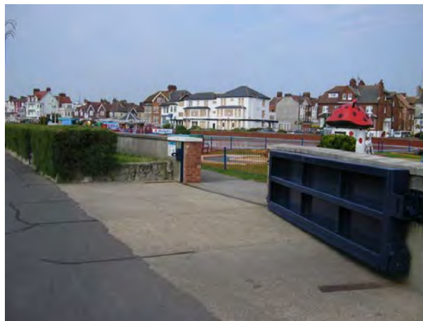
Figure C8.3 Floodwall and gate
