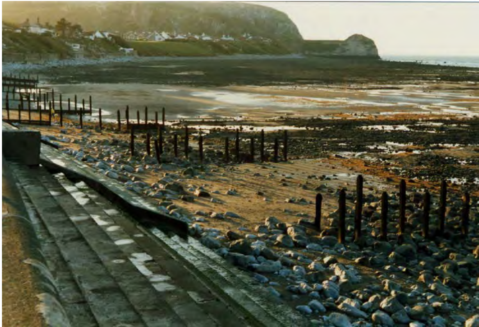
Figure C14.2 Lowered beach exposing shore platform
