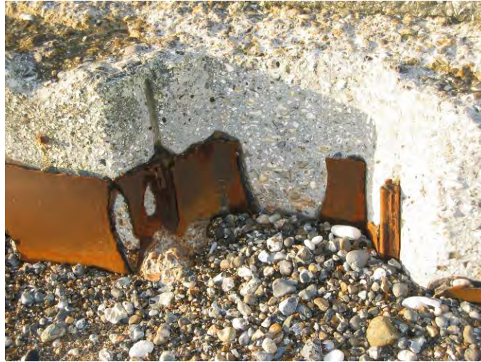
Figure 4.23 Complete loss of section of sheet piles in an area exposed to sediment movement
