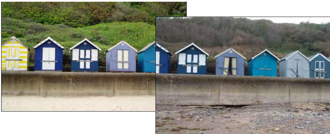
Figure A.3 Storm event sediment scour (right) and post event recovery (left) (courtesy of Peter Frew, NNDC)
