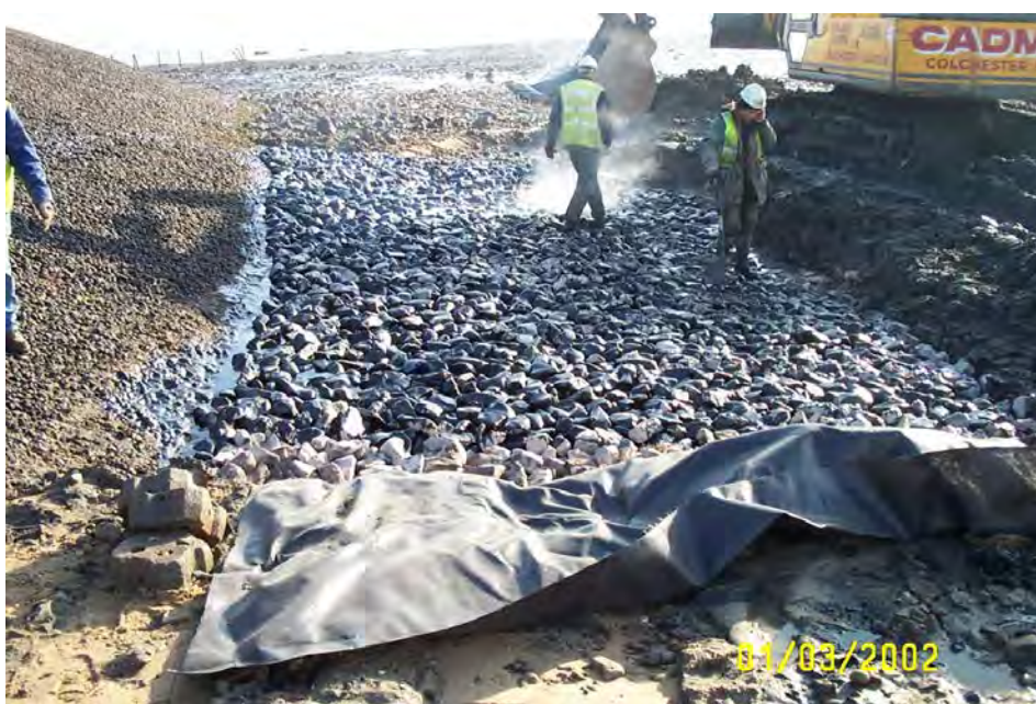
Figure C6.7 Toe construction
