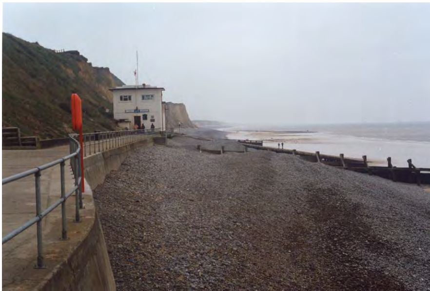
Figure A.17 Accumulation of shingle at updrift end of seawall, Sheringham, Norfolk
