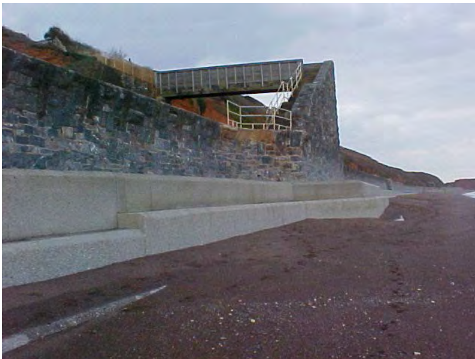
Figure C7.5 Full foundation strengthening – Rockstone footbridge
