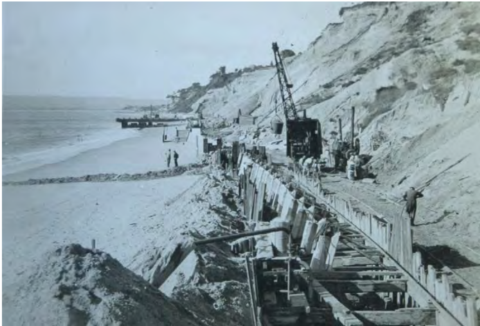
Figure 3.8 Promenade wall under construction (courtesy Poole Borough Council)
