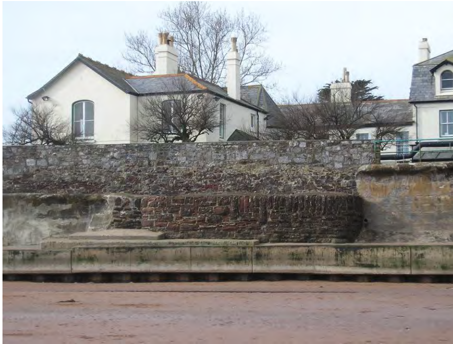
Figure 5.2 Goodrington Sands Seawall, Paignton (courtesy of ENBE)
