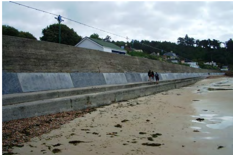
Figure 2.14 Concrete toe beams (courtesy HR Wallingford)
