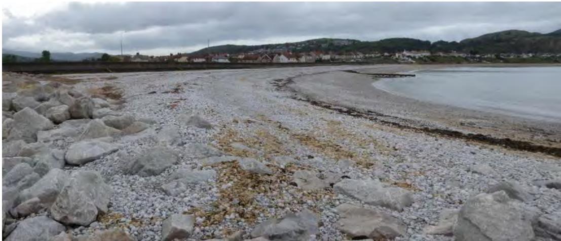
Figure C14.4 View from easterly groyne (CEUK)
