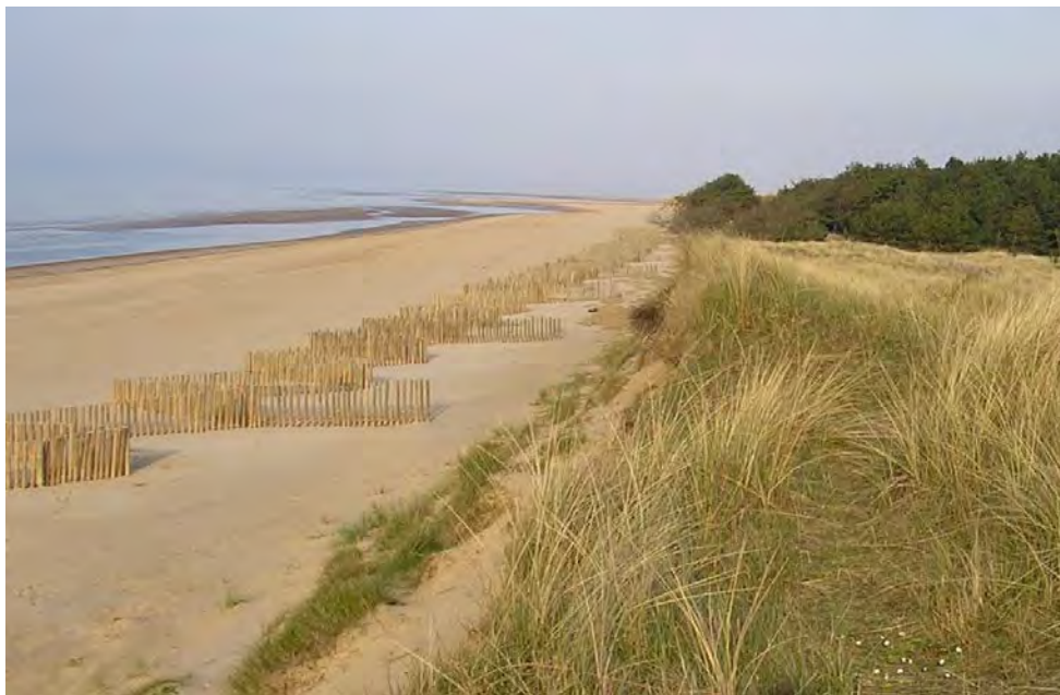
Figure C4.2 The site in 2009 – note the recently installed brushwood dune protection
