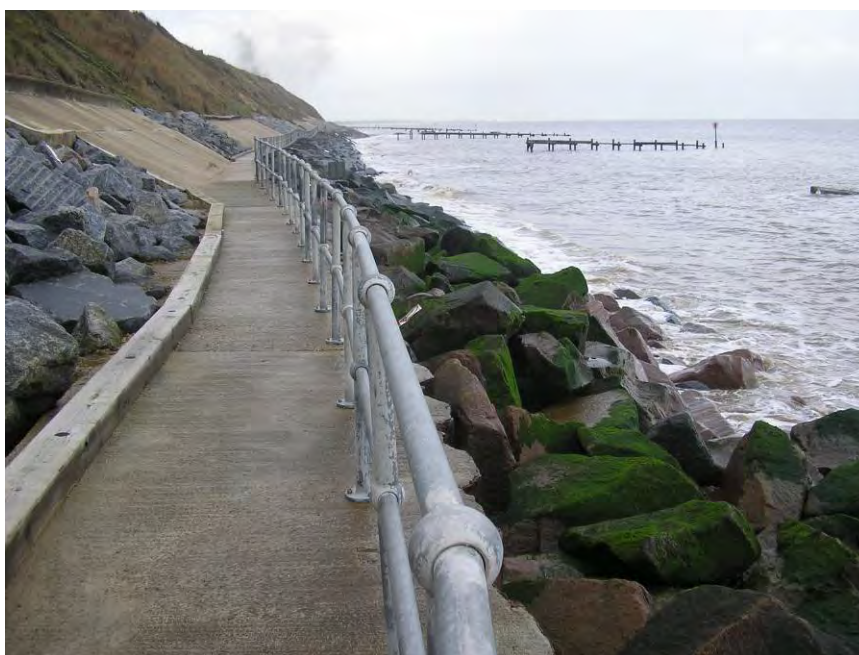
Figure 5.13 Example of rock used to provide passive support
