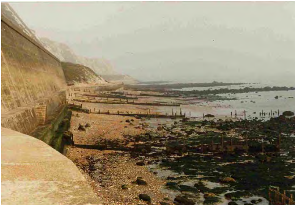
Figure A.7 Beach and shore platform lowering, Shakespeare Cliff, Thanet
