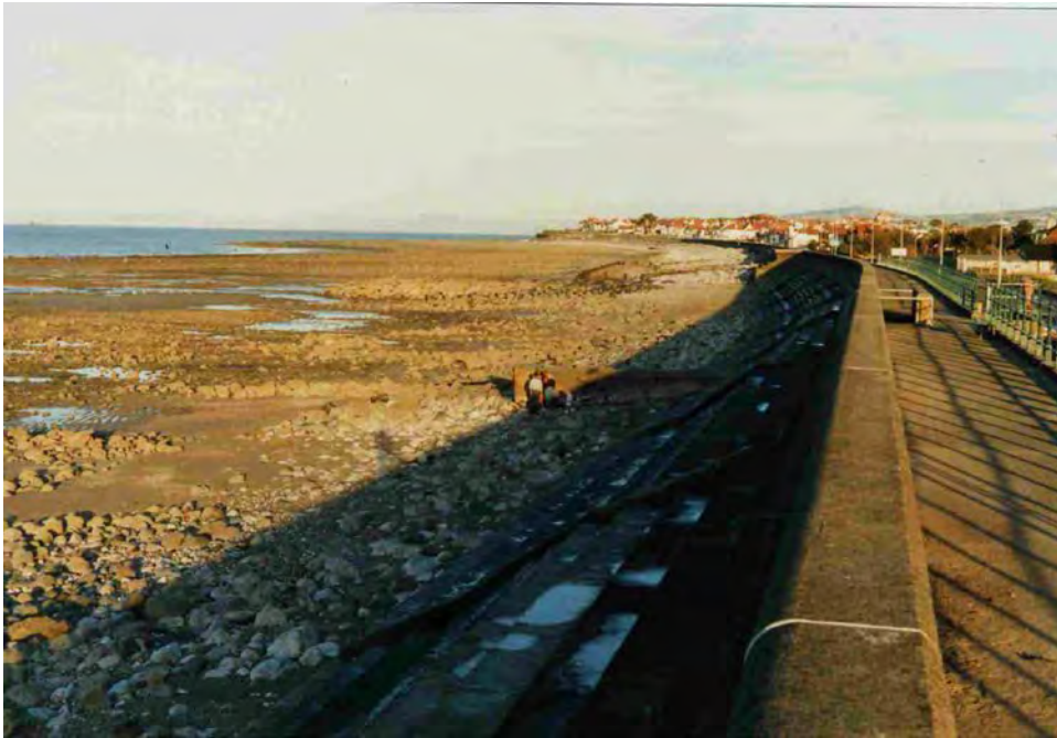
Figure A.8 Removal of beach sediments from shore platform, Penrhyn Bay
