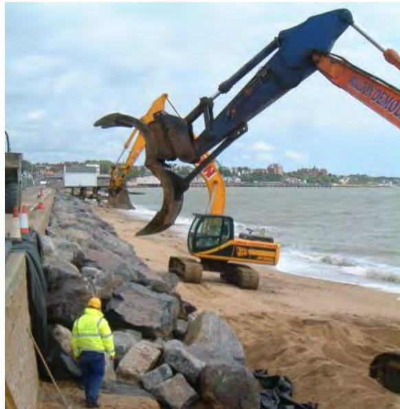
Figure C8.7 Emergency repairs to the seawall, 2007
