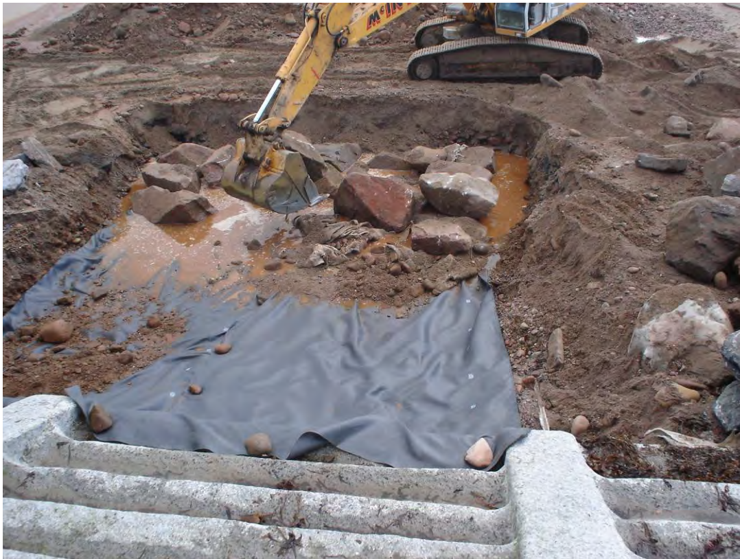
Figure 5.17 Geotextile being incorporated as part of a toe structure
