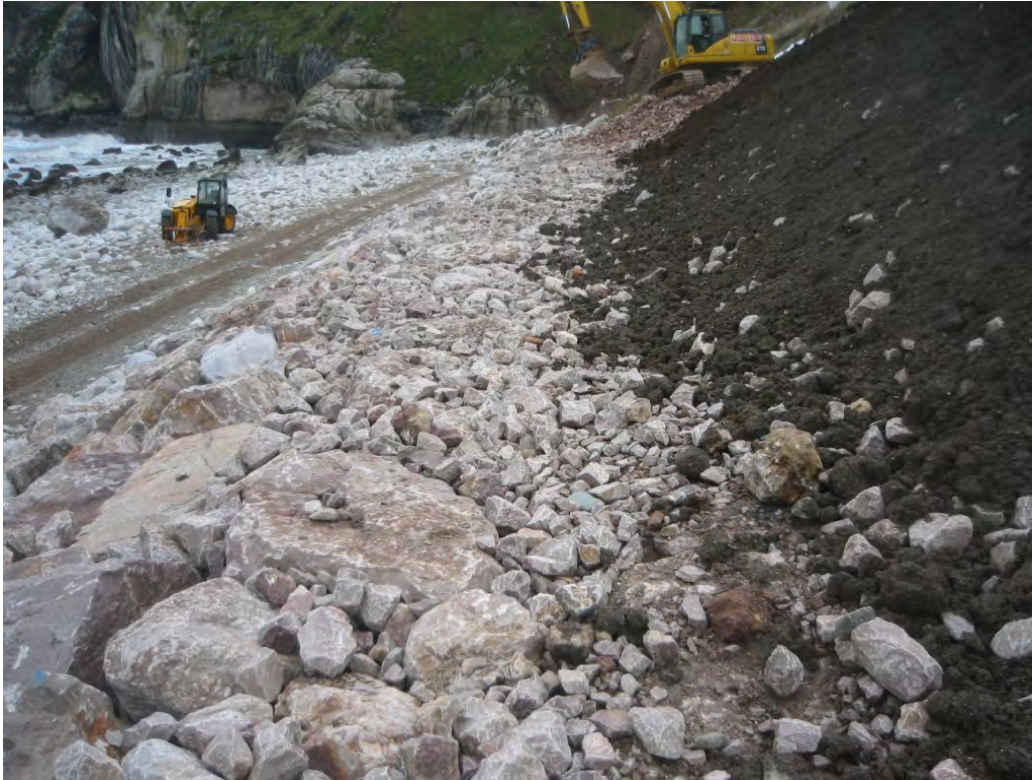
Figure C1.7 Construction in progress
