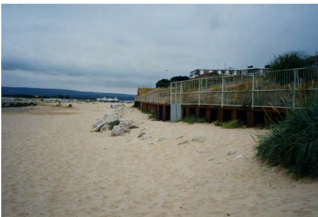
Figure C15.2 Widened beach after installation of sill and rock groynes, 2002
