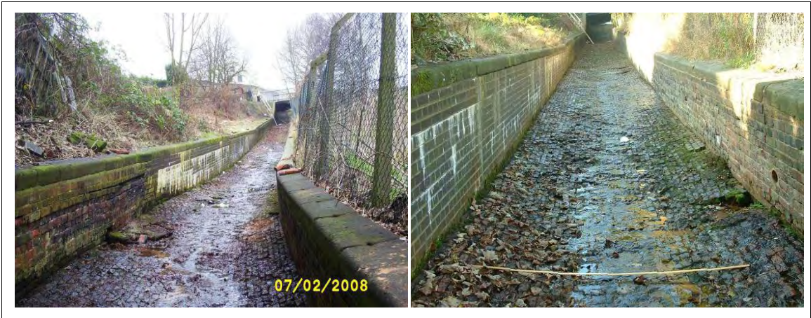
Figure 5.13 Channel invert before repairs
