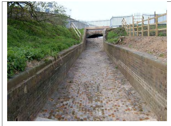
Figure 5.14 Repaired spillway channel
