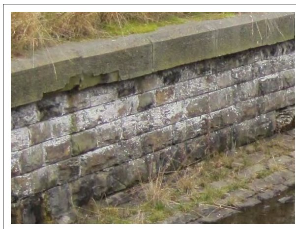
Figure 2.11 Example of coursed dressed stone masonry laid horizontally with ashlar masonry copings
