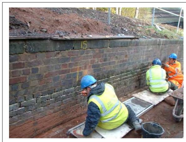
Figure 5.16 Repointing of original brickwork with lime mortar
