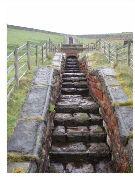
Figure 2.3 An example of a stepped bed in a masonry spillway. The wall masonry is laid horizontally.
