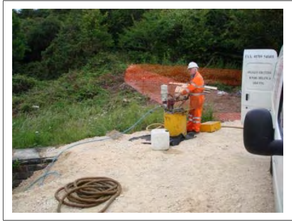
Figure 5.9 Plant for pressure pointing
