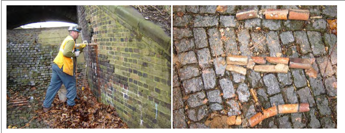
Figure 5.15 Cores being extracted from the side wall to determine thickness
