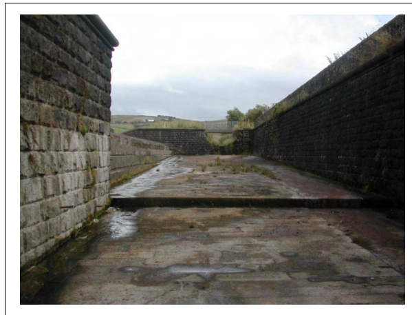
Figure 5.19 Replacement of masonry invert with concrete slab
