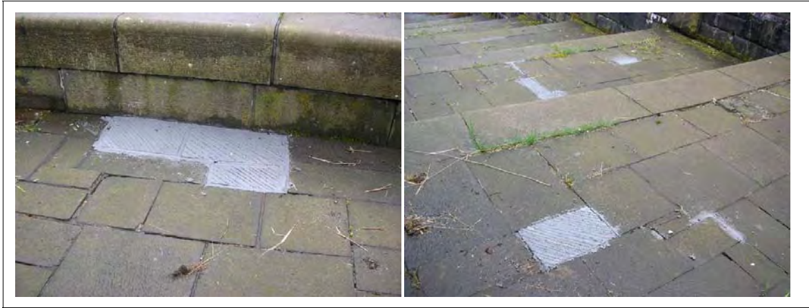
Figure 5.21 Replacement of missing masonry invert blocks with concrete
