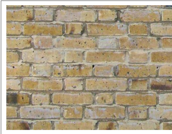
Figure 2.13 Example of Flemish bond masonry
