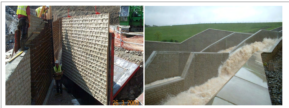
Figure 5.17 Examples of masonry replacement using textured concrete
