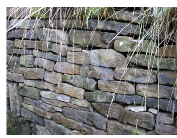
Figure 2.6 Example of dry stone wall masonry
