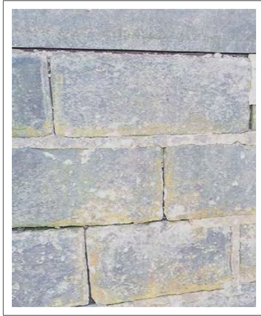
Figure 2.9 Example of coursed stone masonry
