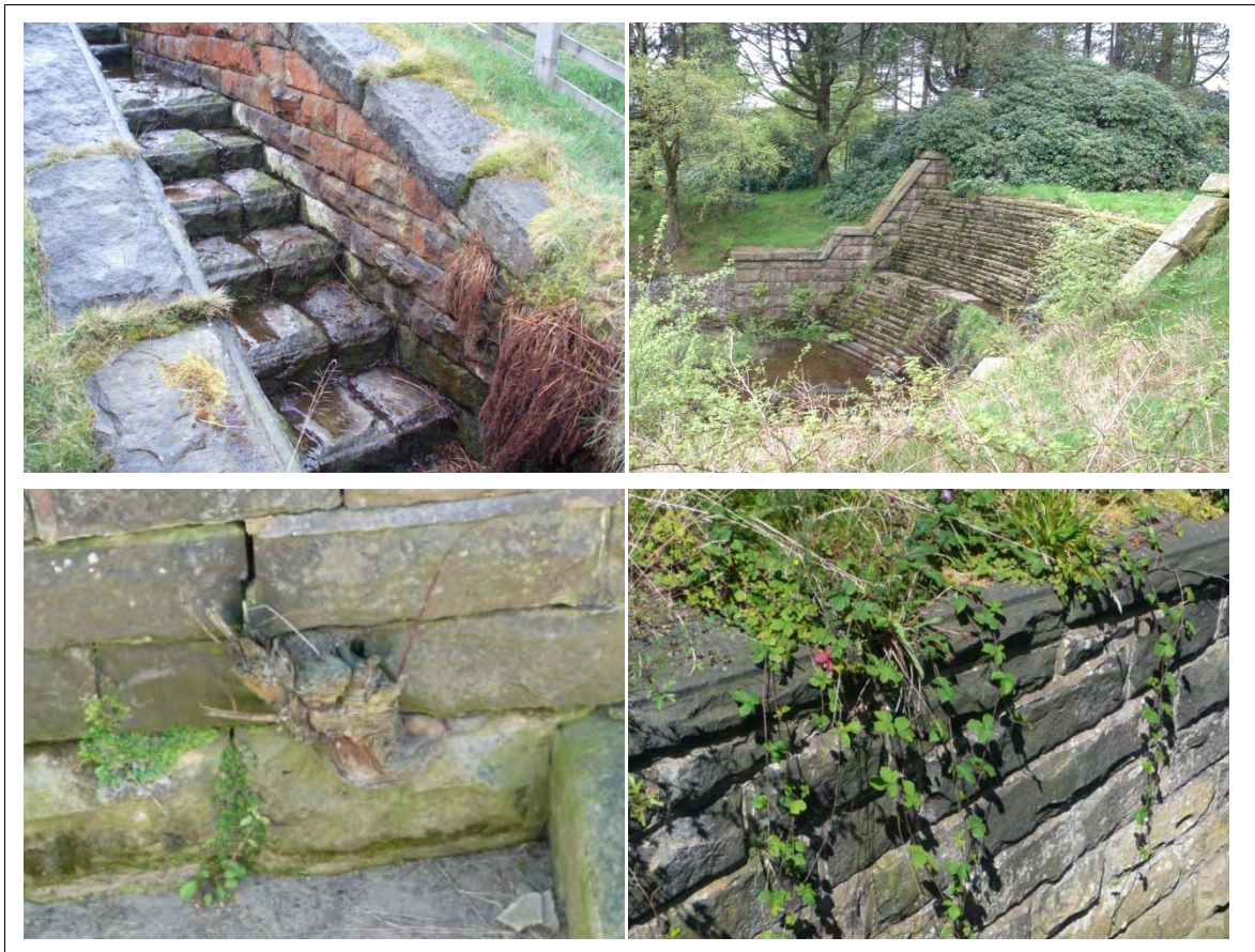
Figure 2.19 Examples of vegetation growing in or on stepped masonry spillways
