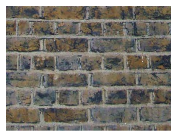
Figure 2.14 Example of English bond masonry
