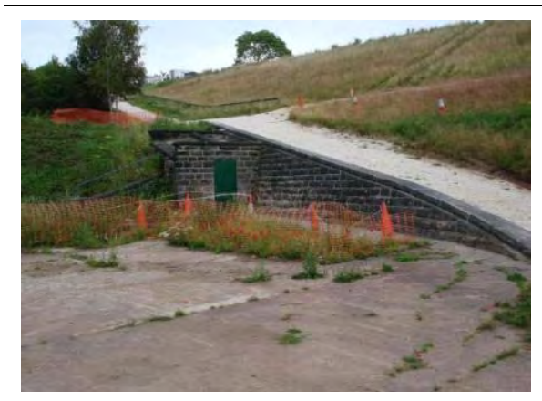
Figure 5.11 Completed wall – spillway behind has been infilled
