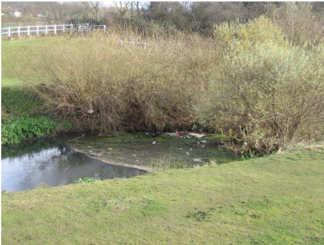
Plate 3.3 Cross Section 4 of River Dearne showing encroaching vegetation growth on berms and banks
