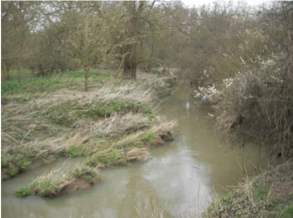
Plate 4.16 River Arun showing local bank failure which may help to narrow overwide reaches over time.
