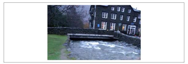
Figure 6.2 Example of limited capacity of a bridge due to sediment deposition (water depth about 30 cm)
