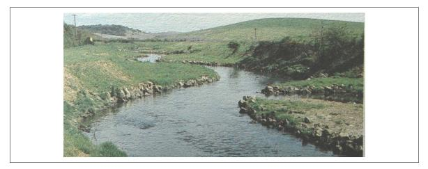
Figure 5.4 Channel narrowed by rock revetment
