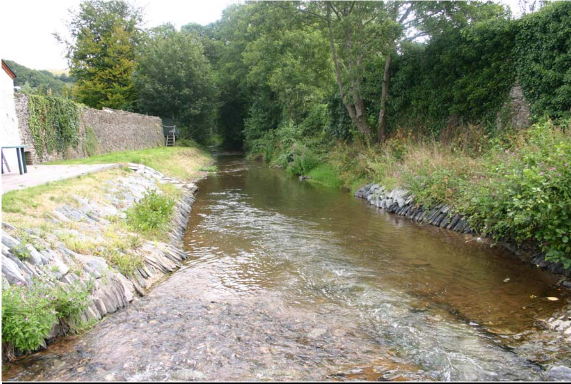
Plate 3.10 River Harbourn showing some of the works carried out in the centre of Harbertonford
