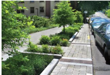
Above: SuDS street planters Source: http://www.portlandonline.com
