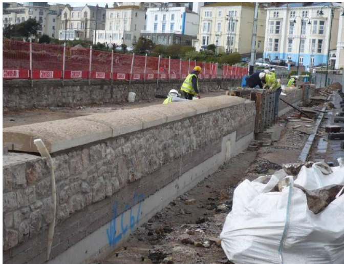
Figure 4. Phase 3. Splash Wall. Photography courtesy of the Environment Agency
