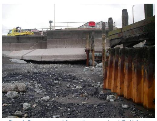
Figure 3. Toe scour to sea defence at the promenade and dilapidation to groynes. Photograph courtesy of Gwynedd Council
