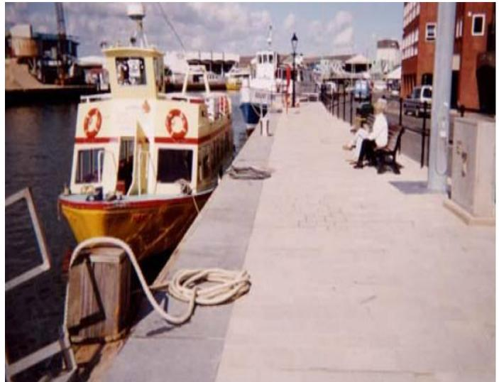
**Figure 1. Poole sea defences - raised quayside section. Photograph Courtesy of the Environment Agency**
