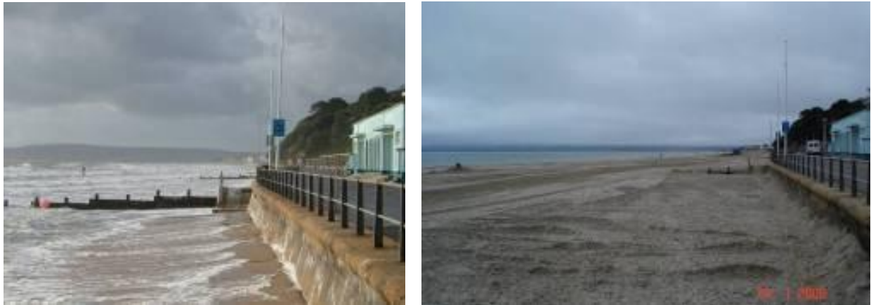
Figure 4. – Before and after the beach replenishment at Poole. Source: David Robson, Borough of Poole Council, 2010
