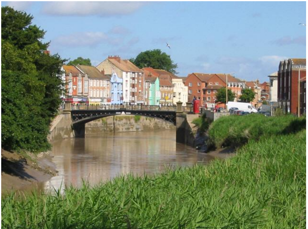
Image of Bridgwater Town Bridge taken from Wikipedia.org, Ken Grainger, 2007
