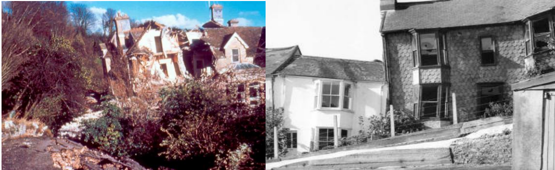
Figure 5. Cliff House 1962 (left) and the Cobb (right). Images courtesy of the Environment Agency
