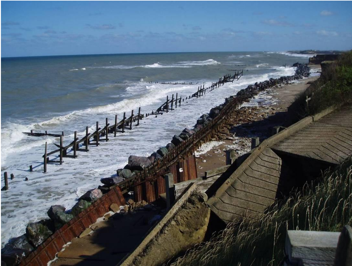
Figure 7. View of dilapidated defences, post construction of rock revetment (2007). Photography courtesy of North Norfolk District Council
