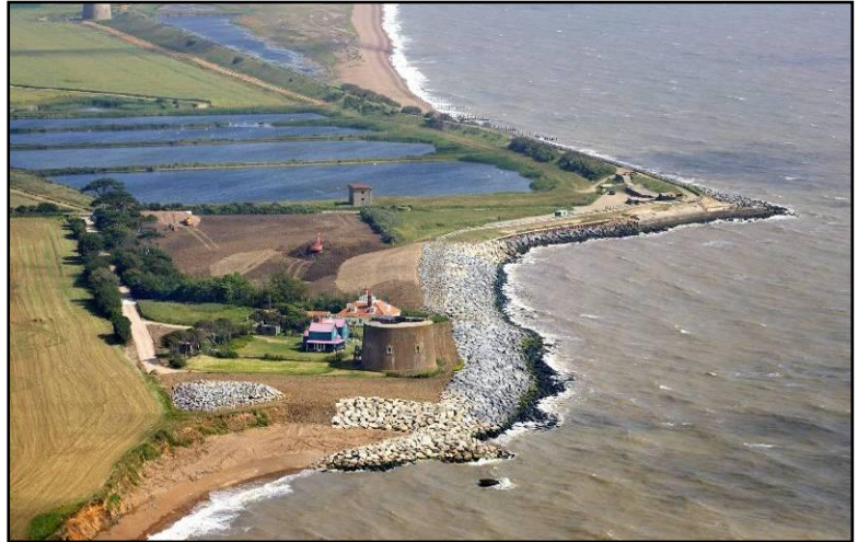
Figure 5. East Lane, Bawdsey Coast Protection and Flood Defence Completed Scheme. Source: M Page
