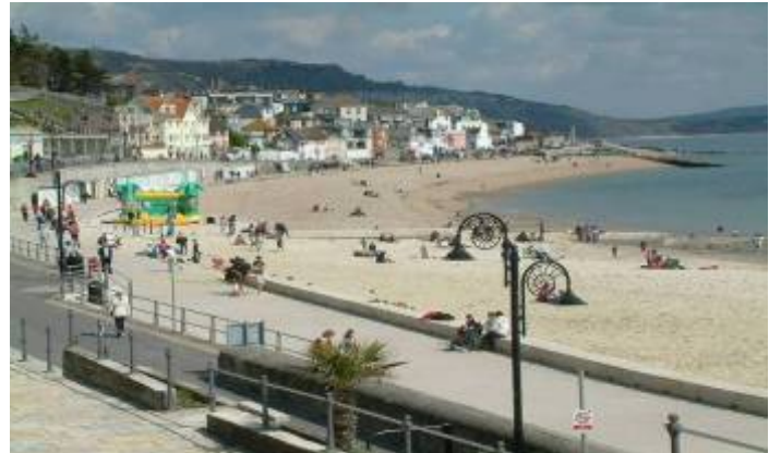
Figure 11. Completed seawall, beach and jetties.
