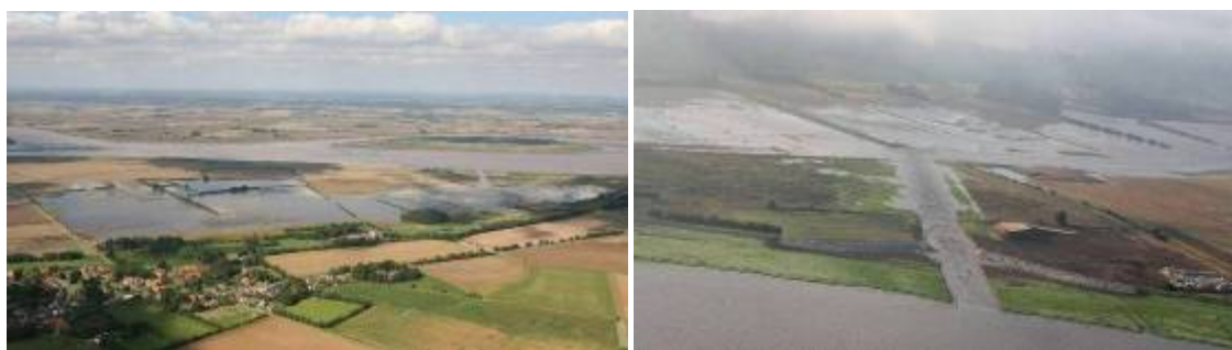
Figure 1. Alkborough Flats Managed Realignment - breach to the right.
