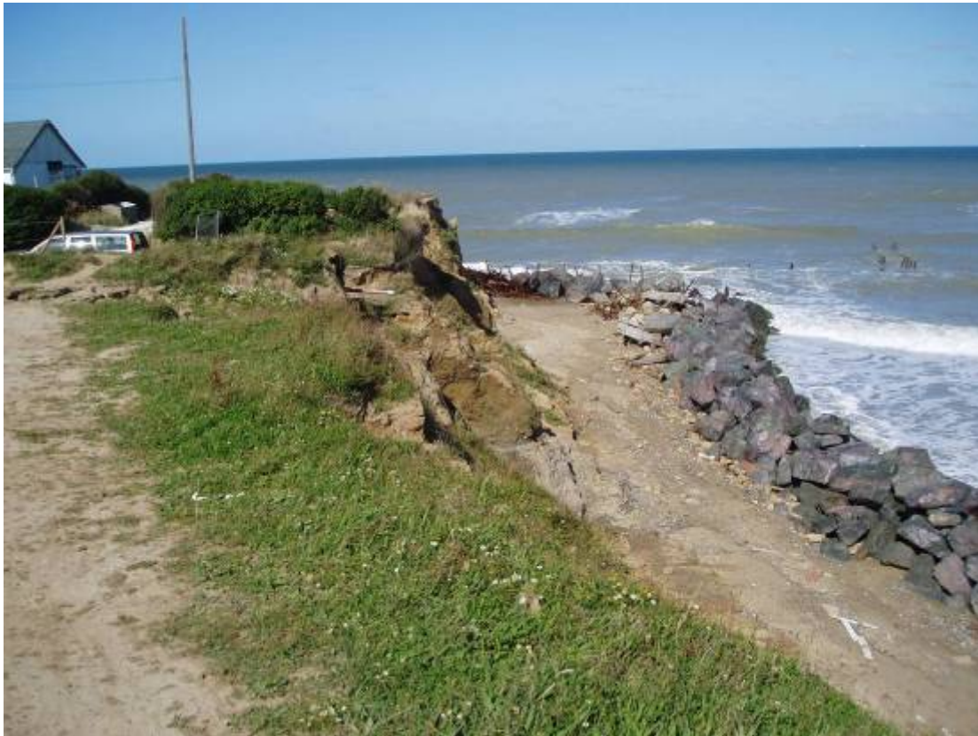
Figure 8. Rock revetment in place at southern end (2007)
