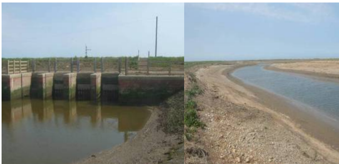
Figure 2. New sluices to allow more rapid floodwater evacuation (left) and the completed new channel (right).
