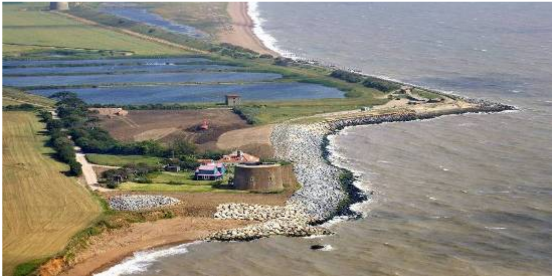
Figure 6. East Lane, Bawdsey Coast Protection and Flood Defence Completed Scheme.
