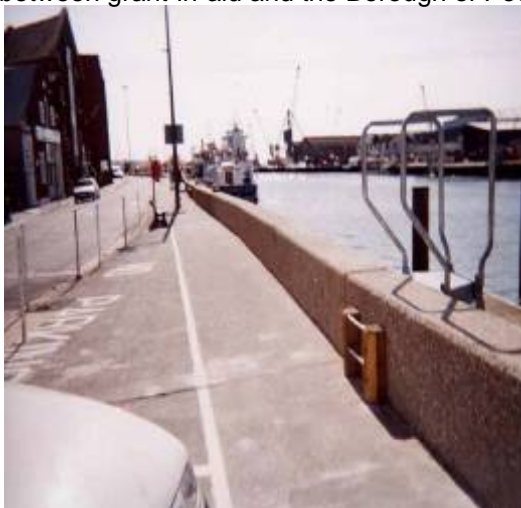
Figure 14. Poole sea defences - long floodwall section.
