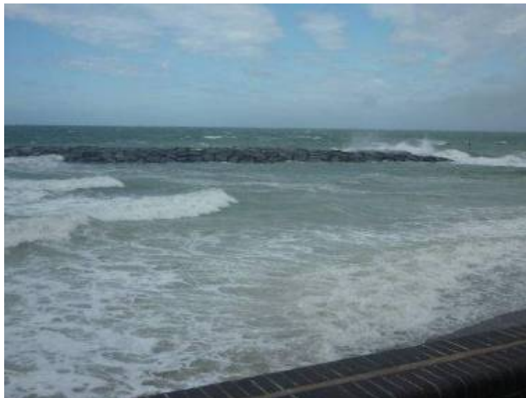
Figure 18. New installed break-water part of unique feature.
