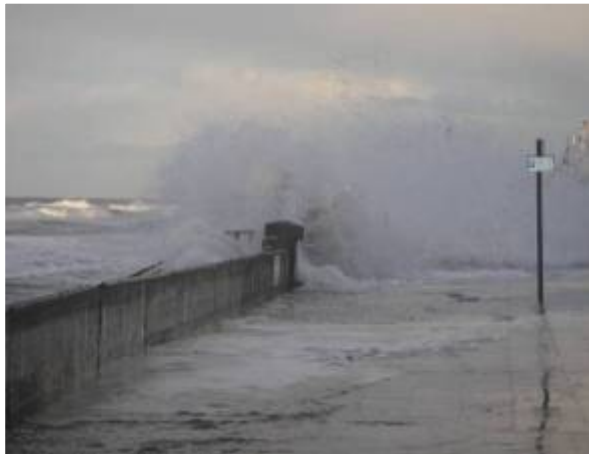
Figure 16. Overtopping at Esplanade on 1 March 2006.
