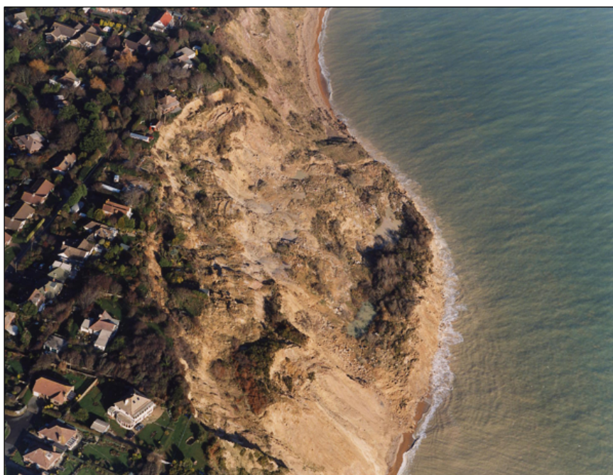
Cliff exposed to wave attack and erosion (2004). Source: Terry Oakes Associates
