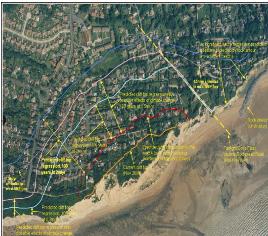
No active intervention scenario – Prediction for Long Term Recession (1998 aerial). Source: Terry Oakes Associates
