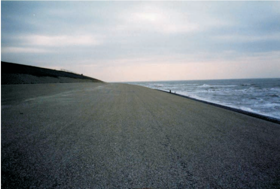
Fig. 5.16: Dike covered by asphalt (photo: SCHÜTTRUMPF)
