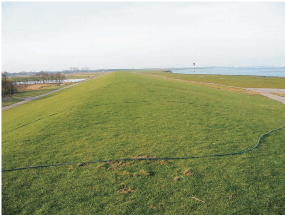
Fig. 5.15: Dike covered by grass (photo: SCHÜTTRUMPF)
