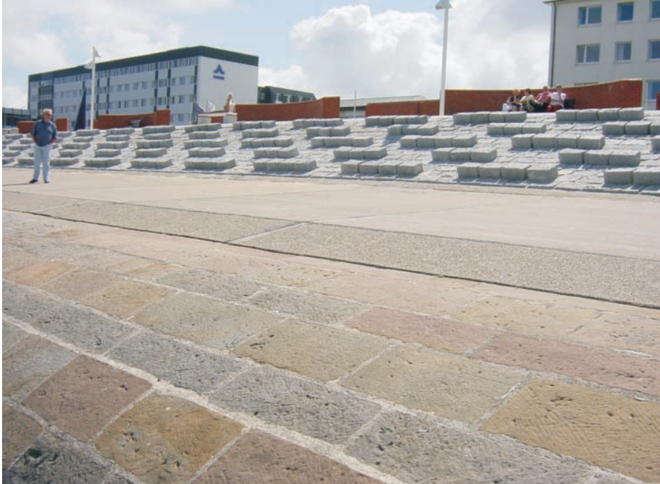
Fig. 5.19: Example for roughness elements (photo: SCHÜTTRUMPF)
