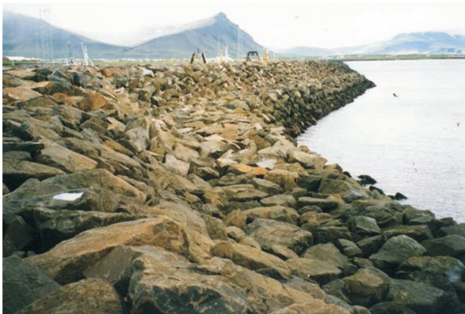
Fig. 6.7: Icelandic Berm breakwater
