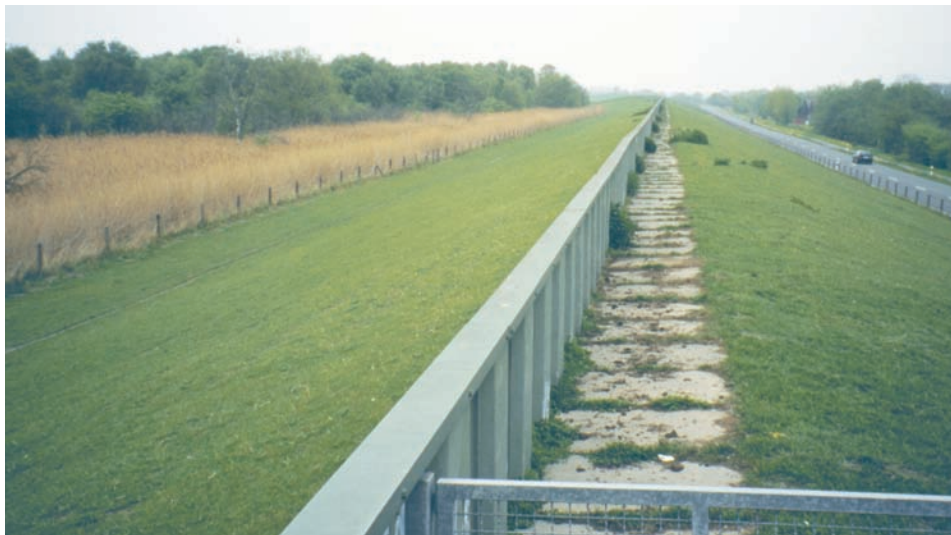
Fig. 5.30: Sea dike with vertical crest wall (photo: HOFSTEDE)
