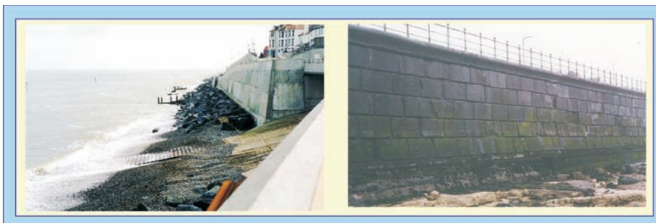
Fig. 7.2: Examples of vertical seawalls: (left) modern concrete wall and (right) older stone blockwork wall
