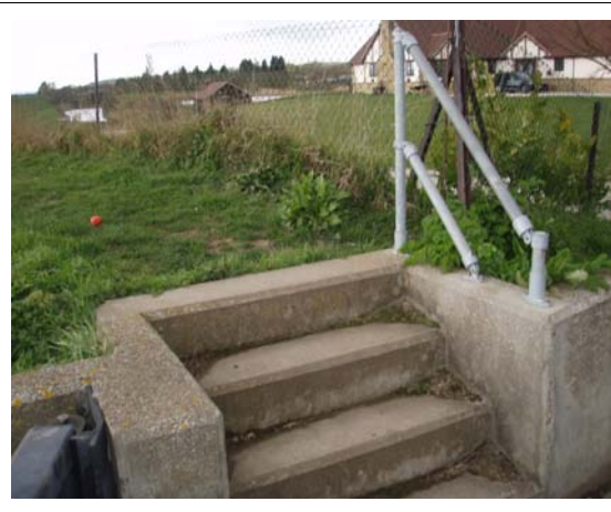
Photograph 6.15 Short handrail.
