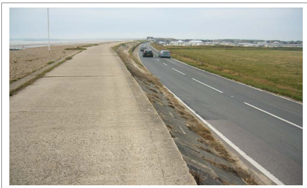
Photograph 6.2 Typical sea wall.
