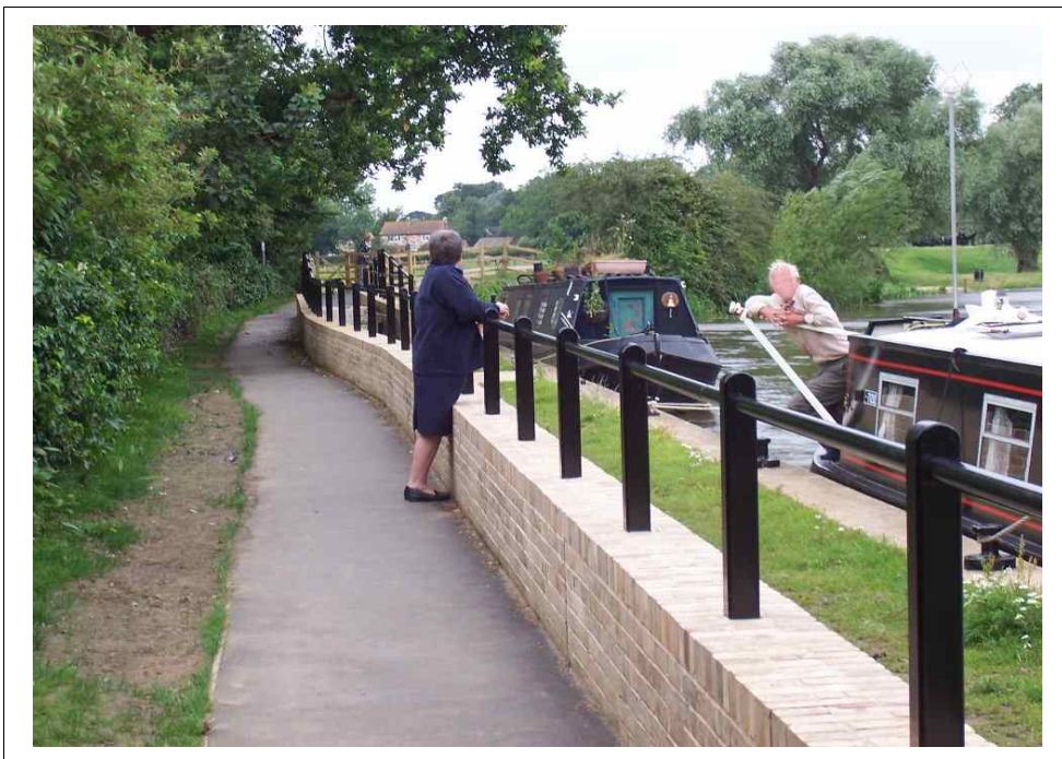
Photograph 6.3 Black coloured hand railing on top of flood wall.
