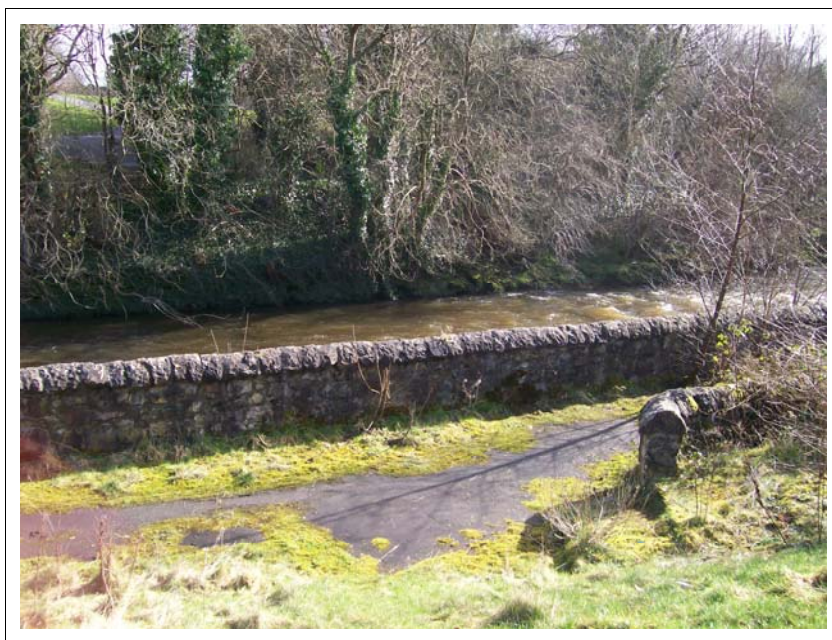
Photograph 6.29 Traditional masonry walled protection.
