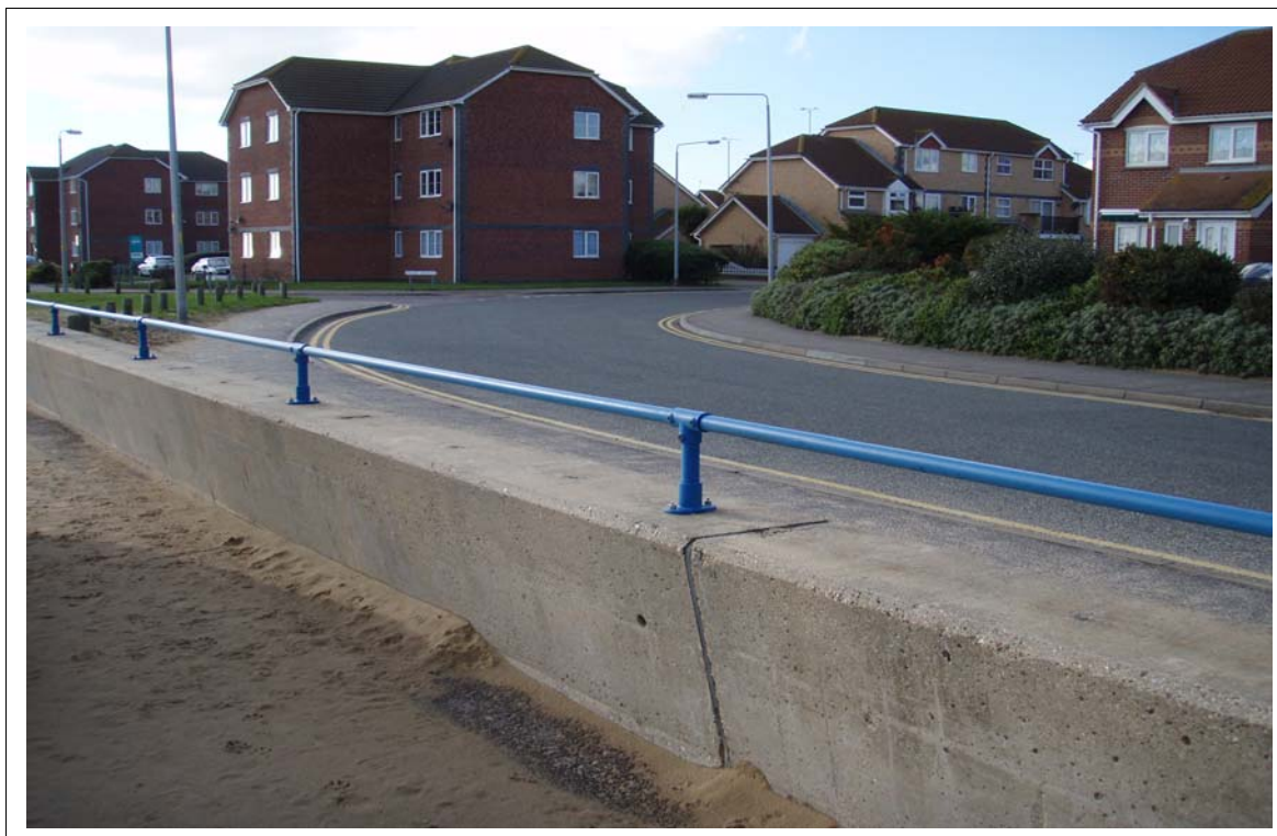
Photograph 6.5 Handrailing to flood wall.
