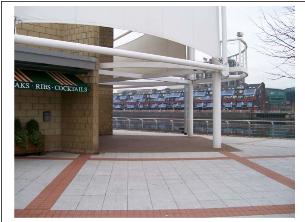
Photograph 6.33 Four rail barrier at a leisure centre.
