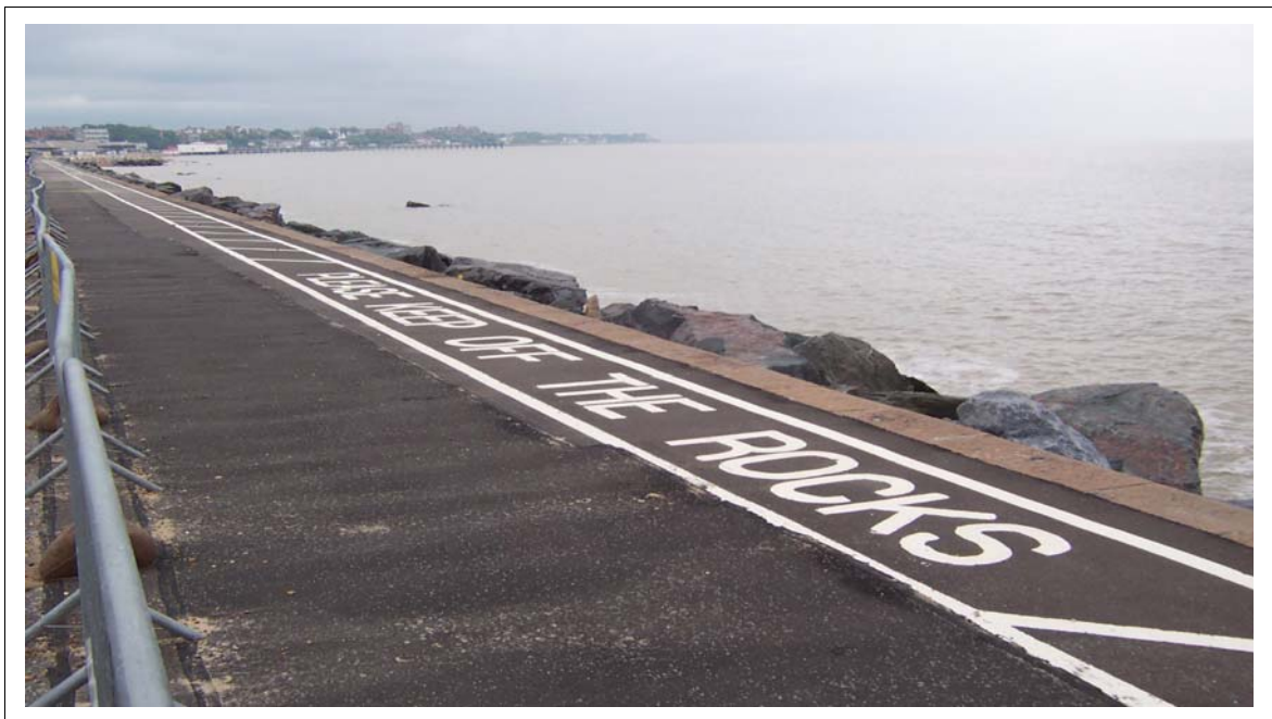
Photograph 6.28 Extensive line marking.
