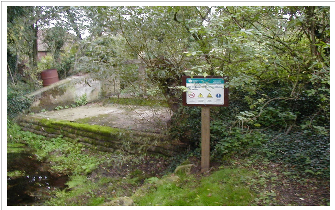
Photograph 6.4 Bypass Weir.
