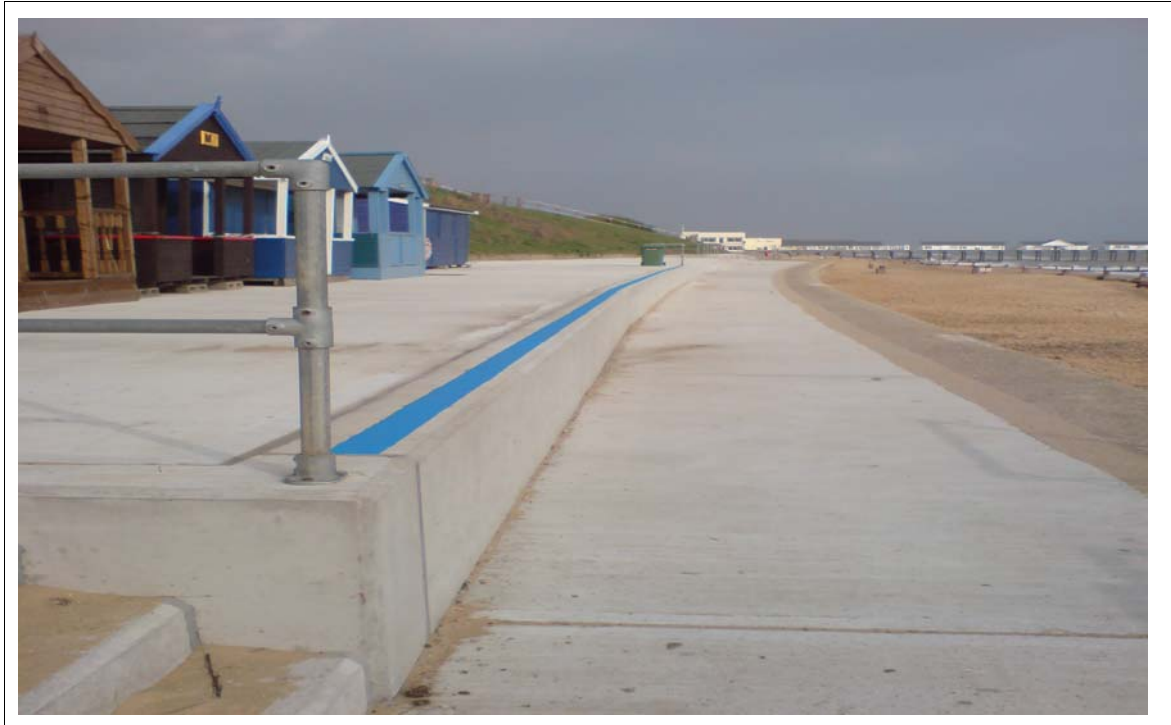
Photograph 6.26 Edge line marking.
