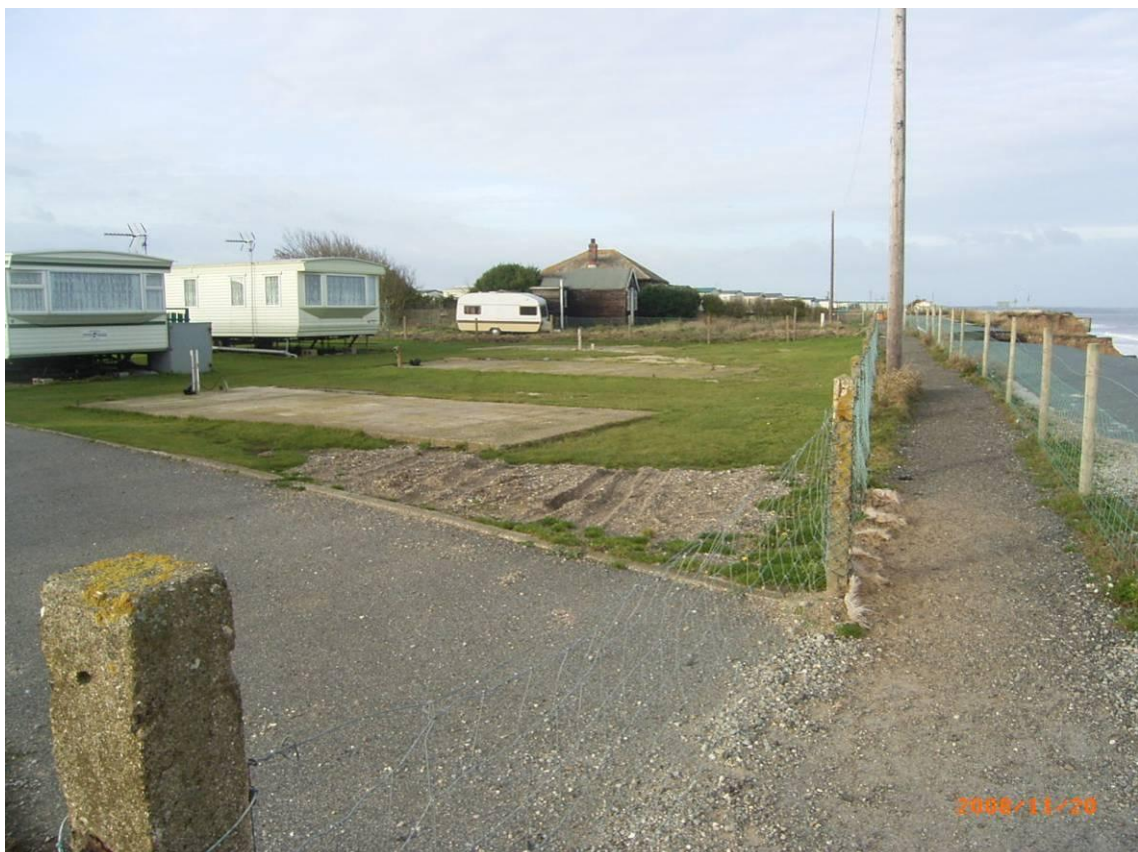
Photograph 13: Vacated pitches at a caravan park at Skipsea, now too close to the cliff edge for occupation
