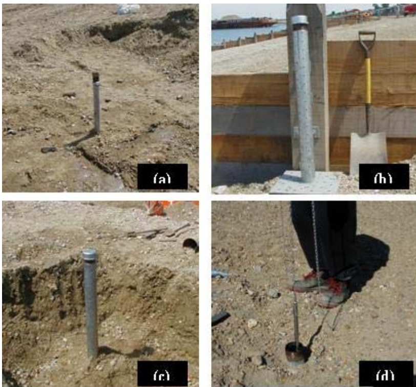
Figure 16 Components of beach water level monitoring system
