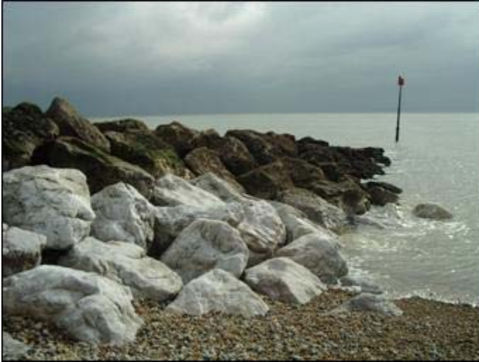
Figure 3 Photograph of a typical rock groyne along the Folkestone to Hythe frontage
