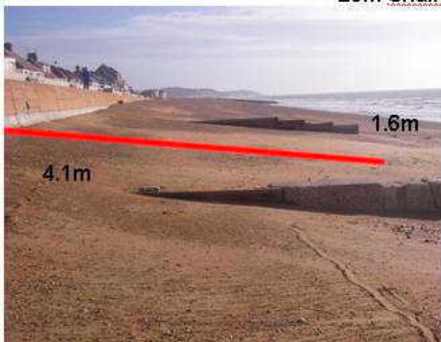
Figure 33 Showing the profile after (a) recycling and (b & c) after two consecutive storm events
