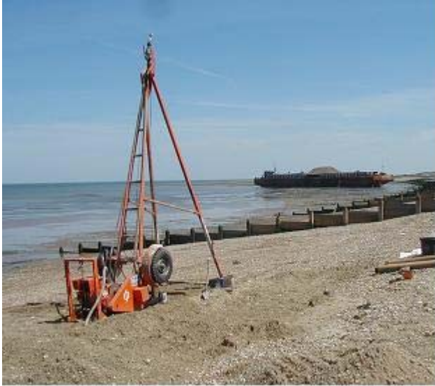
Figure 14 Borehole rig on newly-replenished beach
