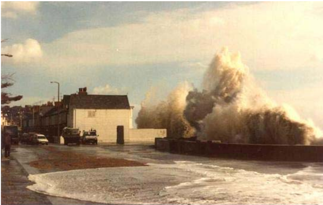
Figure 2 Photograph showing extensive coastal flooding at Sandgate – pre-coast protection scheme
