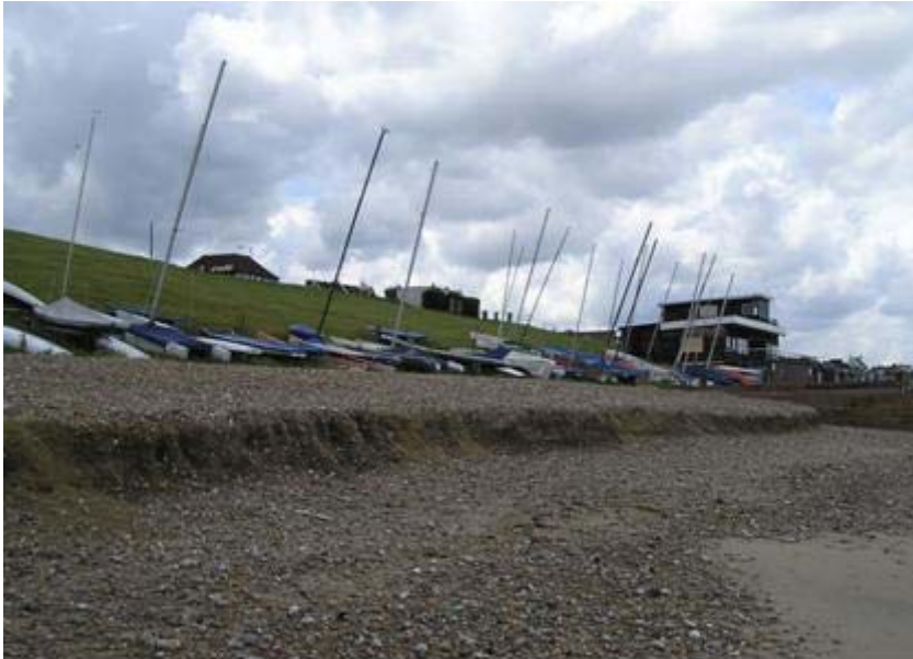
Figure 20 Cliffing in the 'fine' bay a few months after placement
