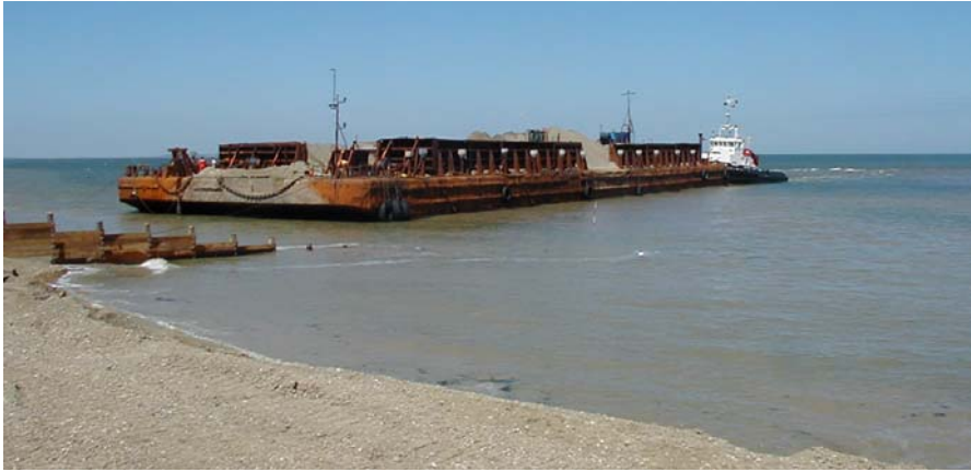
Figure 7 Dredged shingle delivered by barge
