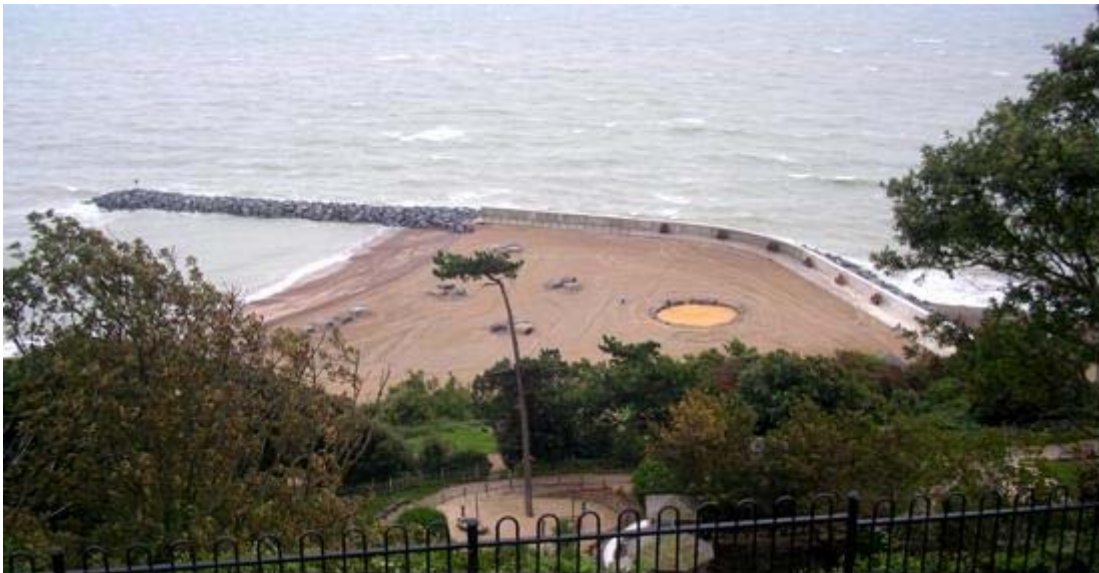
Figure 6 Photograph of the finished scheme at Folkestone
