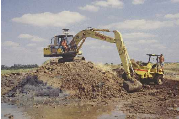
Figure 6.3 Breaching of Tollesbury Creek Realignment
