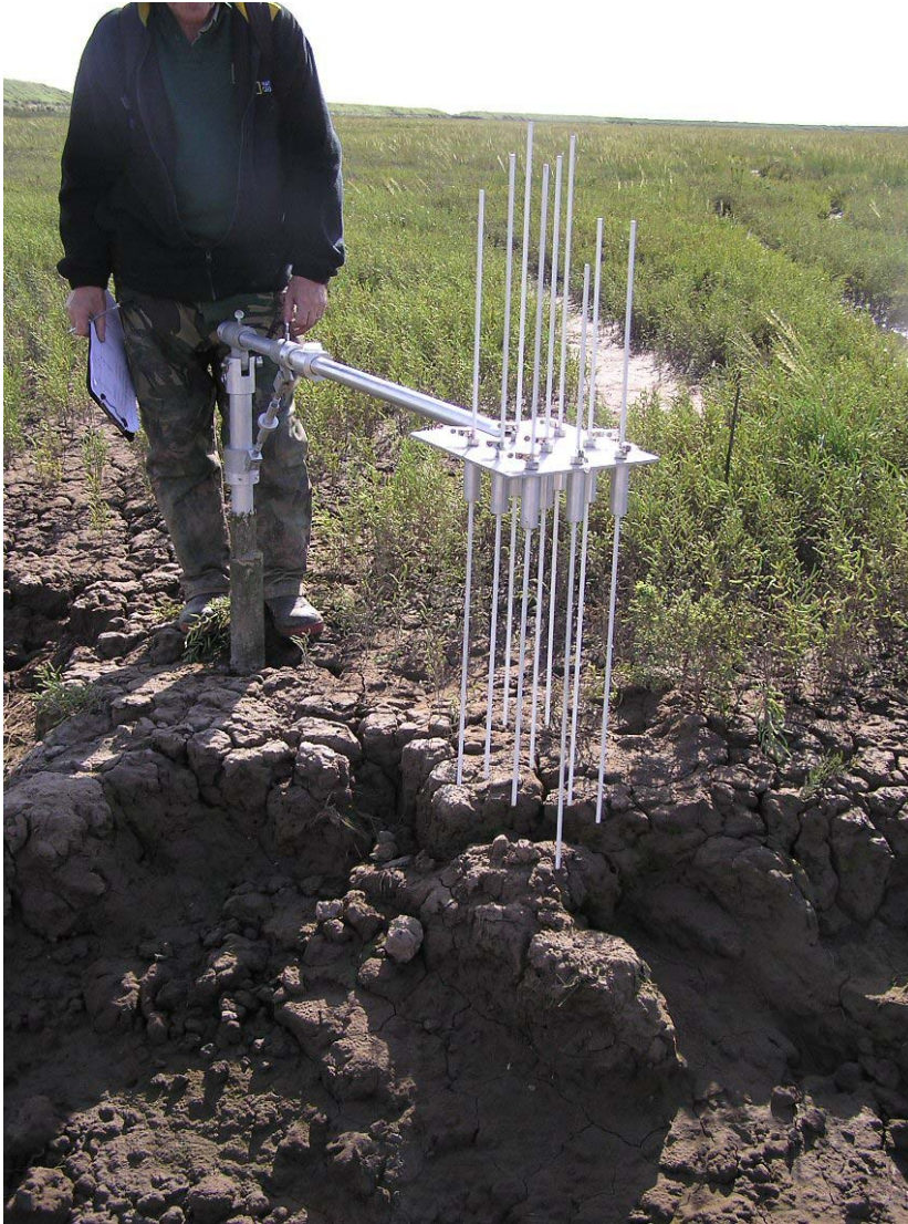
Plate 4.3. Surface collapse due to headward creek expansion at site 7, September 2006 (photograph: A Balbo). Upper creek bank cliff ca. 40 cm high. Note vegetation cover in comparison to Plate 2.
