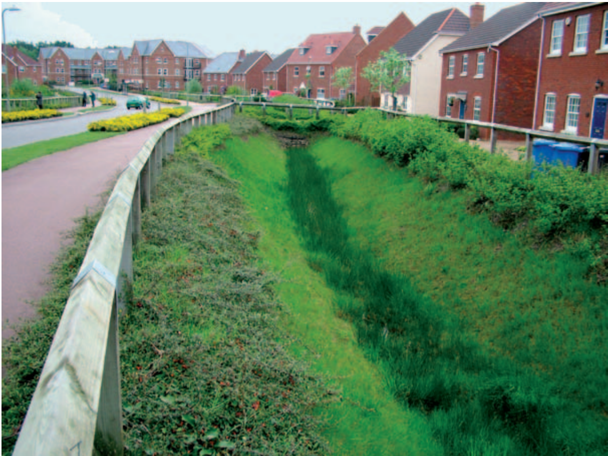
Figure 5.2 Use of SUDS in a new housing development (courtesy of HR Wallingford Ltd.)
