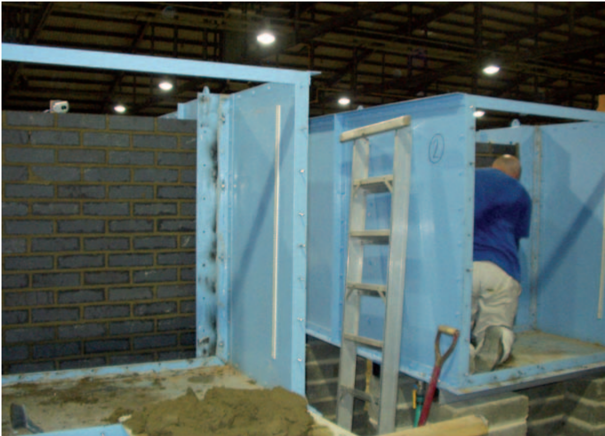
Figure 7.4 Constructing wall test panels in the laboratory test rigs
