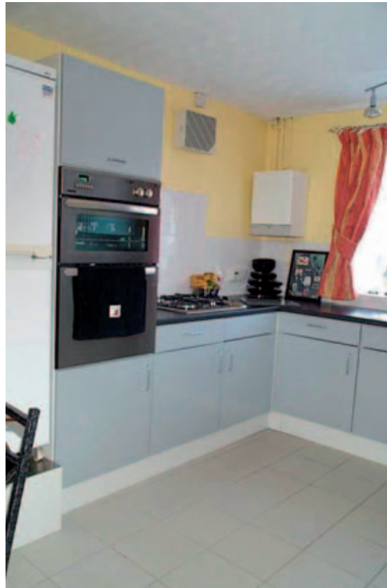
Figure 6.12 Main kitchen appliances (such as oven and fridge/freezer) placed above floor level (courtesy of Norfolk County Council and FLOWS Project)
