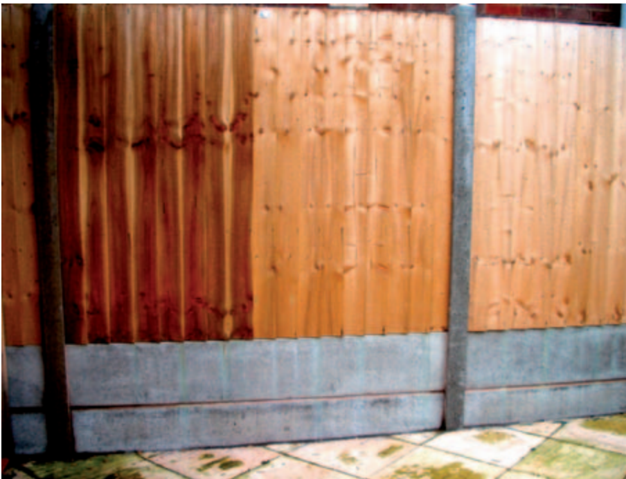
Figure 5.6 Example of protection of fence base with impermeable material (courtesy of Severn Trent Water)
