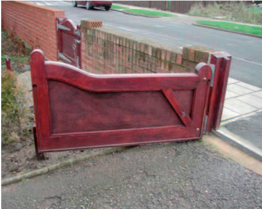
Figure 5.5 Example of sealed gate (courtesy of Severn Trent Water)
