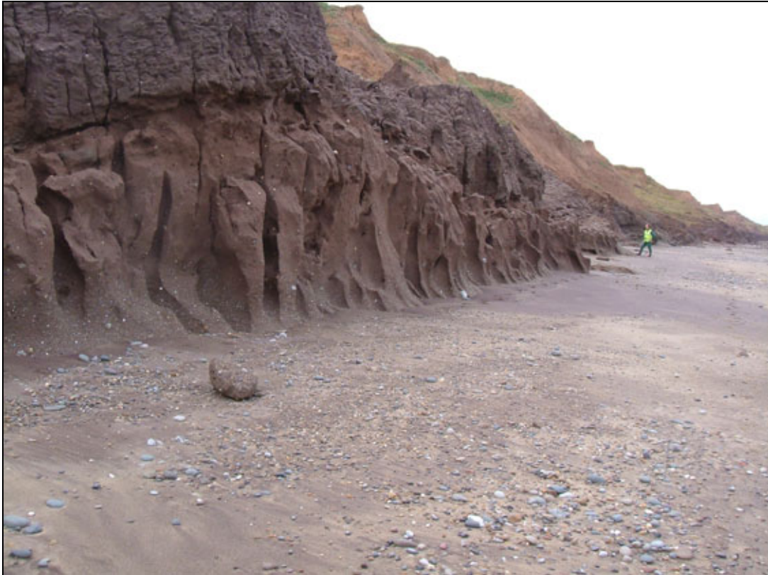
Figure 3.7. Morphology indicating direct erosion of the cliffs by waves at Easington, 26 th July 2005.
