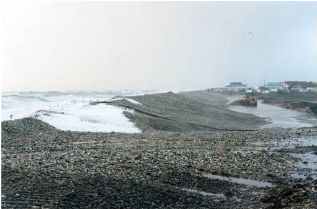
Plate 5.11 Management of the shingle ridge at Medmerry
