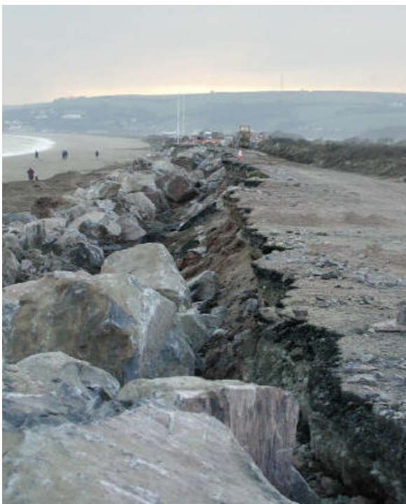
Plate 1.4 Erosion of Slapton coast road - 1999 (Peter Wagstaff) http://www.saveslaptoncoastroad.co.uk
