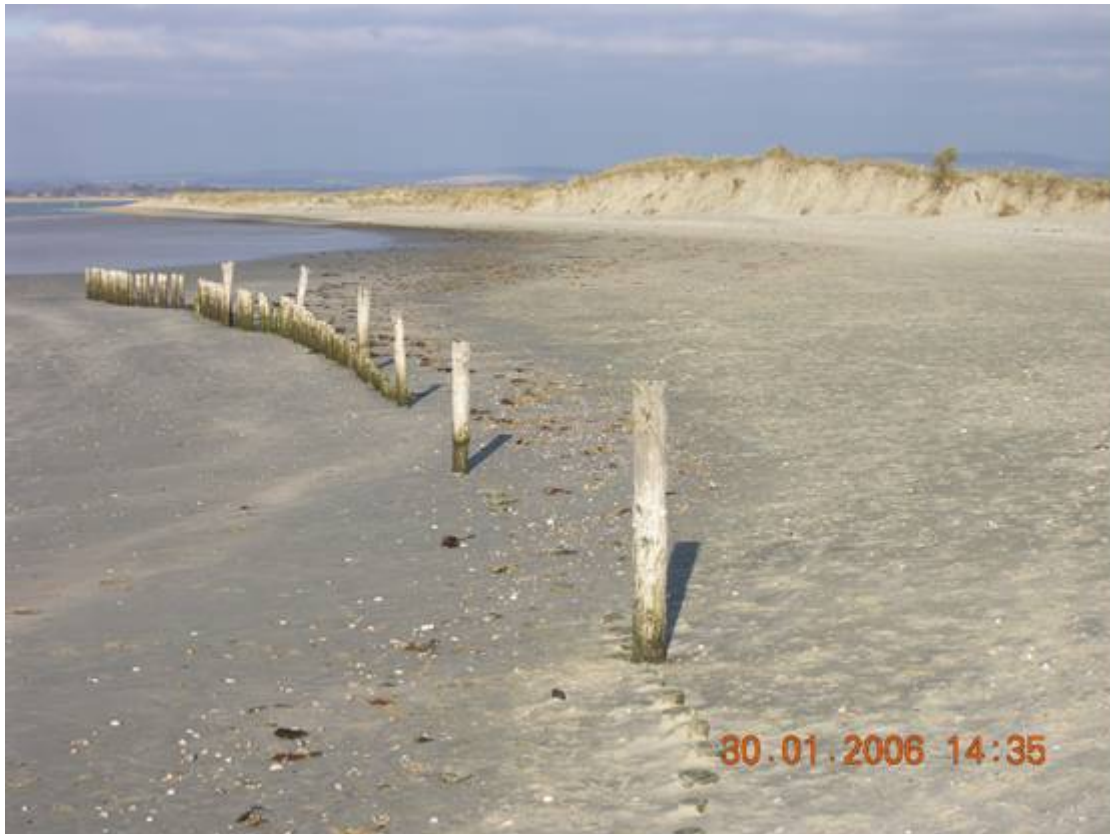
Plate 5.28 Dune recession from line of timber piles, at neck of spit
