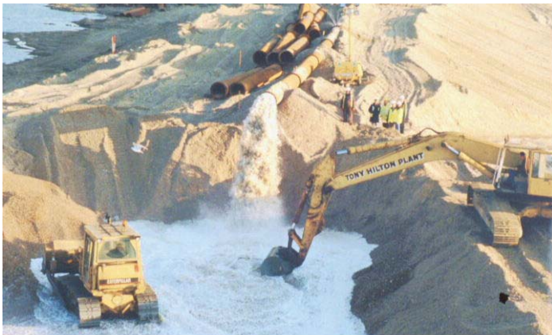
Plate 6.5 Placement of beach recharge materials at Hurst Spit (1996, David Bowie Photography)
