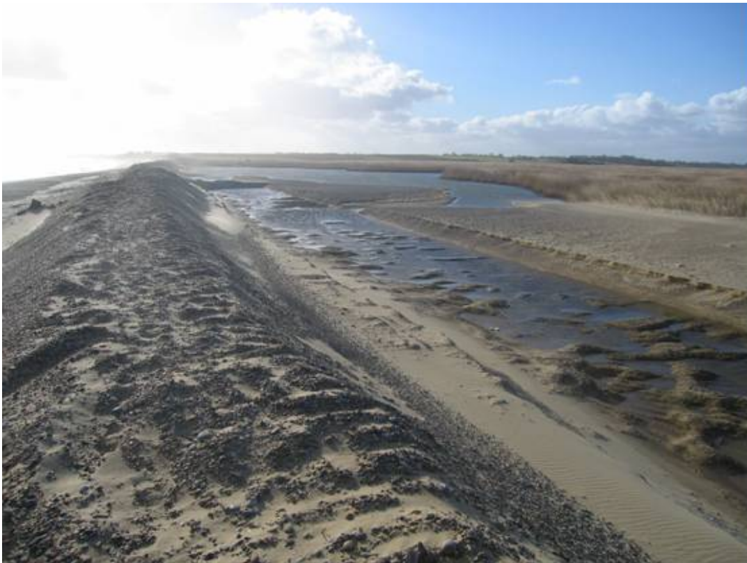
Plate 5.34 Sand blow removing fines from the crest and infilling saline lagoon (Motyka)
