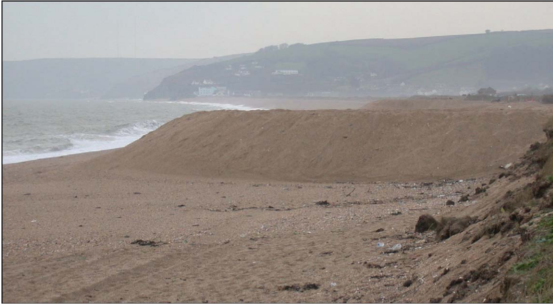
Plate 5.19 Shingle bastion placement at Slapton Sands, 2002 (Ian Stevenson)
