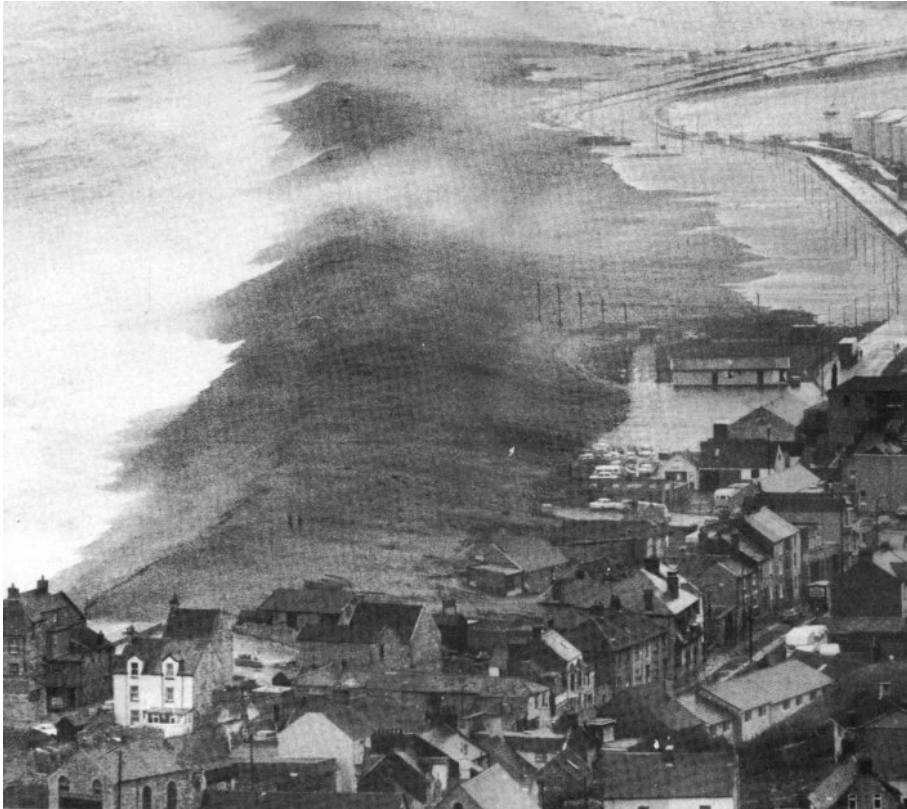
Plate 5.15 Overwashing at Chiswell during 1979 storm
