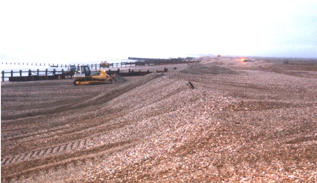
Plate 6.2 Post-storm reprofiling of Medmerry barrier, November 1998 (Pett, Environment Agency)
