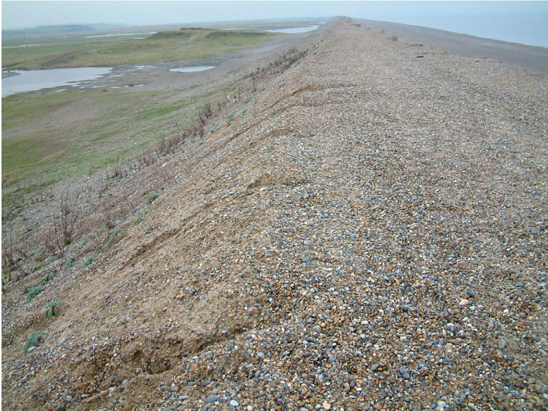
Plate 6.4 Lee slope runnels formed by overtopping waves at Cley-Salthouse (Bradbury)
