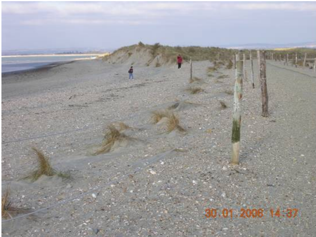
Plate 5.29 Sand nourishment berm at neck of East Head
