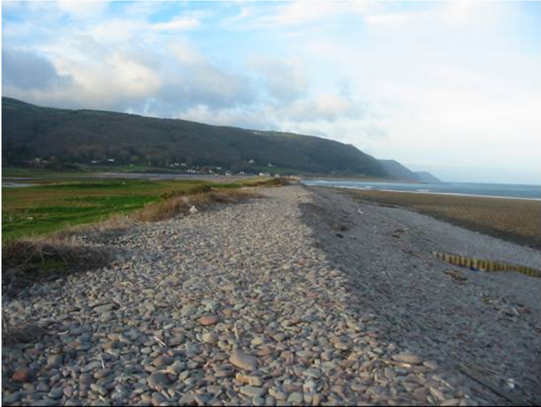
Plate 5.1 Looking west towards the breach at Porlock, January 2005 (Cope)
