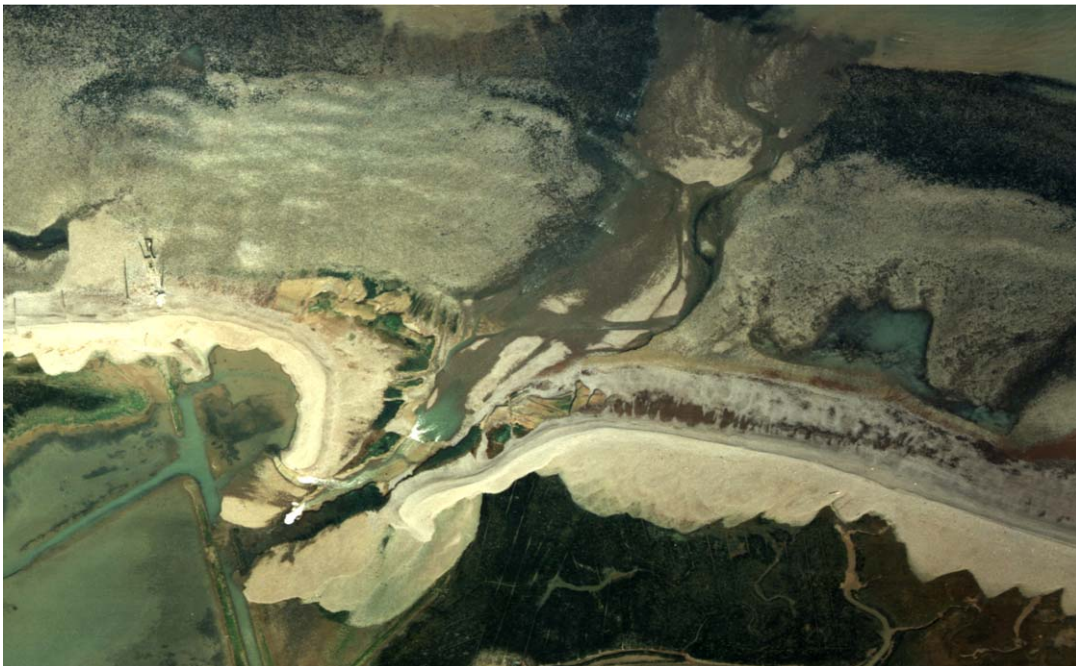
Plate 2.4 Example of Porlock barrier, Somerset that breached 26 th October 1996 (Environment Agency, 1999)
