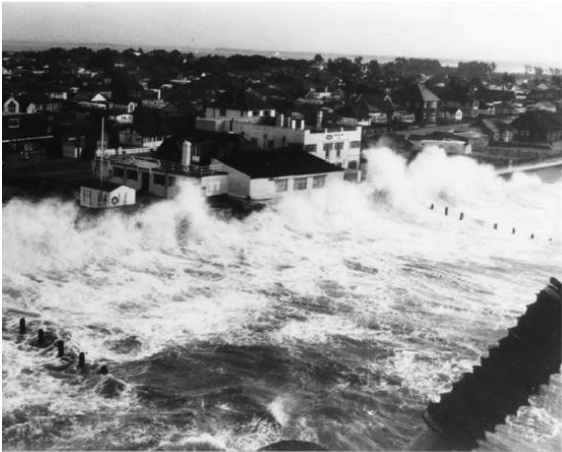
Plate 5.32 Wave overtopping at Eastoke in the late 1970s
