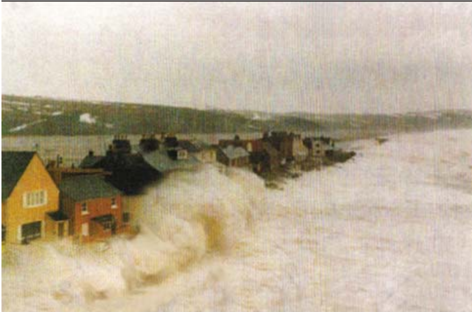
Plate 5.18 Over-topping at Torcross during the 1979 storm
