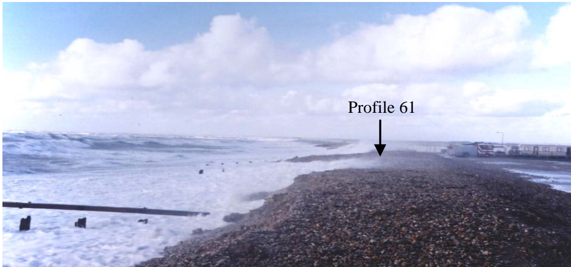
Plate 2.2 Overtopping of the Medmerry barrier, West Sussex, looking NW. 1 st February 2002 (Cope, 2004)
