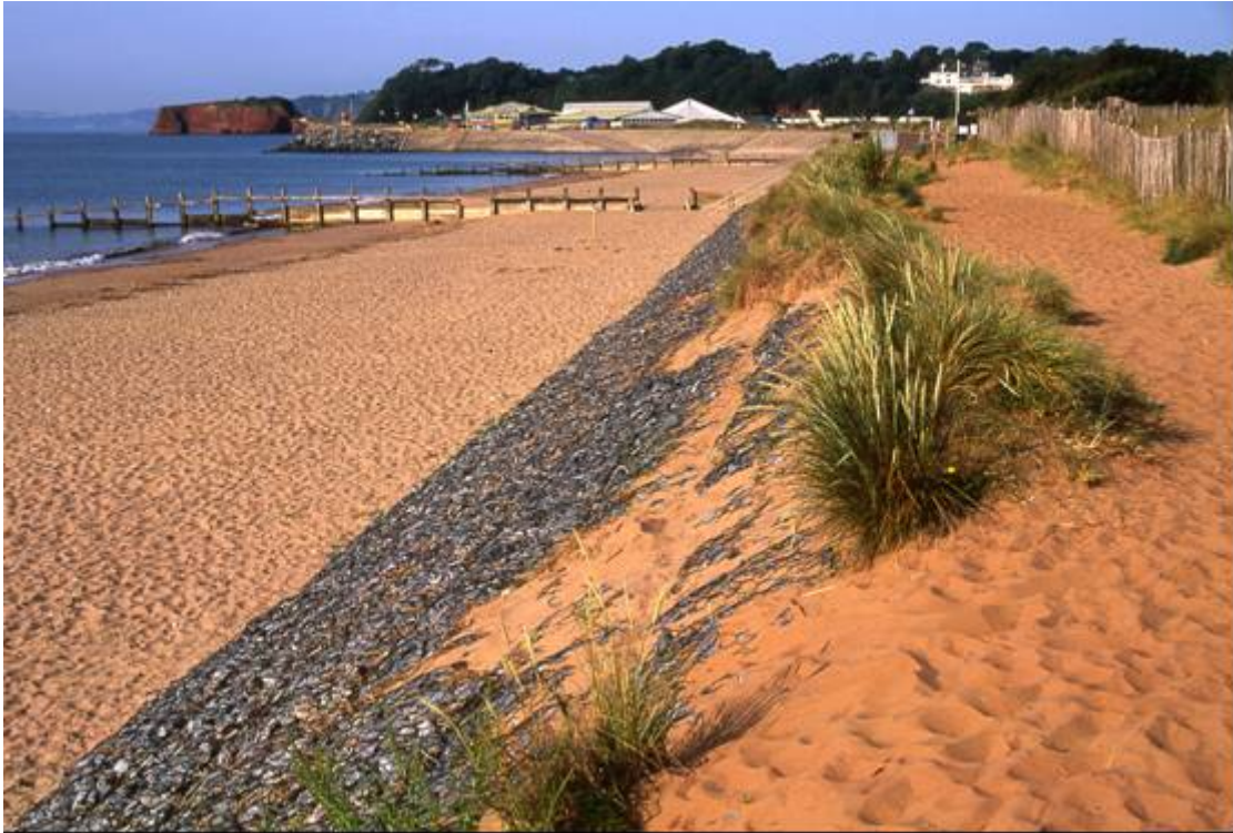
Plate 5.40 Old gabion baskets at western end of Dawlish Warren – 2005
