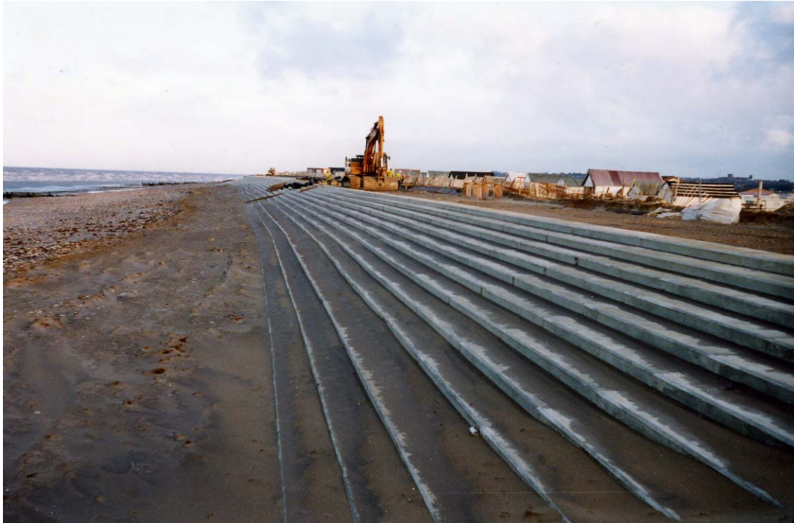
Plate 24 Stepped sloping seawall, Heacham, Norfolk, 2003
