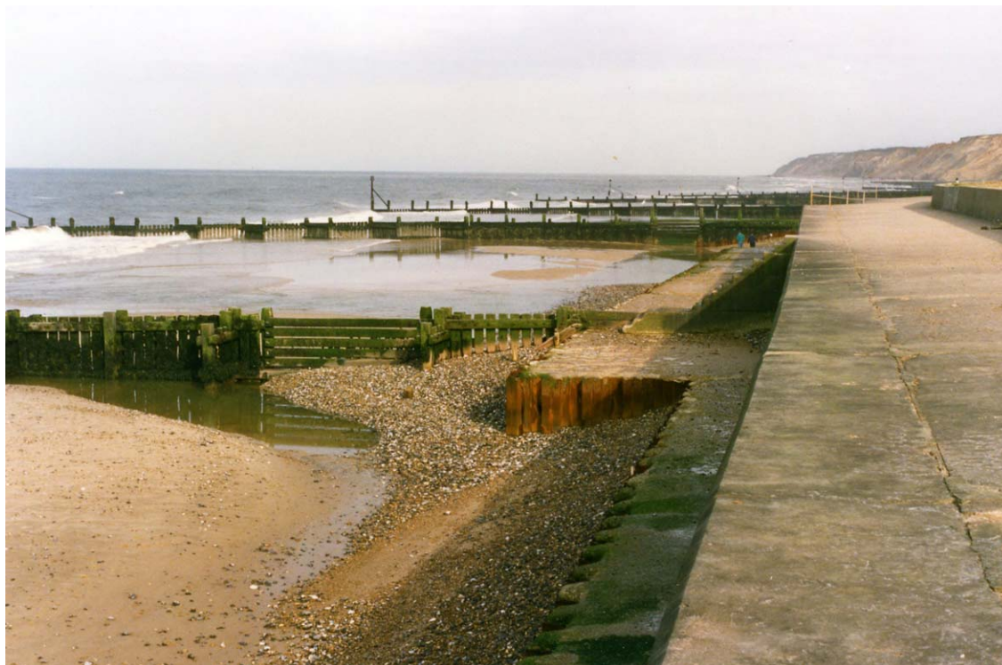
Plate 20 Vertical faced apron, Overstrand, Norfolk, 1991
