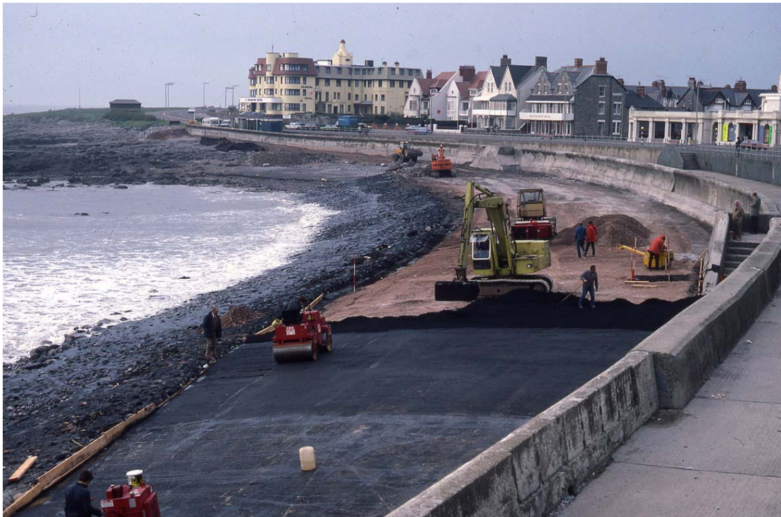
Plate 22 Asphaltic revetment under construction, Porthcawl, Glamorgan, 1984
