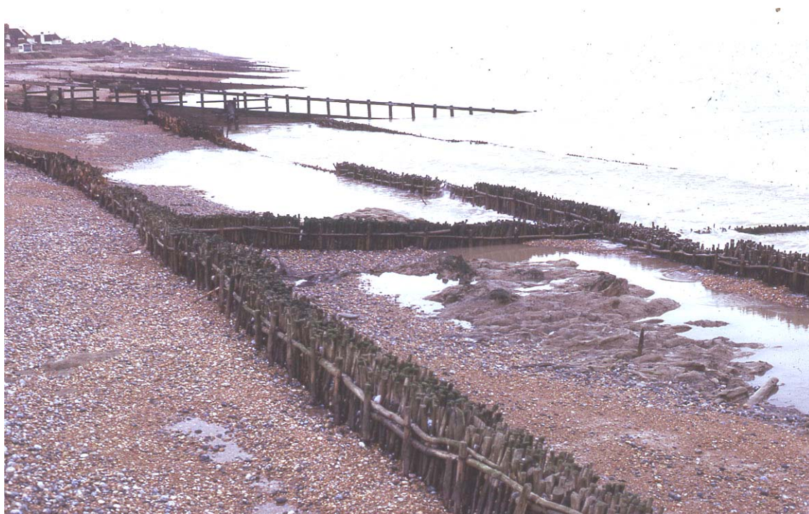
Plate 1 Fagotting at Cooden shingle beach, Pevensy Bay, 1983
