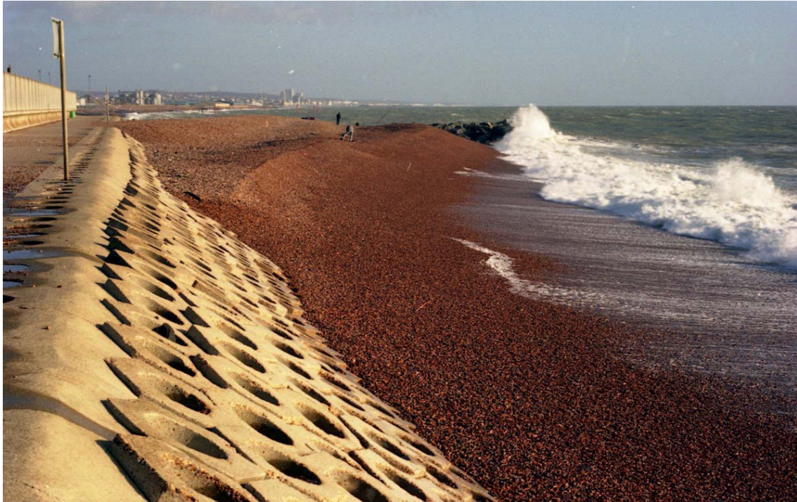
Plate 27 Energy dissipating concrete block wall, Shoreham, West Sussex, 2005
