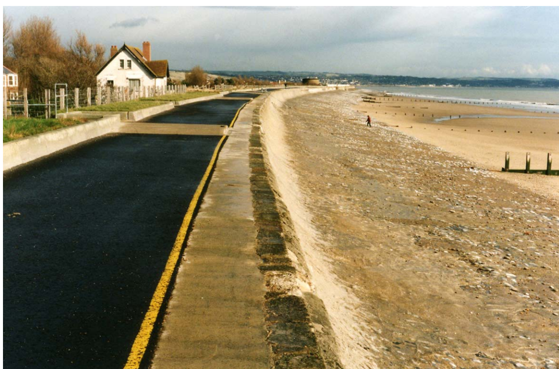
Plate 21 Sloping apron to seawall, Dymchurch, Kent,
