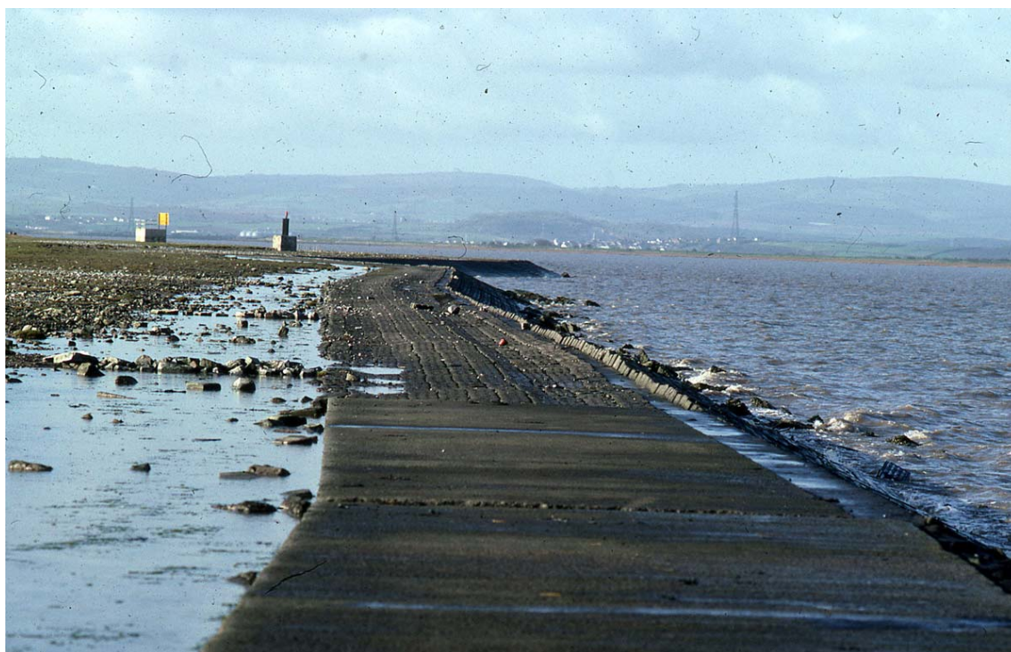
Plate 5 Concrete mattress revetment, West Huntspill, Somerset, 1993
