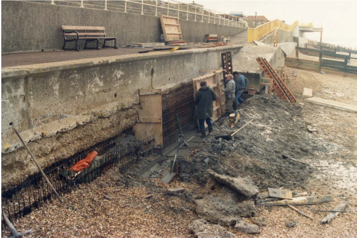
Plate 19 Extension of seawall footings, Lee on Solent, Hampshire
