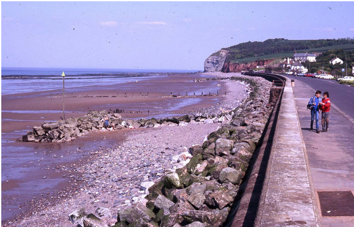
Plate 6 Rock fillet and groynes, Blue Anchor Bay, Somerset, 1988
