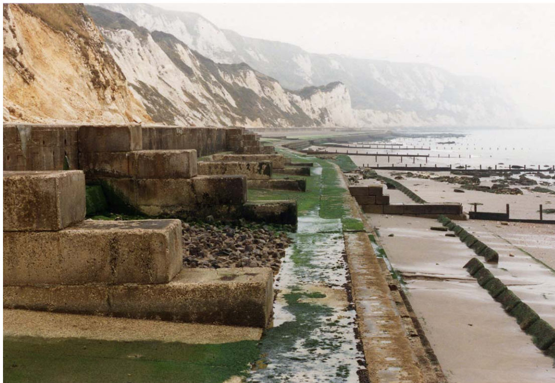
Plate 12 Concrete sill, East Wear Bay, Folkestone, 1986
