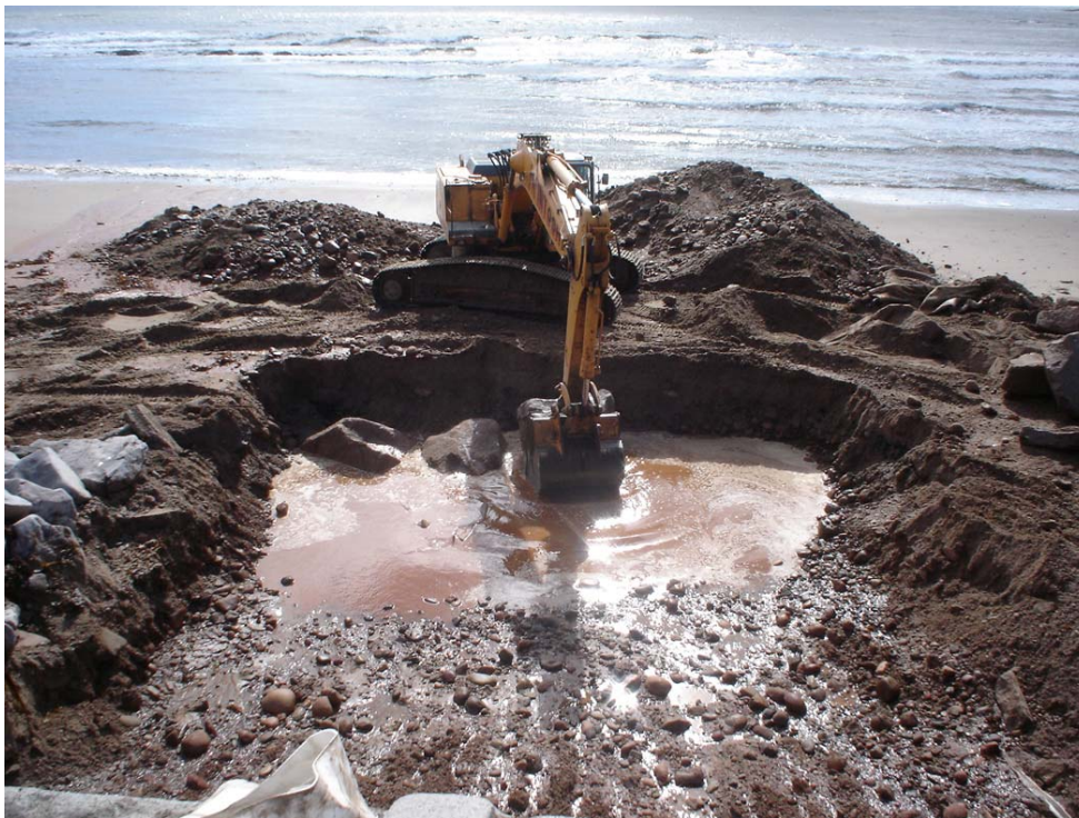
Plate 8 Installing sloping rock toe, Stonehaven, Aberdeenshire, 2004
