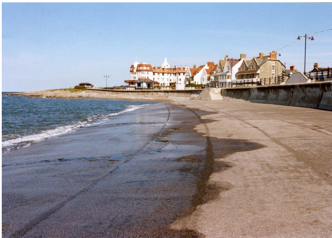
Plate 23 Asphaltic apron at high tide, Porthcawl, Glamorgan, 1995
