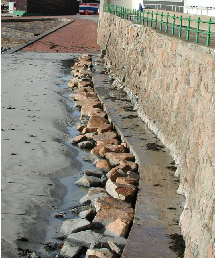
Plate 7 Rock infill of scour trough, Le Dicq, Jersey, 2005
