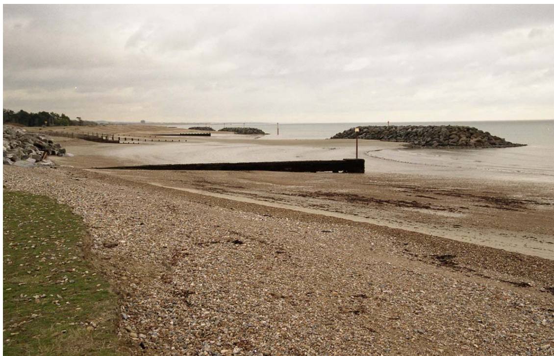
Plate 11 Detached breakwaters, Elmer, West Sussex, 2005
