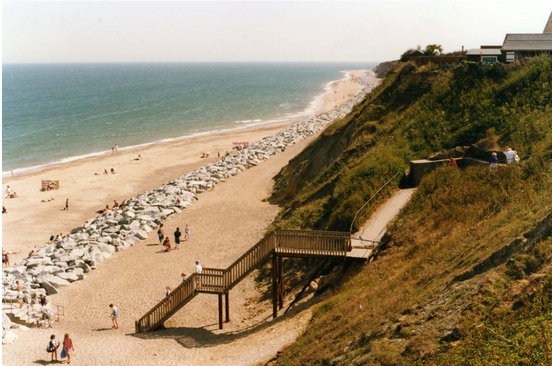
Plate 13 Rock sill, California, Norfolk
