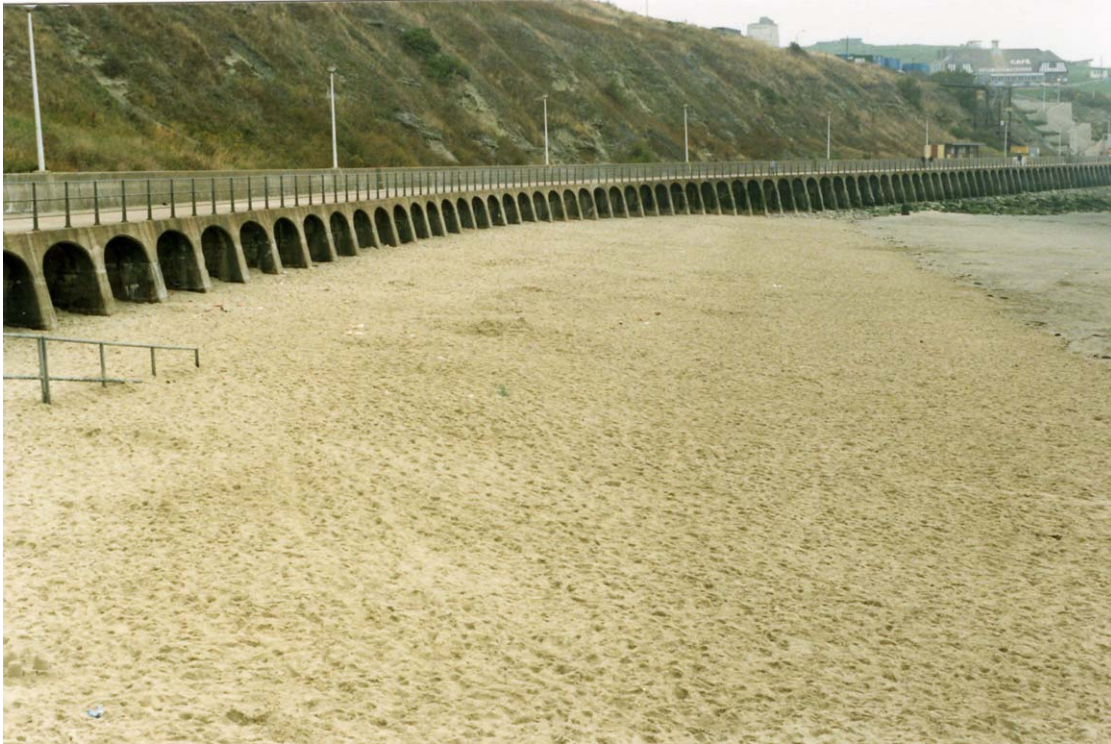
Plate 25 Cellular seawall, Folkestone, Kent, 1986
