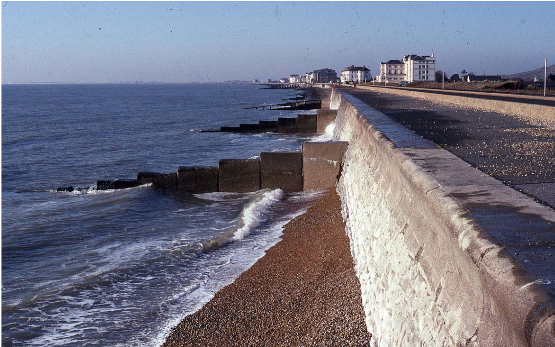
Plate 16 Old groyne field, Sandgate, Kent, 1986
