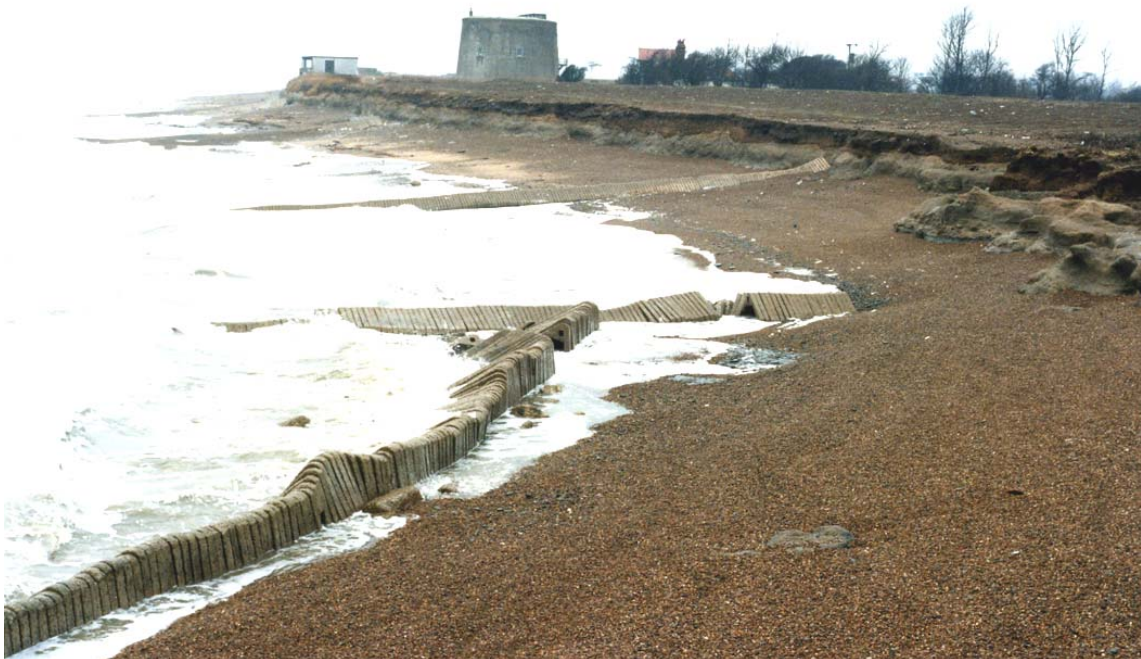
Plate 14 Concrete sill and groynes, Bawdsey, Suffolk, 1996
