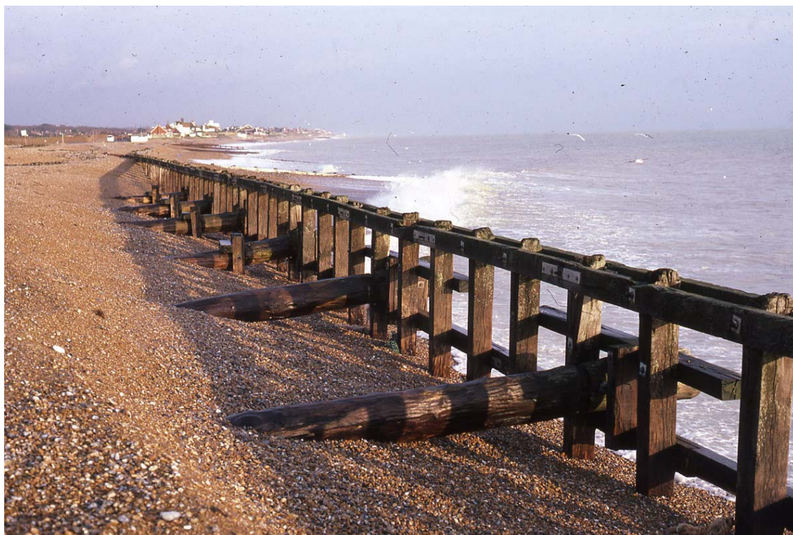
Plate 3 Wave breaker at Cooden Beach, Pevensey Bay, 1986
