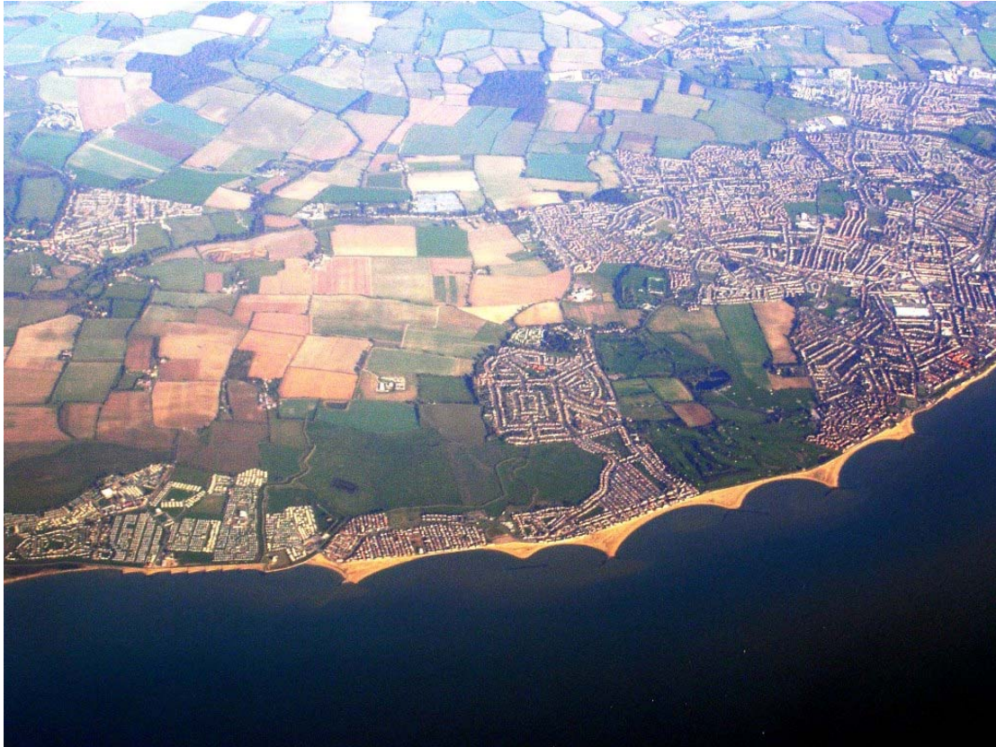
Plate 17 Variations in beach width caused by rock groynes at Jaywick
