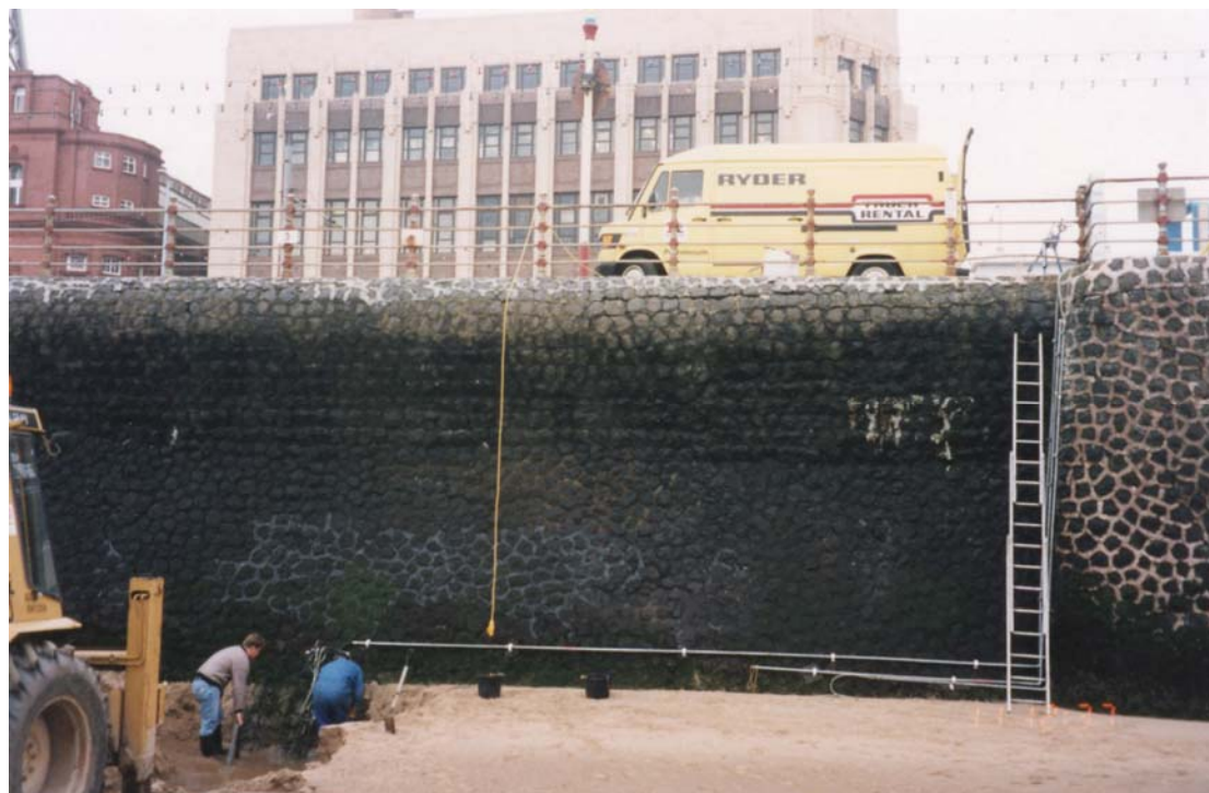
Plate 2 Installation of three scour monitors at Blackpool
