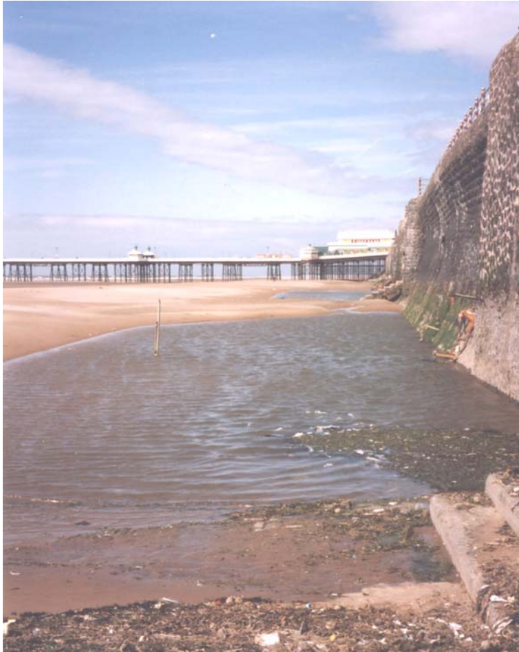
Plate 7 Three scour monitors in front of seawall, looking north
