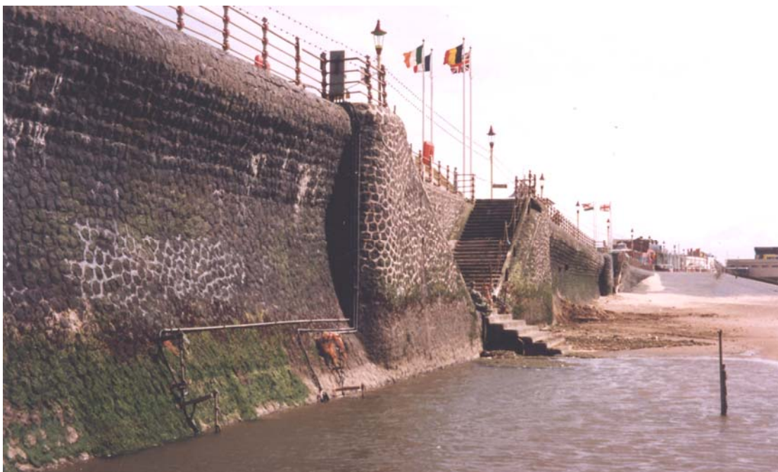
Plate 8 Three scour monitors in front of seawall, looking south
