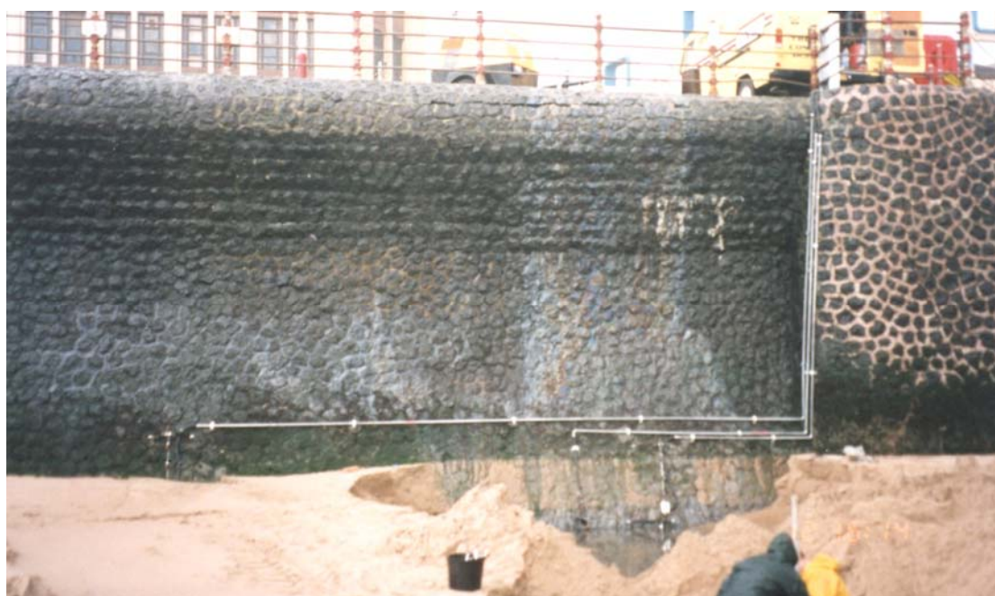
Plate 1 Installation of three scour monitors at Blackpool
