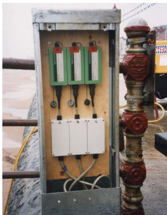
Plate 3 Scour monitor data collection box on Blackpool promenade
