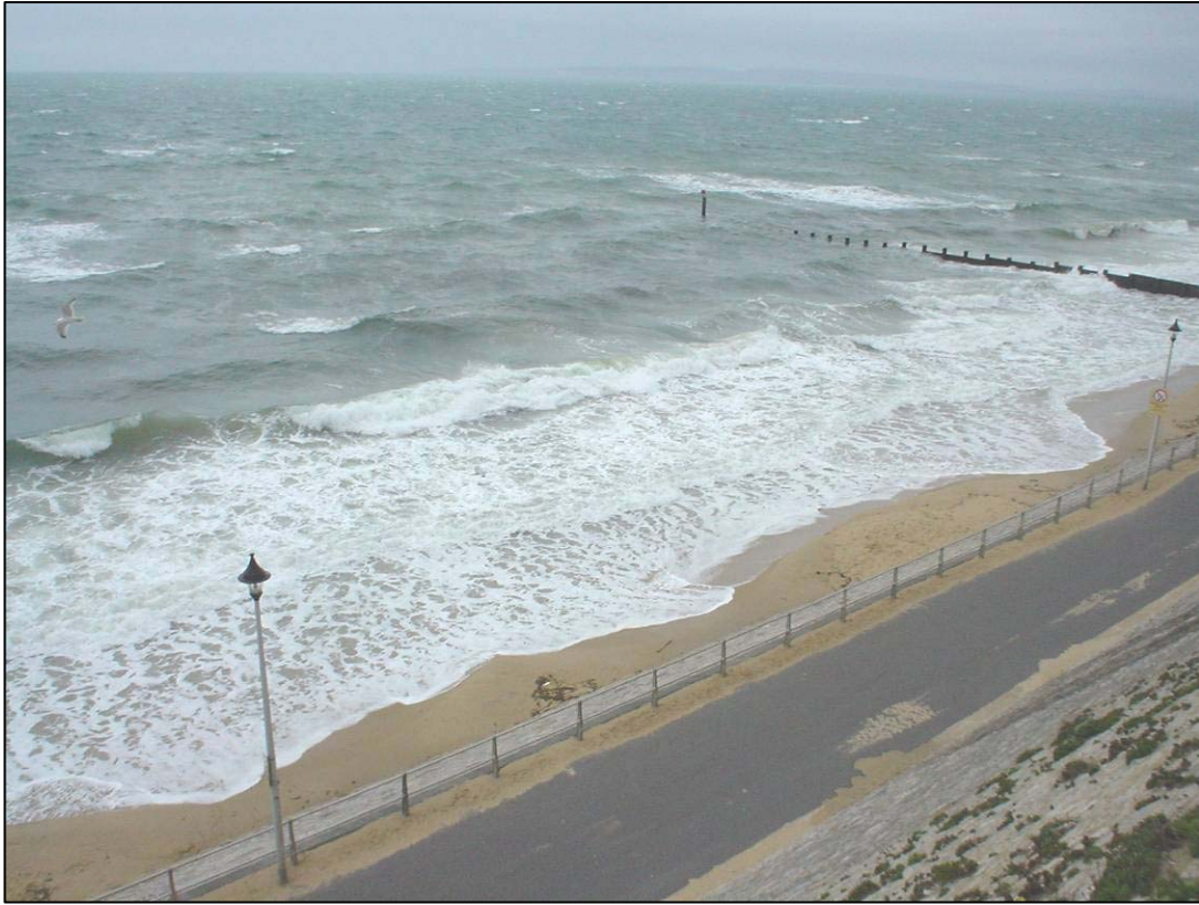
Plate 19 Looking west towards groyne G32 on 28 April 2005. Note sand on promenade.
