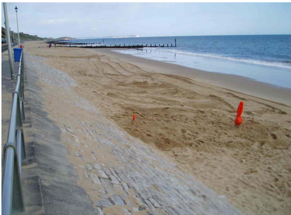
Plate 24 Scour monitors as initially deployed on 9 May 2005.
