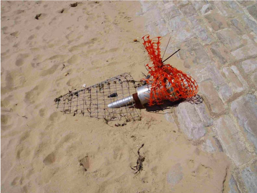
Plate 28 Upper scour monitor prior to recovery on 7 June 2005.
