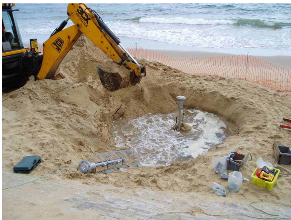
Plate 23 Backfilling of hole after placement of 2 scour monitors on 9 May 2005.
