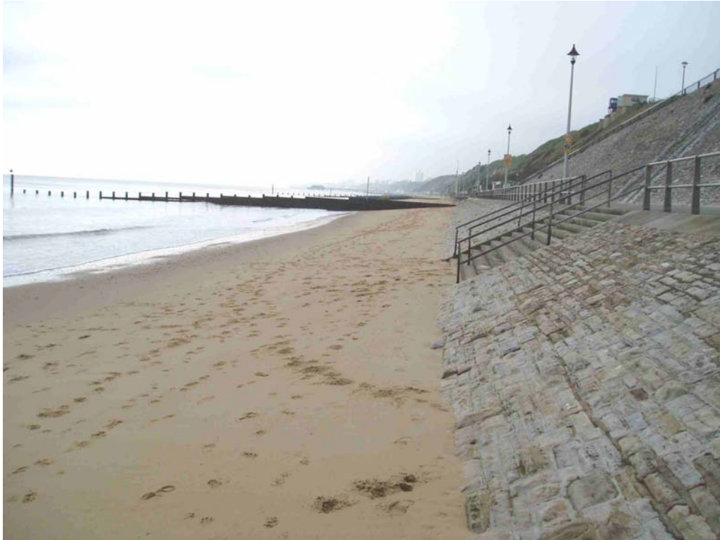
Plate 10 Looking west from profile 5f00409 (21 December 2004). Note beach extends to bottom of hand rail.
