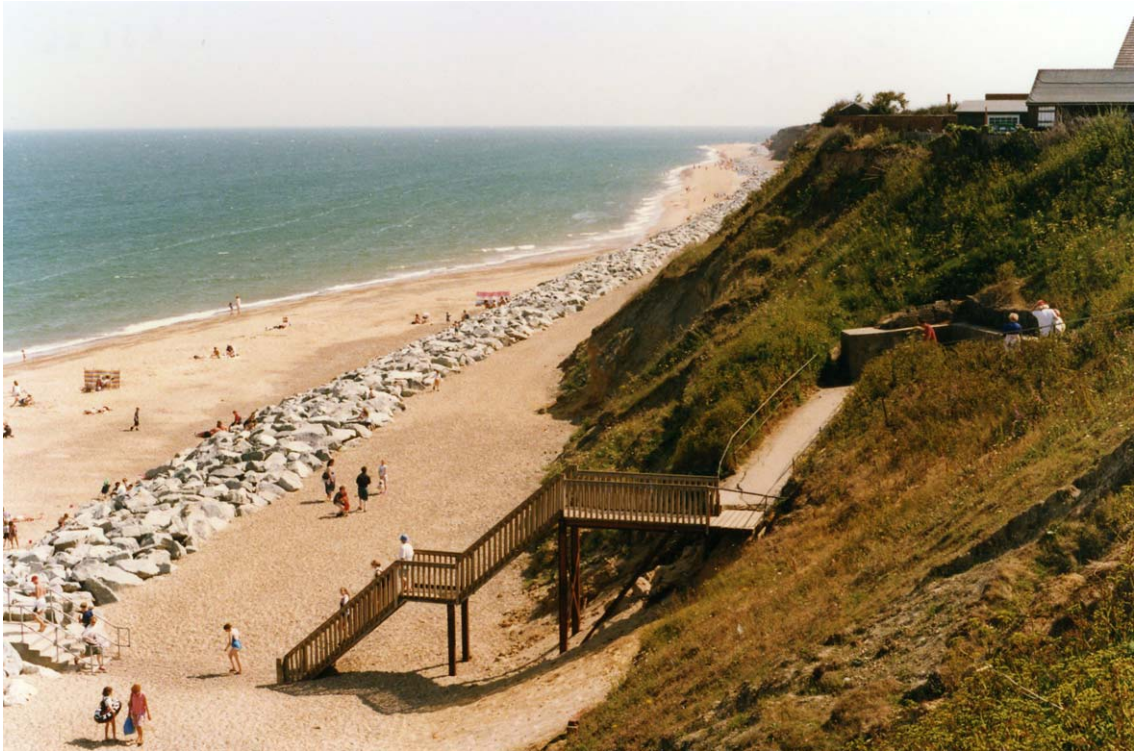
Figure 5.3 Rock sill, California, Norfolk
