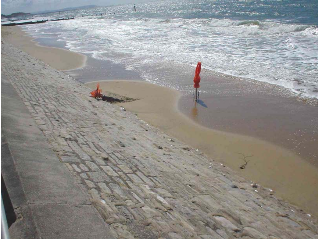
Figure 3.1 Deployment of Tell-Tail scour monitors at Southbourne
