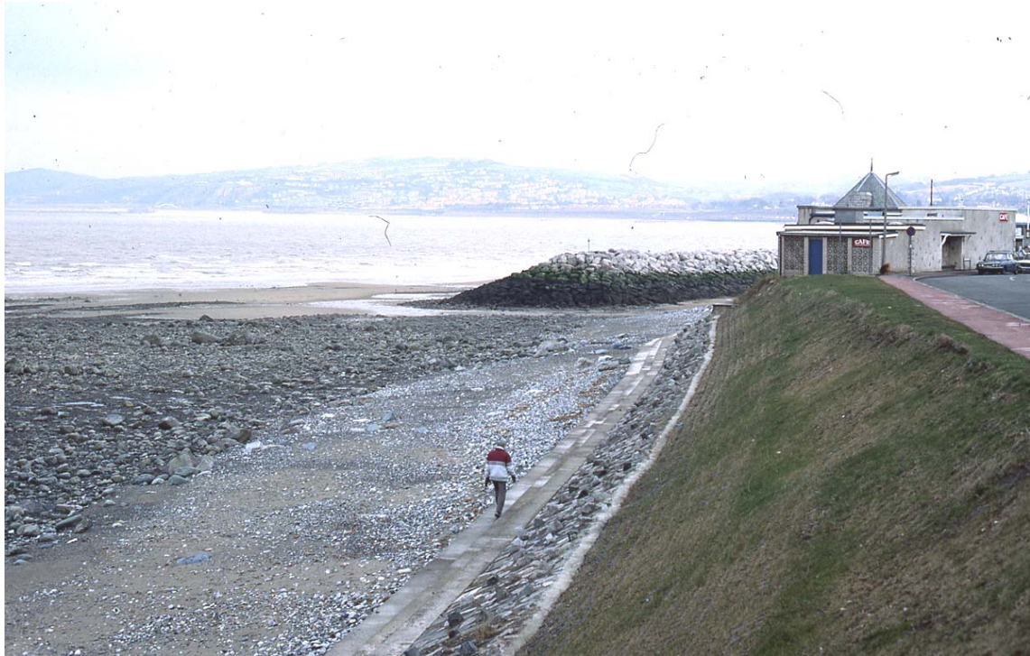
Figure 5.2 Detached breakwater, Rhos-on-Sea, Clwyd, 1986
