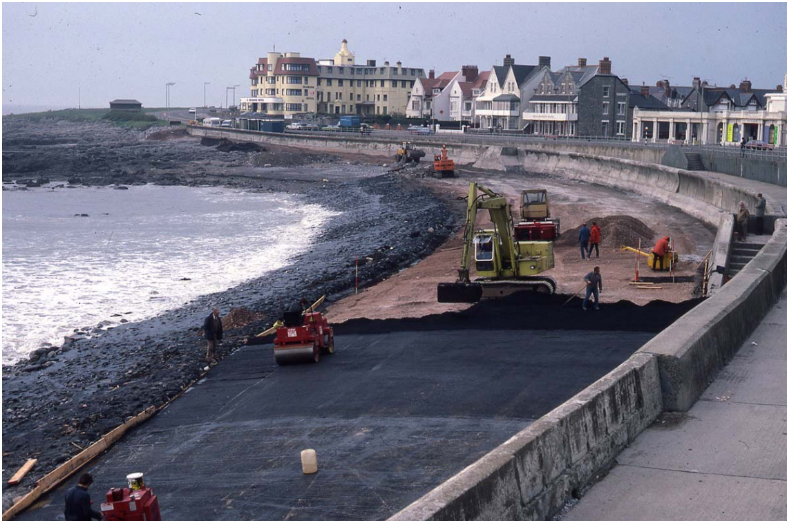
Figure 5.5 Asphaltic revetment under construction, Porthcawl, Glamorgan, 1984
