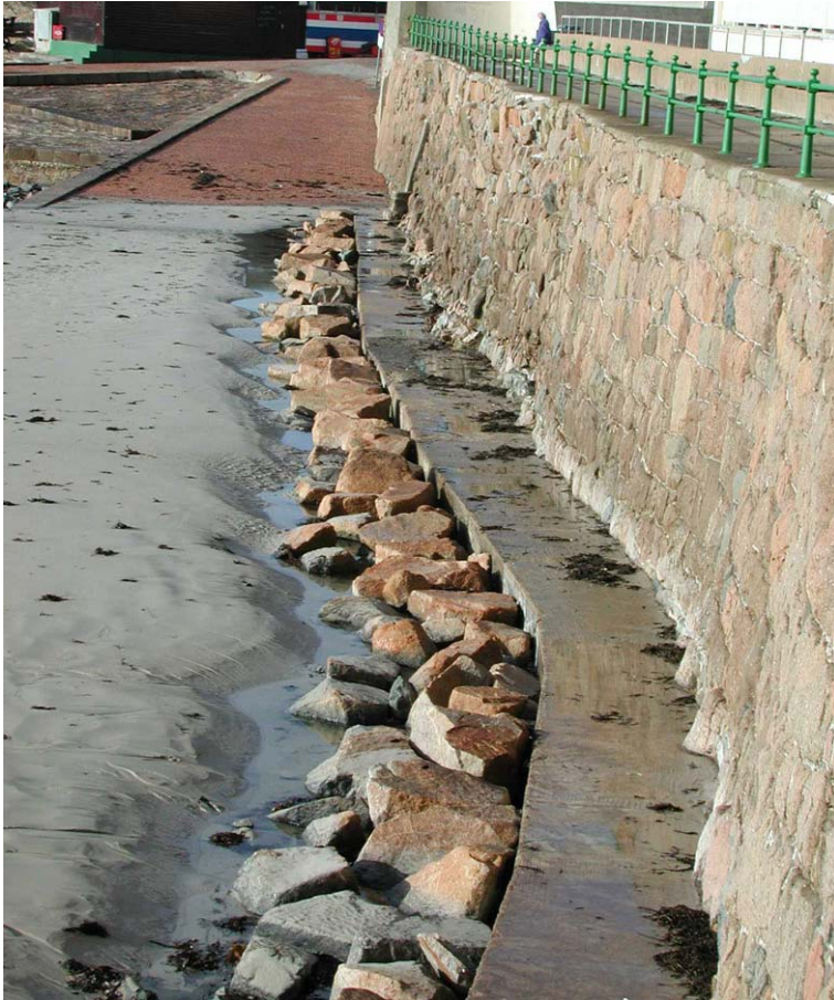
Figure 5.1 Rock infill of scour trough, Le Dicq, Jersey, 2005
