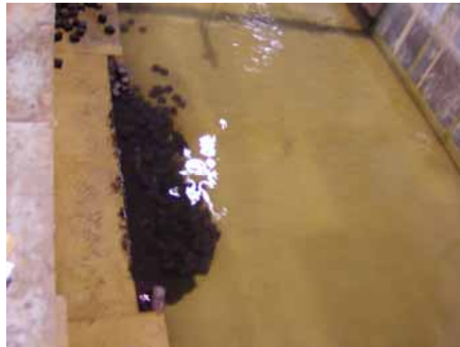
Figure A6.5 Failure of the bank (nominal depth 0.2m)
