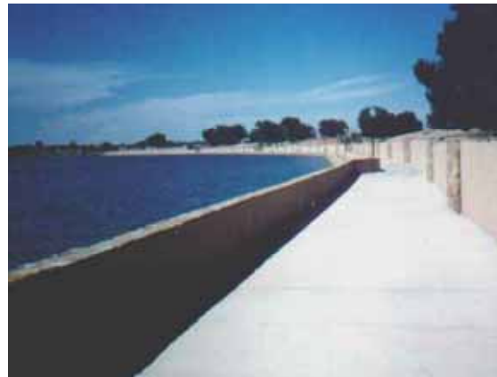
Figure 5.26 Bank stabilisation of the Pecos River in New Mexico using tyre bales (courtesy Encore Systems)
