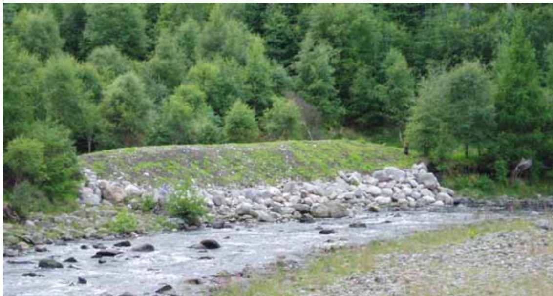
Figure 5.34 The finished river embankment
