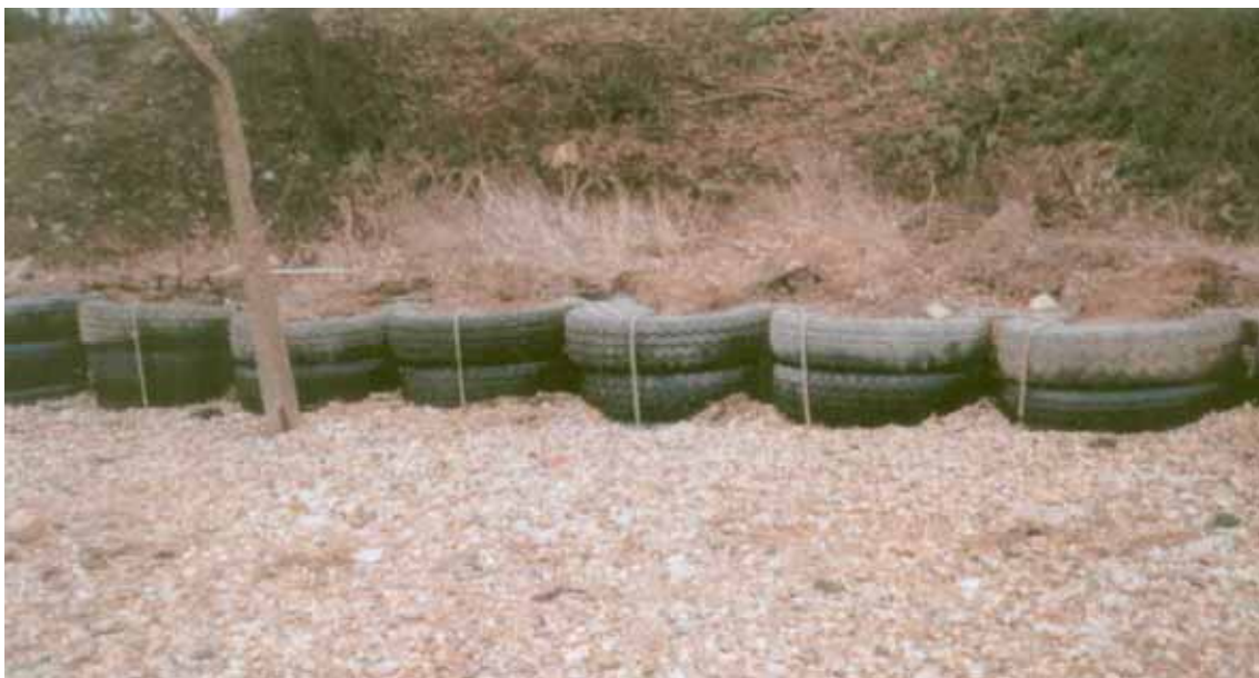
Figure 5.8 The same defence after 4 years (courtesy of Sorrell Flood Protection)
