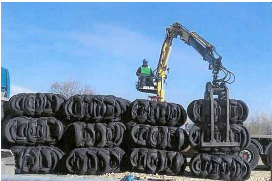
Figure 4.5 Offloading tyre bales from a delivery vehicle at a project site. (courtesy Environment Agency)
