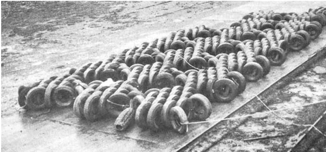
Figure 5.17 Floating tyre breakwater at Port Edgar
