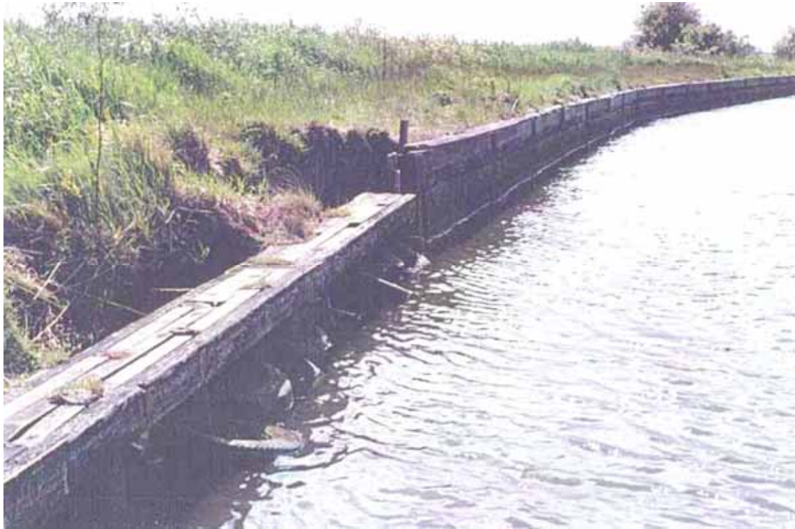
Figure 5.12 Tyre and post bank protection (courtesy Environment Agency)
