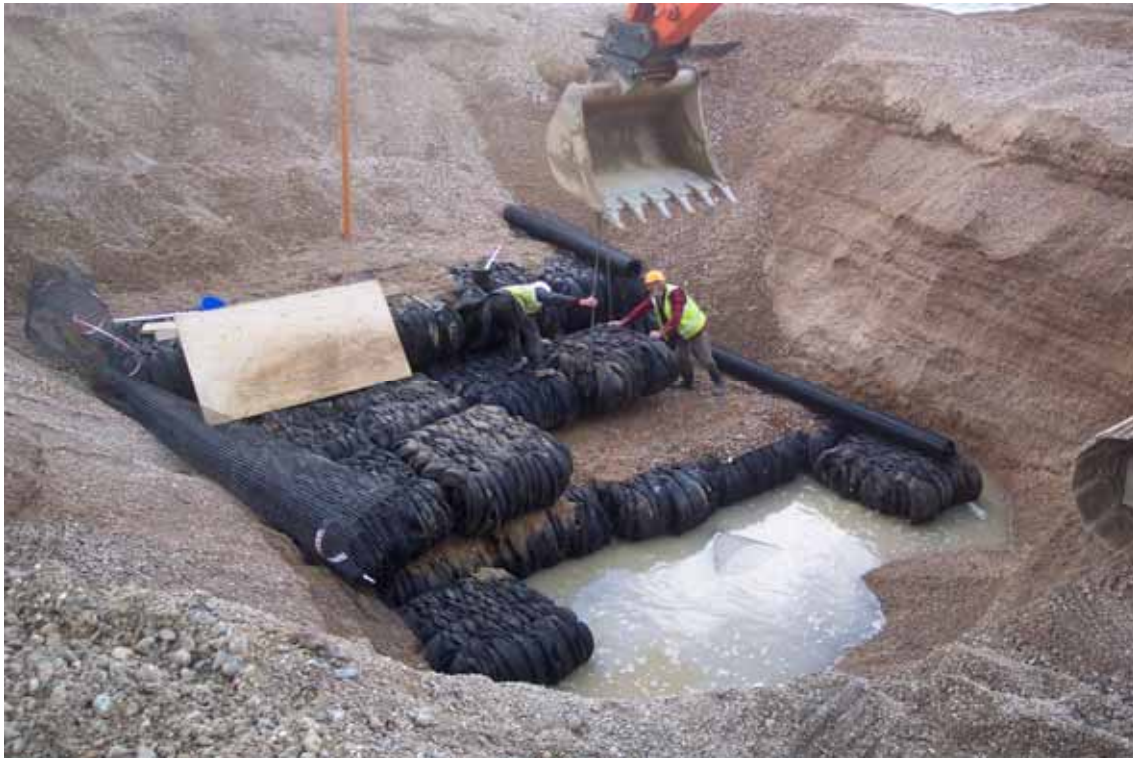
Figure 5.29 Installation of bales in the beach at Pevensey Bay in East Sussex (courtesy PCDL)
