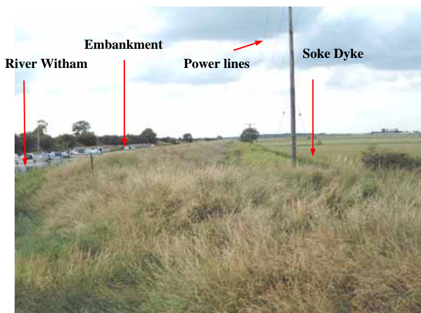
Figure A8.3 Relative positions of the river, embankment, powerlines and soke dyke (courtesy Environment Agency)
