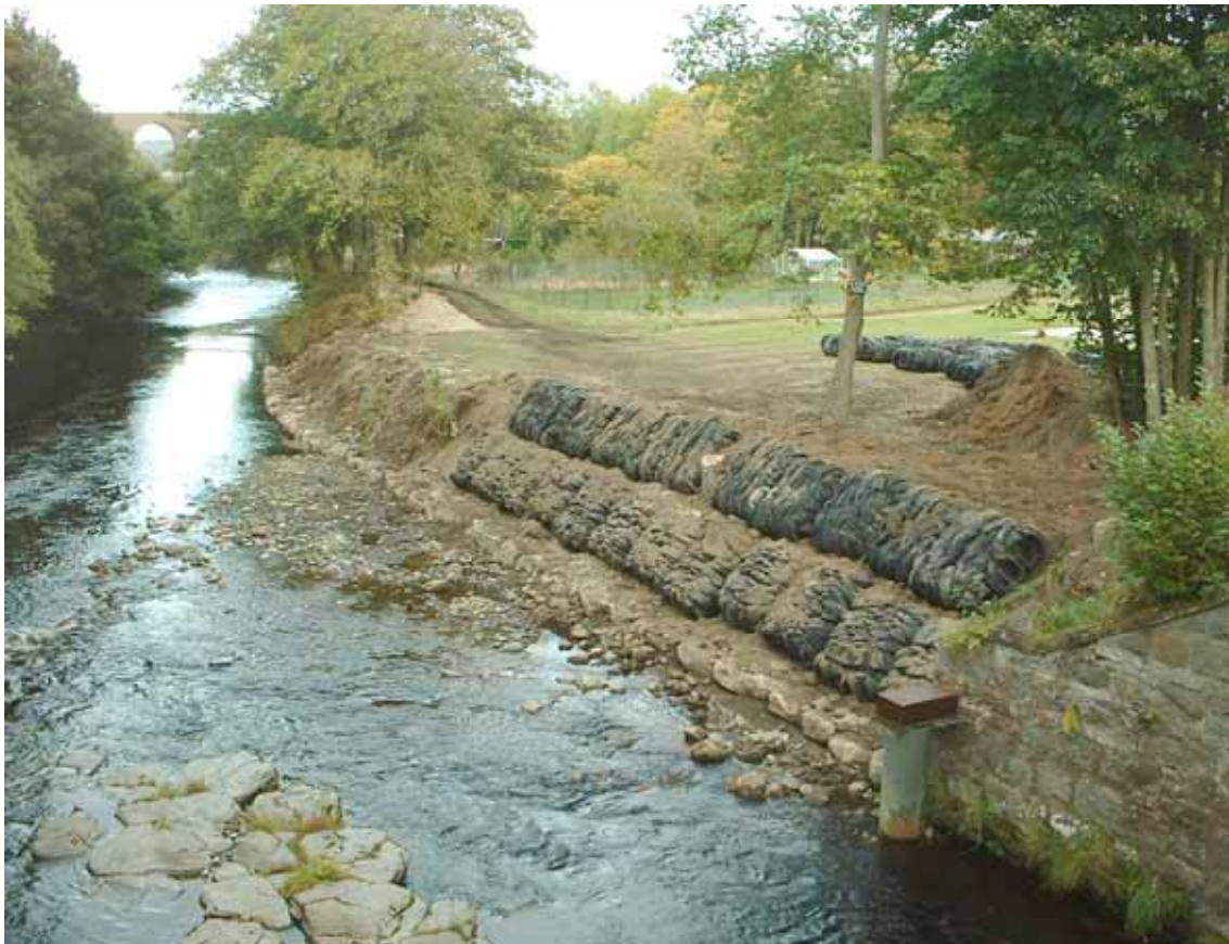
Figure 5.36 The Nairn River Bank, during construction (courtesy Northern Tyre Recycling)
