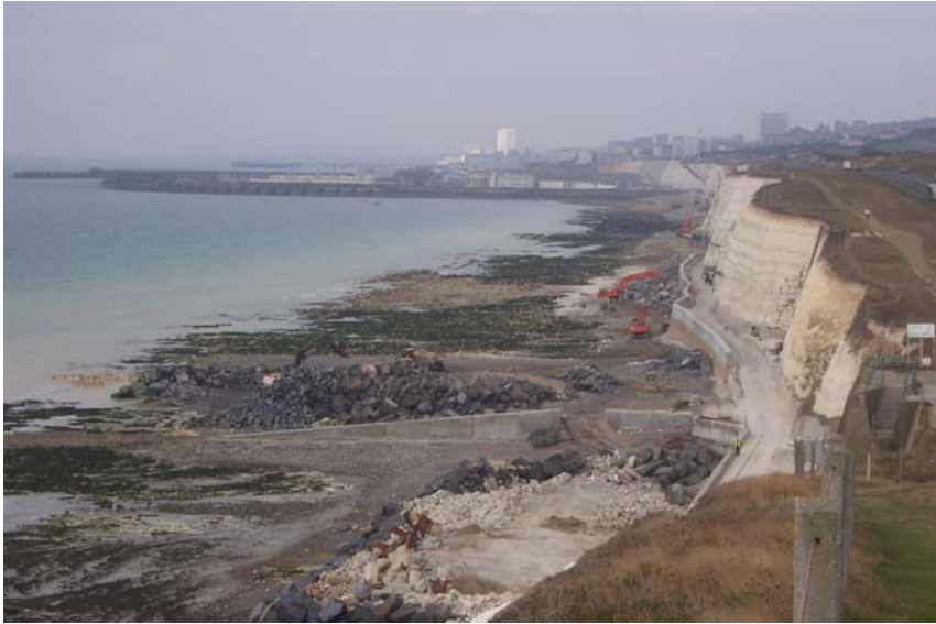
Plate 8.1 Brighton to Ovingdean coastal frontage during construction
