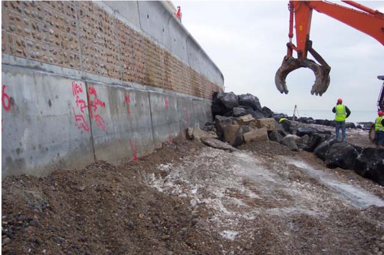
Plate 8.2 Use of demolished bullnose as secondary armour
