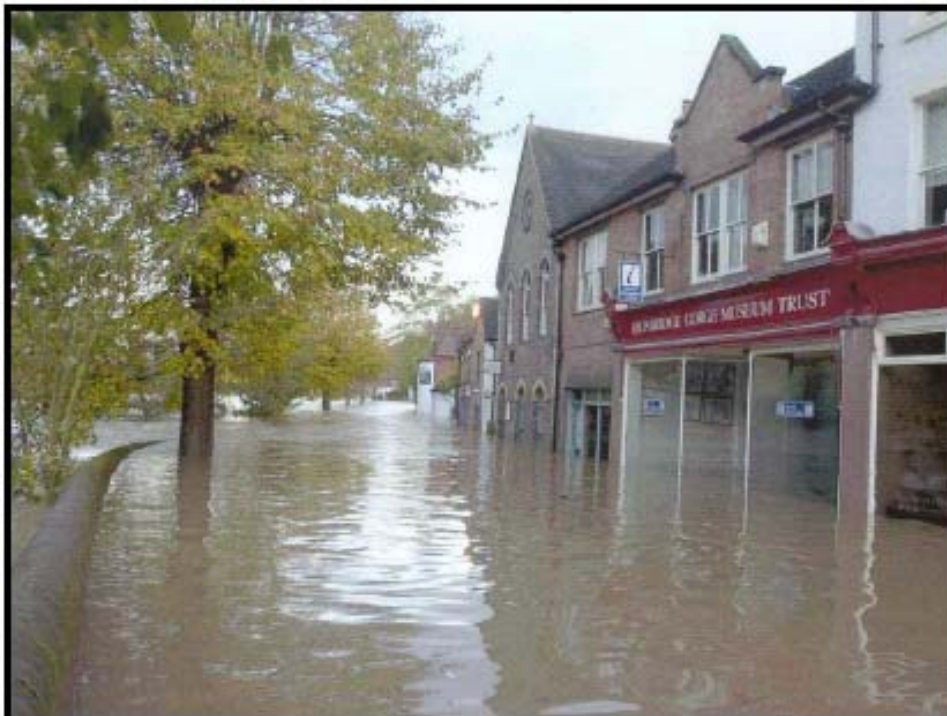
Flooding at the Wharfage in Ironbridge
