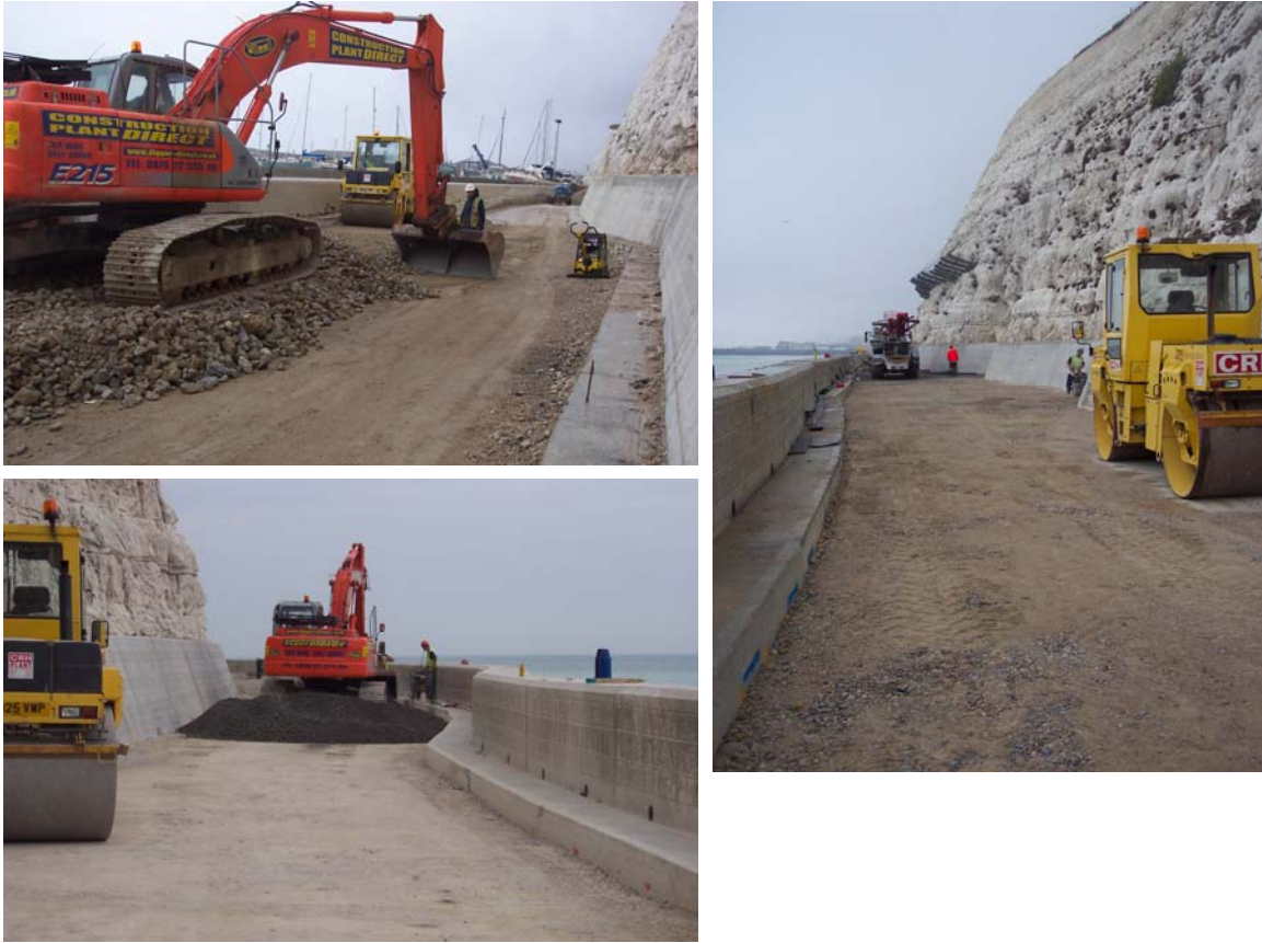
Plate 8.3 Use of demolition arisings as fill for promenade raising
