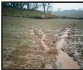
7. Erosion of unprotected natural drainageways
