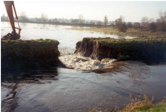
Figure 1 Overtopping and erosion of bank material led to this breach of a river embankment
