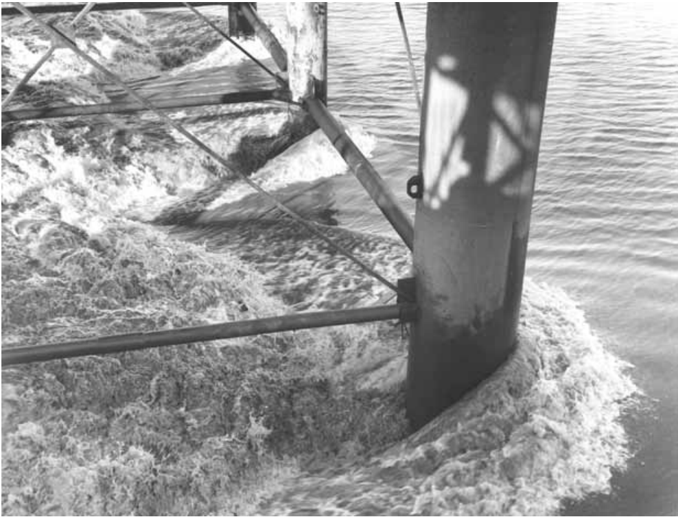
Plate 1 – Flow around bridge piers – River Severn
