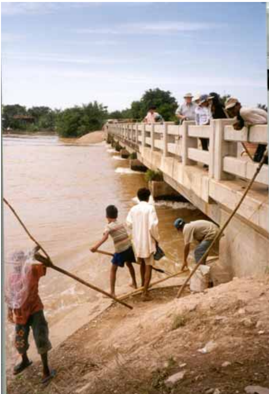
Plate 6 – Flood flow at bridge – Cambodia
